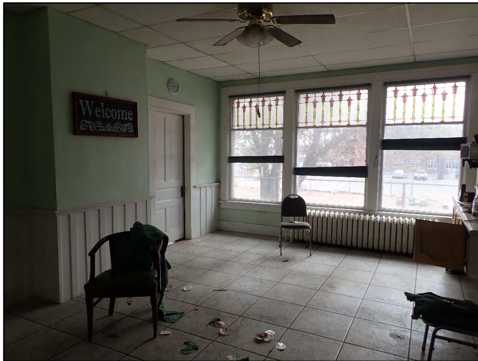
Figure D-136. Overview of the interior of the dining room.
