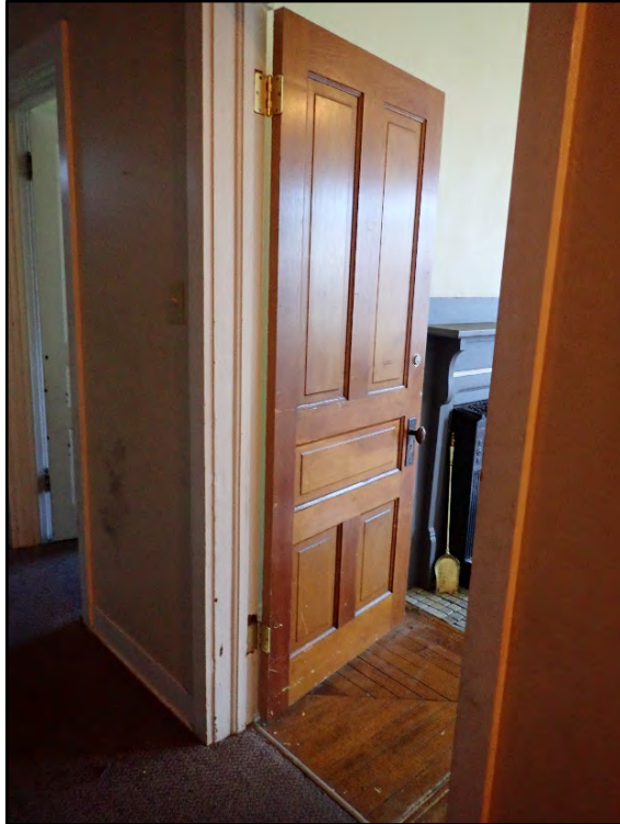
Figure D-233. The solid-core wood door to the master bedroom.
