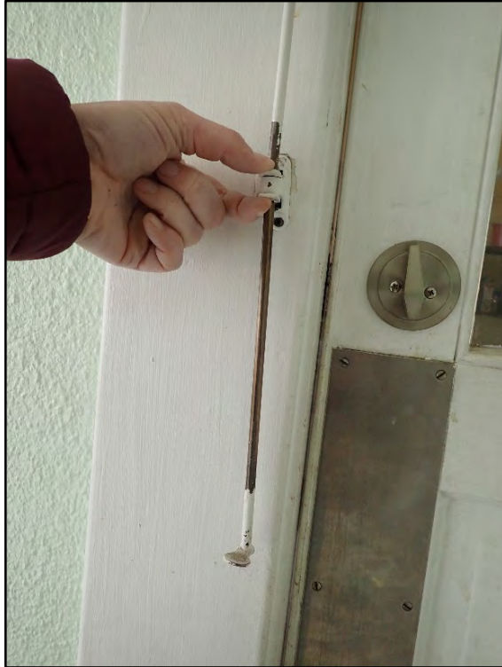
Figure D-141. The mechanism for the upper transom is still in working order.
