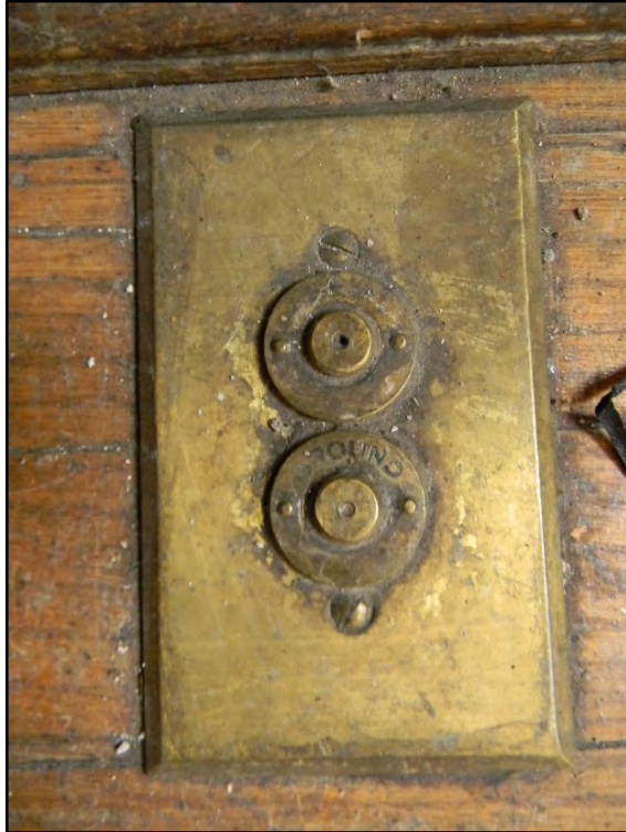
Figure D-121. Electrical outlet in the floor of the formal living room (likely also original).
