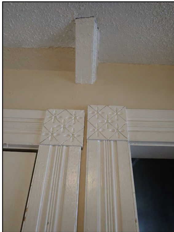
Figure D-220. Detail of the decorative architraves (side casings) and corner blocks of the under-stair closet and entrance hall as seen in the main hallway.
