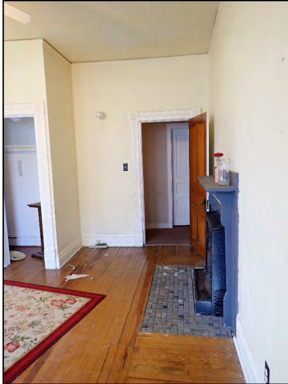
Figure D-237. A view of the profile of the fireplace and door to the hallway.
