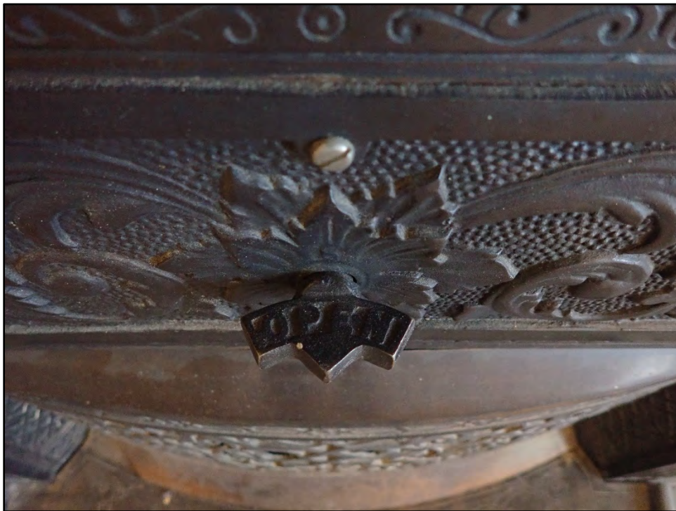
Figure D-248. A view showing the details on the knob that opens and closes the fireplace damper in the master bedroom.
