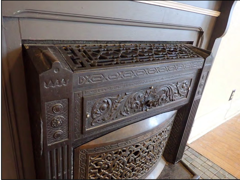
Figure D-247. The similarities between the master bedroom fireplace and that in the living room can be seen here.
