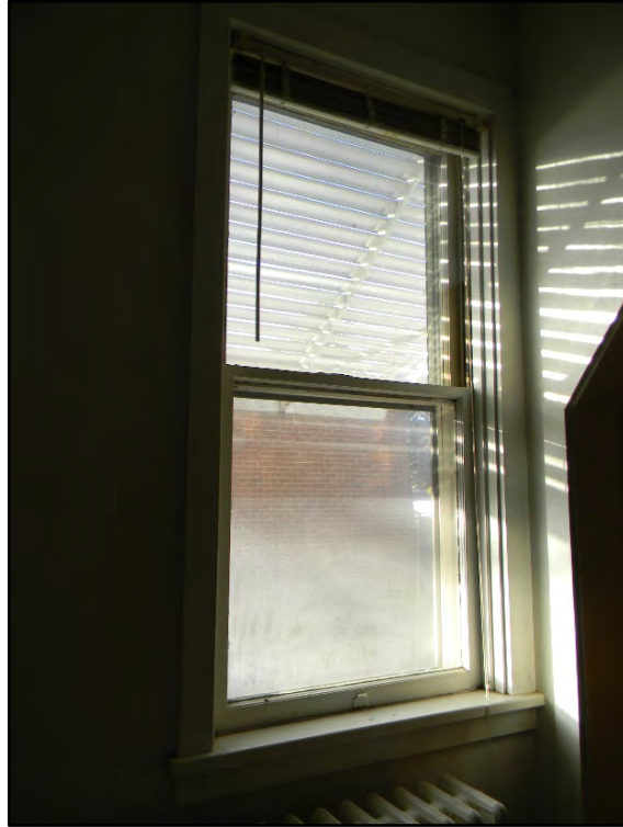
Figure D-169. Detail of one of the chapel windows.
