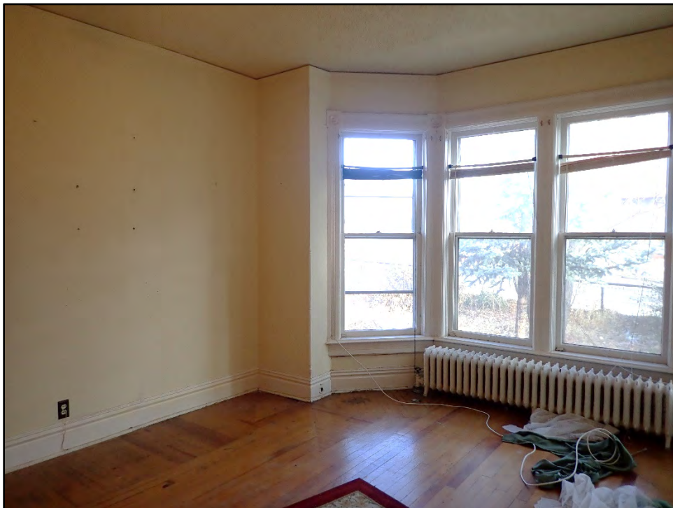
Figure D-236. View of the cant bay window in the master bedroom with original hardwood floors.
