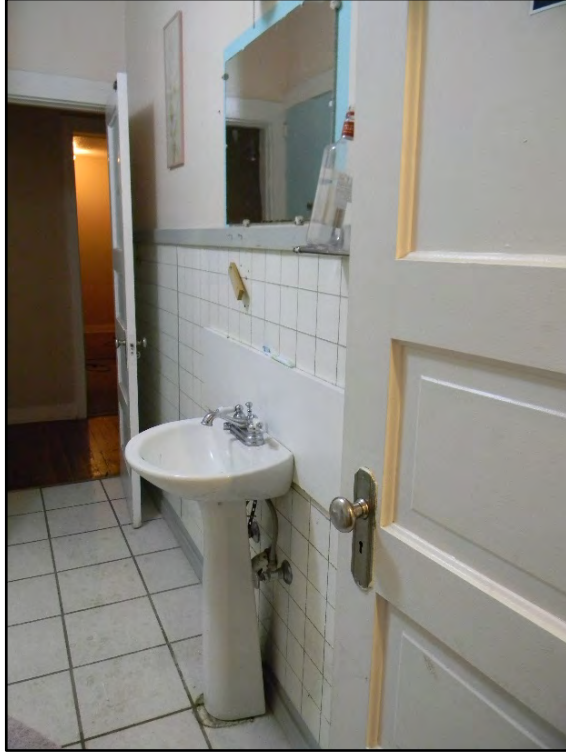
Figure D-197. A view through the connected bath as seen from the hallway near the small bedroom.
