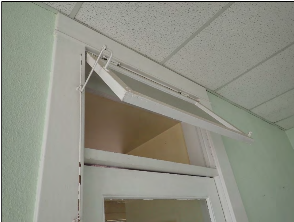
Figure D-140. Detail of the upper transom above the swinging door to the kitchen.
