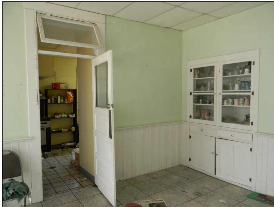
Figure D-138. View of the built-in cabinet and the swinging door to the kitchen.
