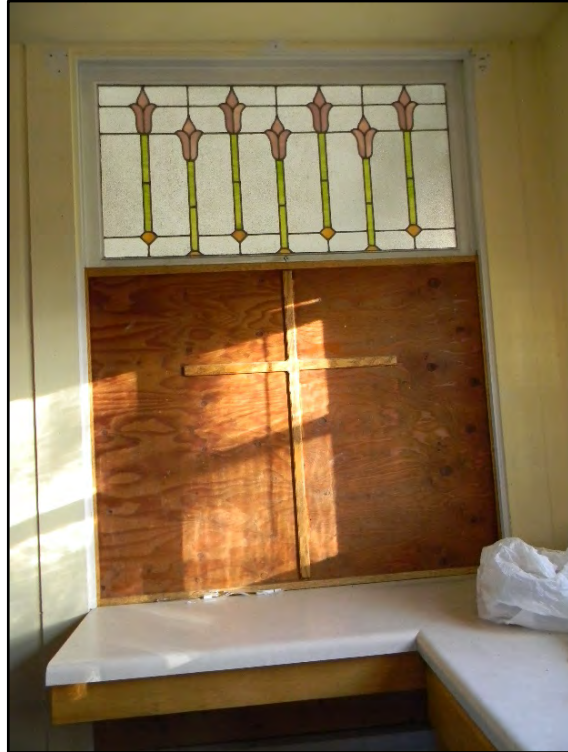
Figure D-155. View of the cottage window of the dining room.
