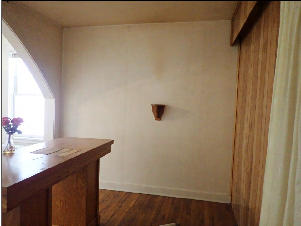
Figure D-173. View of the west wall of the chapel extension.
