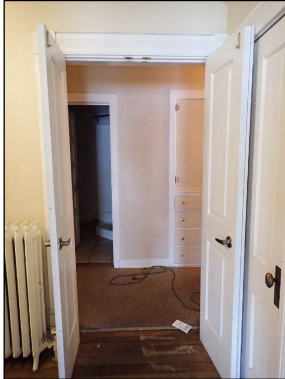
Figure D-229. The modern French doors opened to the hallway to the bedrooms (the under-stair closet is on the right).
