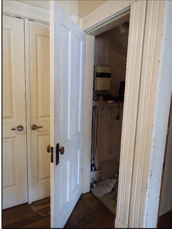
Figure D-223. The door to the under-stair closet next to the modern French doors in the main hallway.
