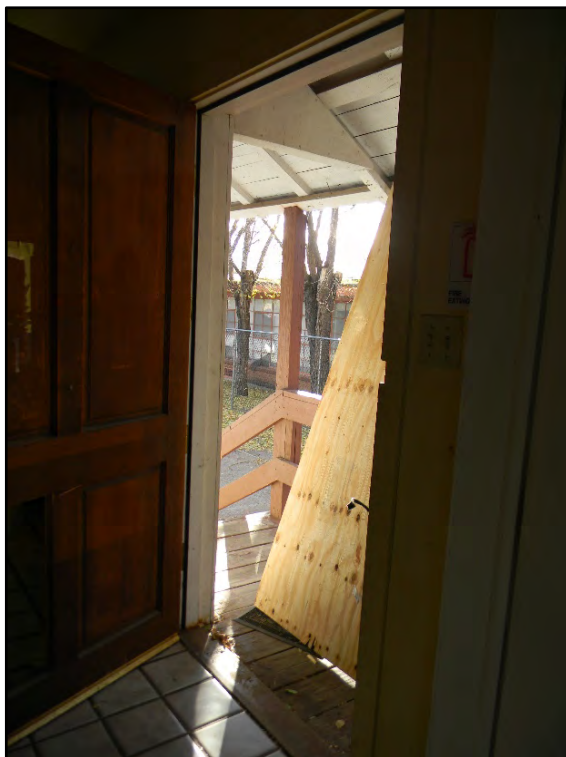
Figure D-160. The exterior door that is currently boarded up, and the only way to access the interior of the residence.
