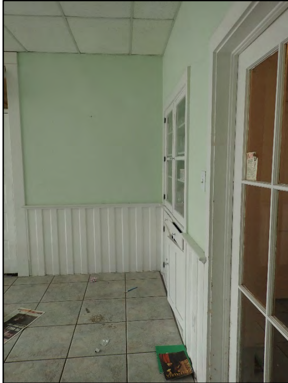
Figure D-133. View showing the wainscoting around the dining room.
