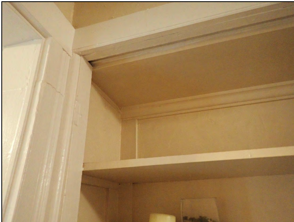
Figure D-212. Detail of the craftsmanship of the built-in cabinet shelving.
