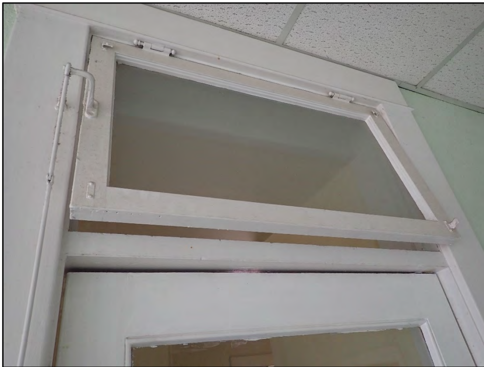
Figure D-142. View of the upper transom, which still opens and closes.
