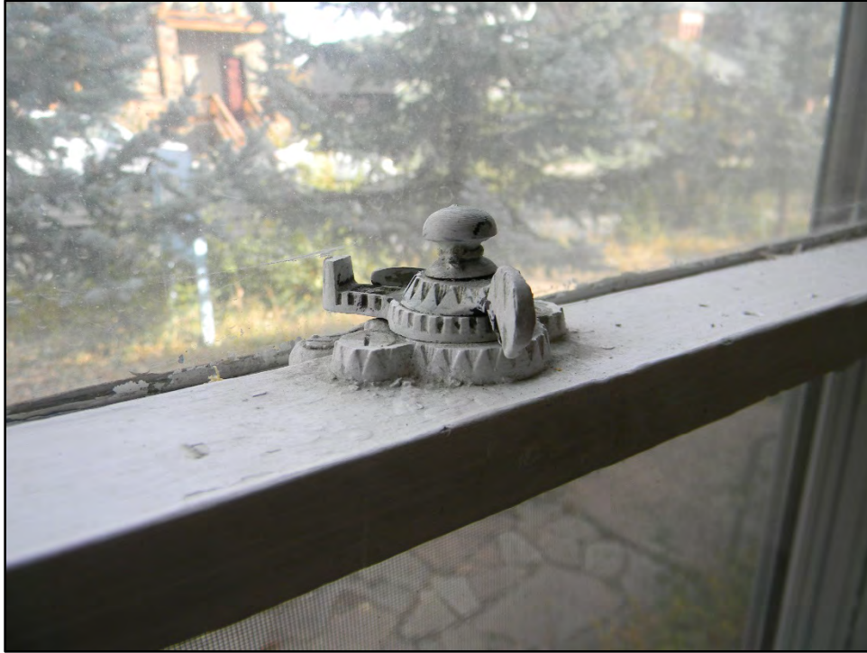
Figure D-241. Close-up view of the elegant details in the brass window lock of the cant bay window in the master bedroom.
