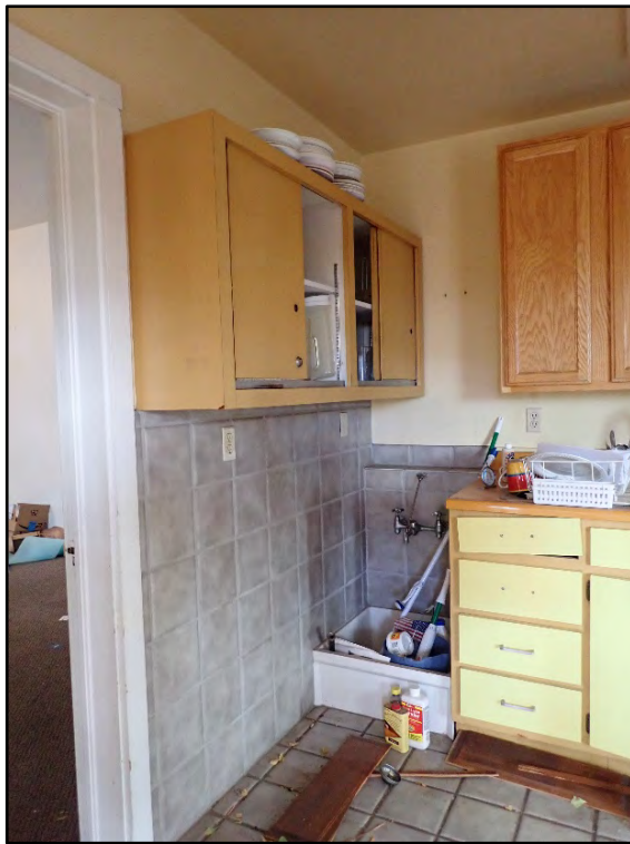
Figure D-164. View of the corner of the kitchen just outside the chapel.
