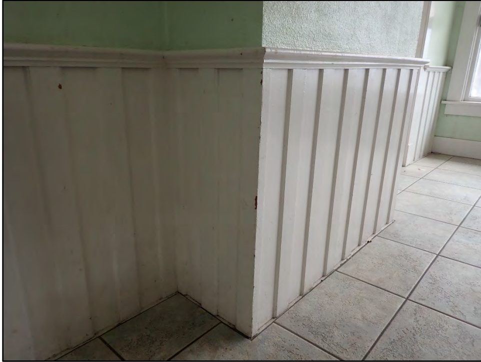
Figure D-131. Alternative view of the back of the built-in cabinet in the formal dining room, showing the wood wainscoting that rings the dining room.
