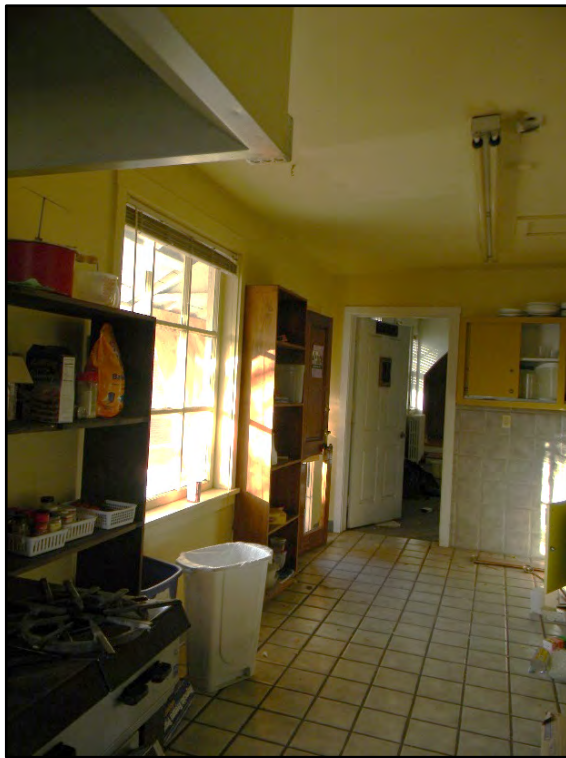
Figure D-152. Interior of the kitchen toward the exterior door.
