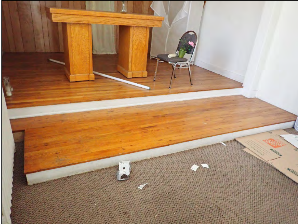
Figure D-171. Detail of the wooden steps of the chapel.
