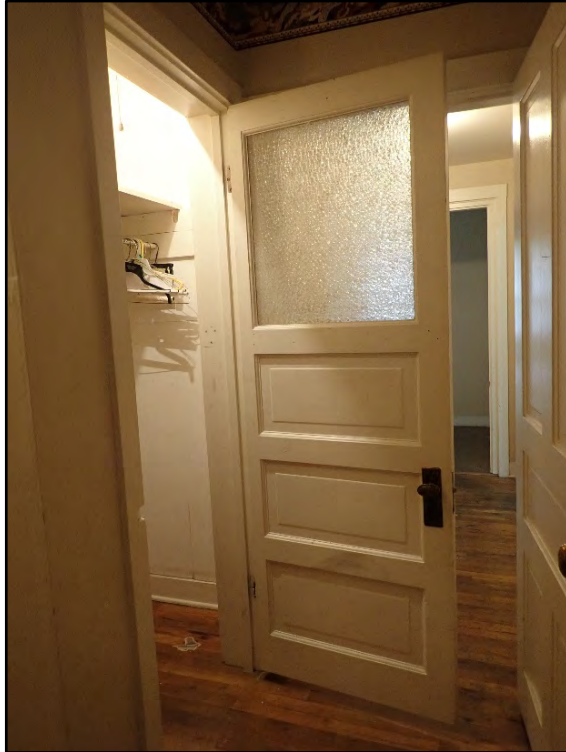
Figure D-193. View of the wood panel door with an upper panel of privacy glass.
