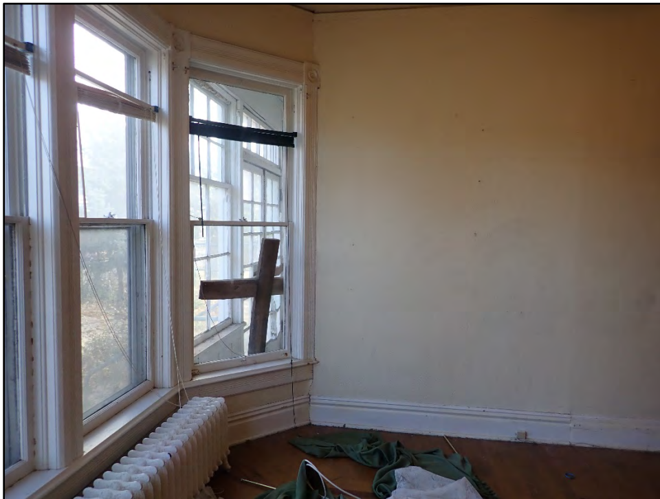
Figure D-238. A view toward the enclosed porch adjacent to the master bedroom, with the outline of the former entrance door visible in the right of the image (note the change in the baseboard at the lower right).
