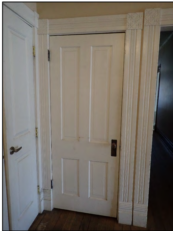
Figure D-222. Original door to the under-stair closet in the main hallway of the first floor.
