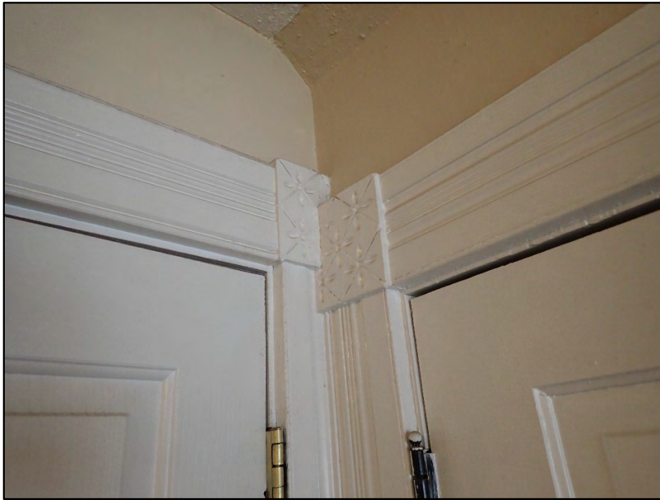
Figure D-228. Detail of the decorative corner blocks and side casings around the door to the under-stair closet and French doors to the other hallway to the bedrooms.
