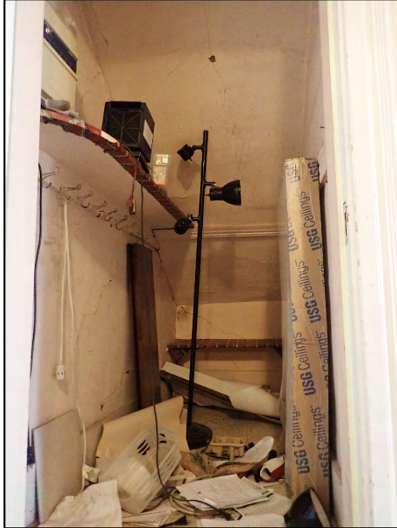
Figure D-225. An additional view of the under-stair closet.
