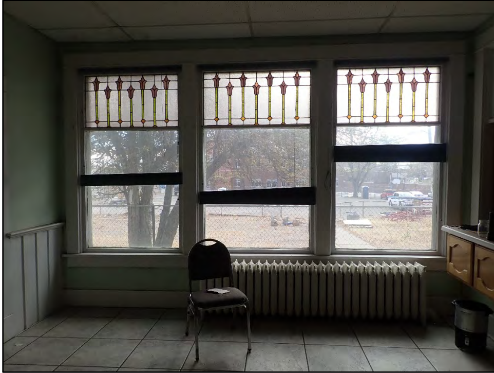
Figure D-145. Overview of the cottage windows in the dining room.
