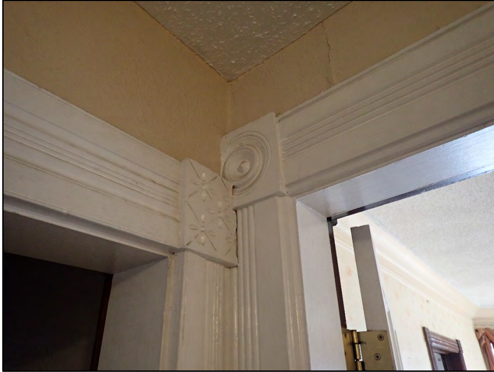
Figure D-221. Detail of the architraves (side casings) of the entrance hall and formal living room as seen in the main hallway.
