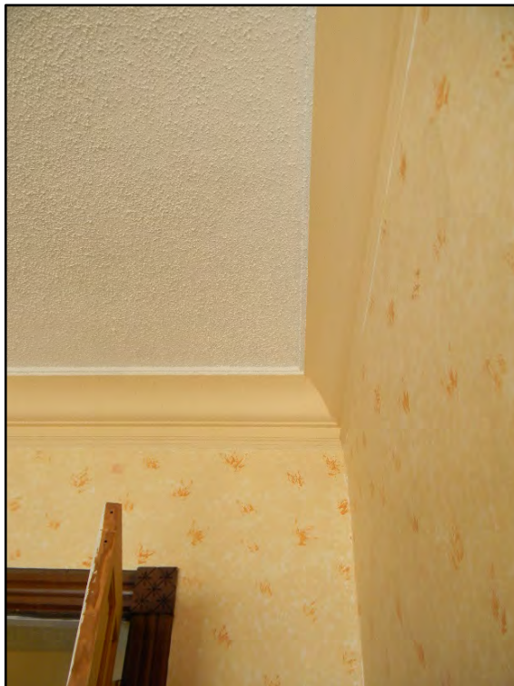
Figure D-118. Detail of the crown molding and curved ceiling of the formal living room.
