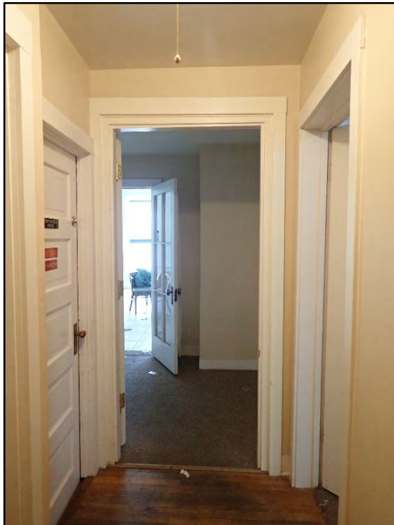
Figure D-198. From outside the connected bath, one can see the door to the chapel (right), to the basement (left) and through to the main hallway.
