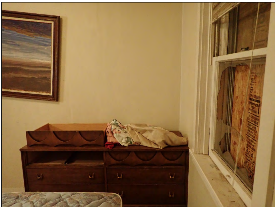
Figure D-188. Alternative view of the small bedroom and window.
