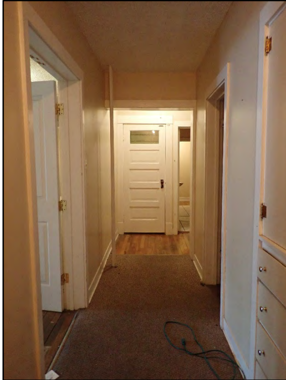
Figure D-279. View down the hallway toward the secondary staircase to the second floor.
