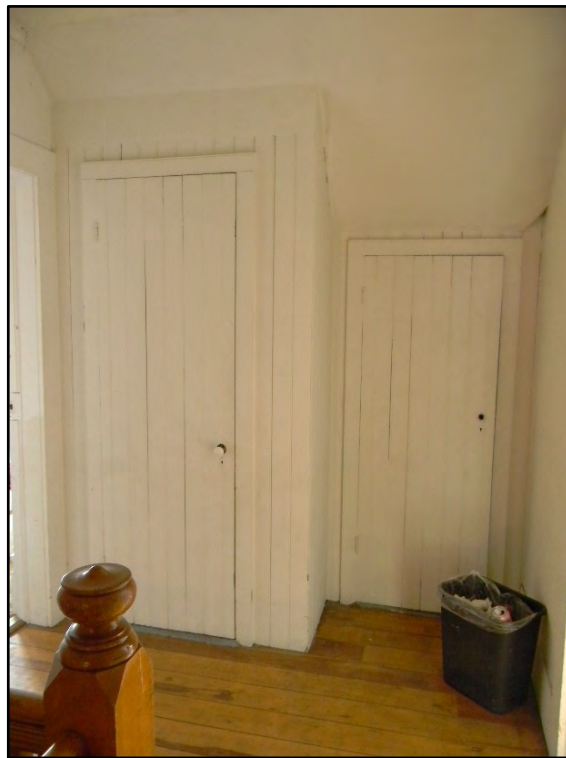
Figure D-358. Between the first and second bedrooms are two small storage closets created from batten panels and doors.
