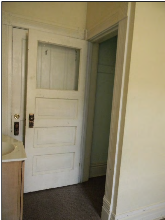
Figure D-262. The solid-core wood door with upper glass panel.
