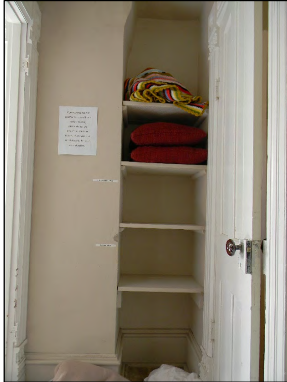
Figure D-385. Shelving has been placed between the outline of the chimney (from the master bedroom below) and the closet wall.
