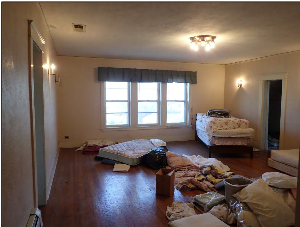
Figure D-392. An overview of the interior of the third bedroom, which was reconfigured to eliminate the steeply pitched roof and incorporate a grouping of three windows and full-height ceiling.
