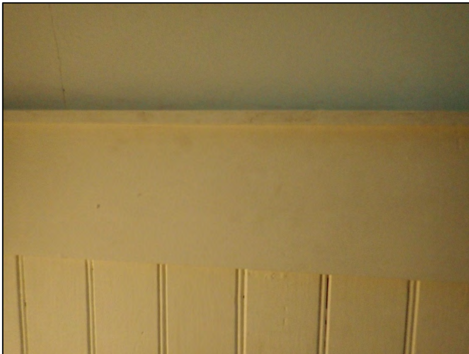
Figure D-332. A close-up view of the batten wood paneling and cap molding in the secondary staircase.
