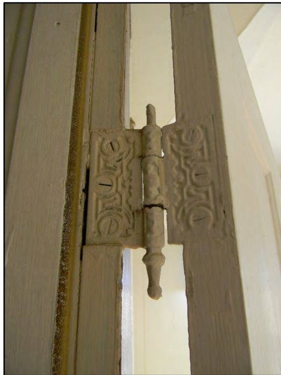
Figure D-354. A close-up view of the decorative bedroom door hinges which are still present.
