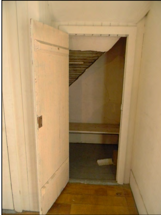
Figure D-359. The smaller closet door reveals the angled space obscured by these storage closets.
