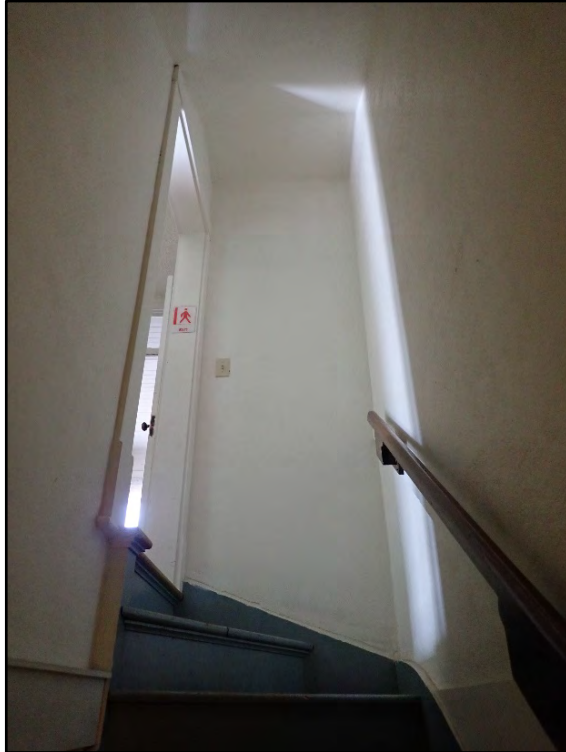
Figure D-327. Walking up the stairs toward the second floor.
