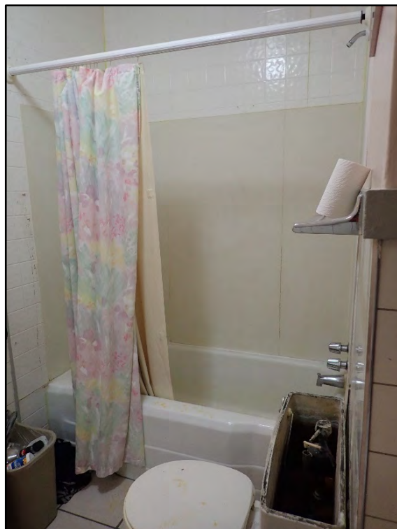
Figure D-298. Detail of the modern tub/shower combination.
