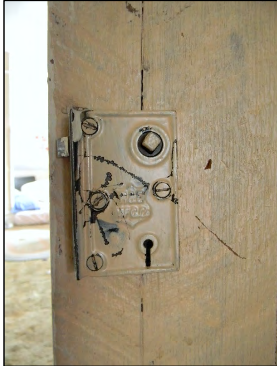
Figure D-363. A close-up view of the lock mechanism of the larger batten door.
