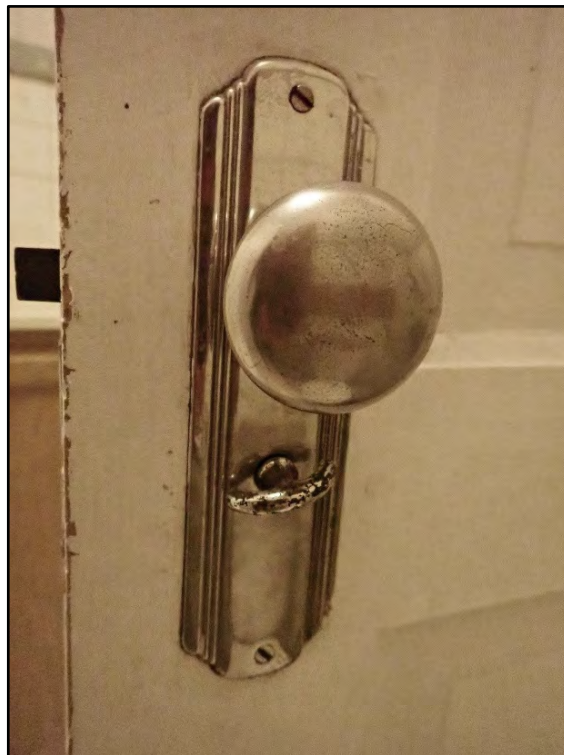
Figure D-288. Close-up view of the decorative door hardware of the hall bath.
