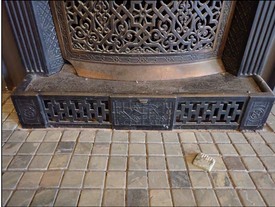
Figure D-249. Detail of the tiles of the hearth extension of the fireplace.
