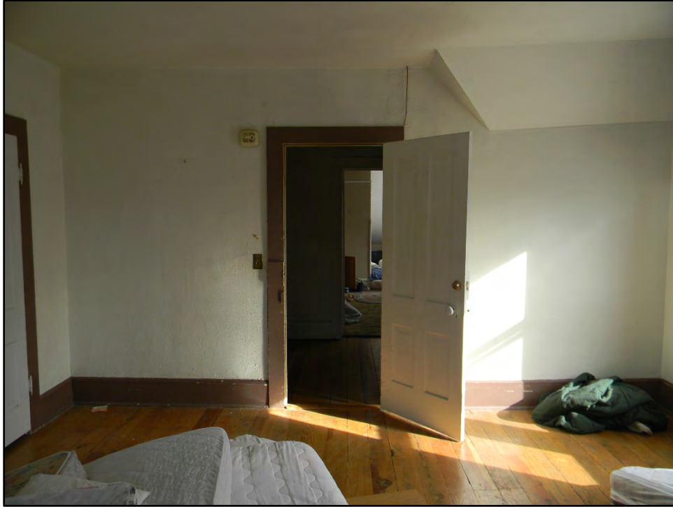
Figure D-349. A look back toward the main hallway on the second floor.
