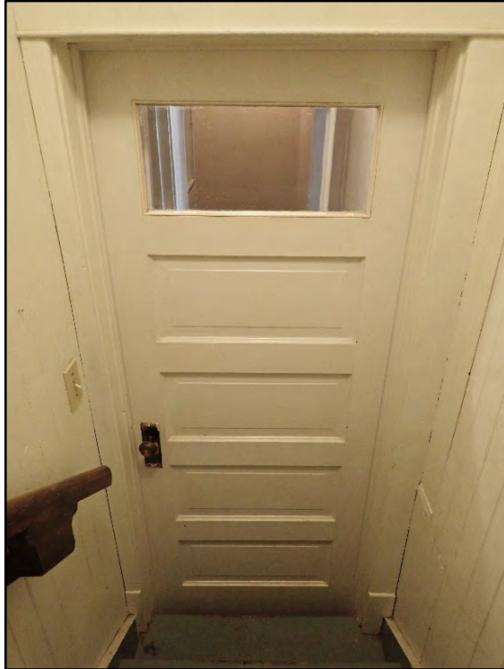
Figure D-329. The interior of the door at the bottom of the secondary stair.
