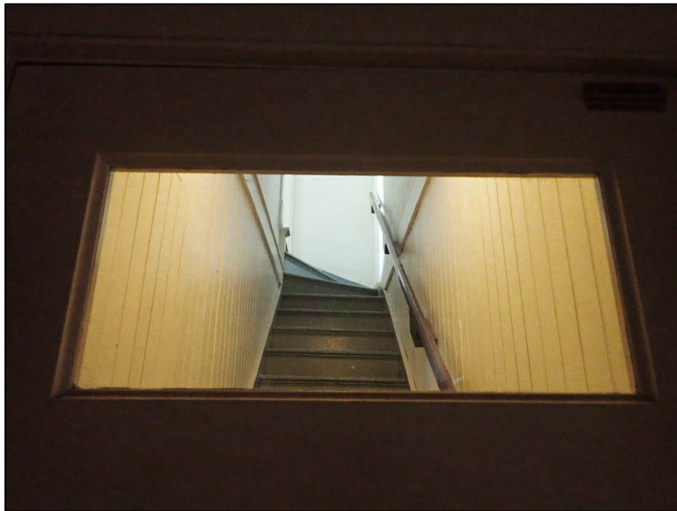
Figure D-324. The secondary staircase on the west end of the home as seen through the upper glass panel of the door.
