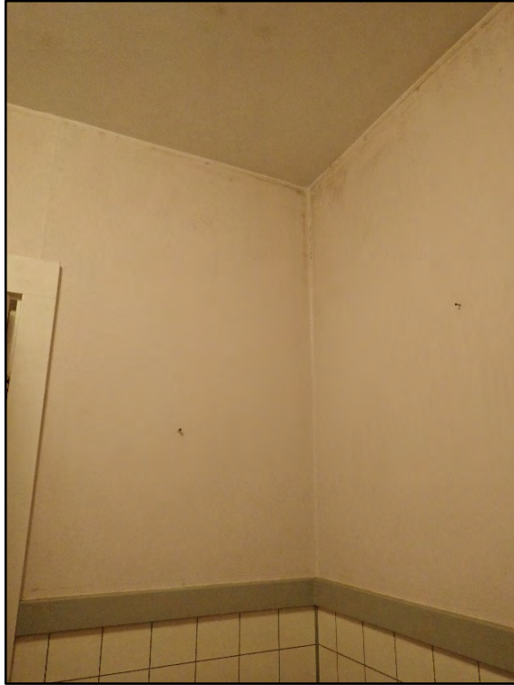
Figure D-285. Detail of the finish of the walls above the tile wainscot and cap molding in the hall bath.
