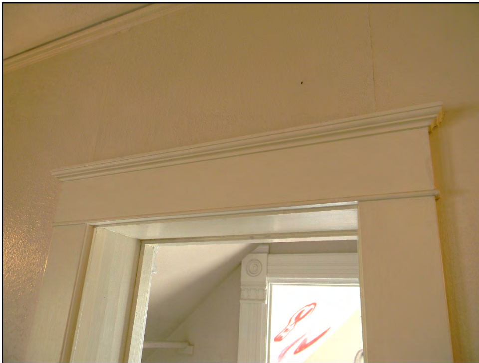
Figure D-390. Compared to the trim in the second bedroom, the door trim of the third bedroom appears rather plain, but still reveals a high-level of craftsmanship through the cap molding and side door jambs.
