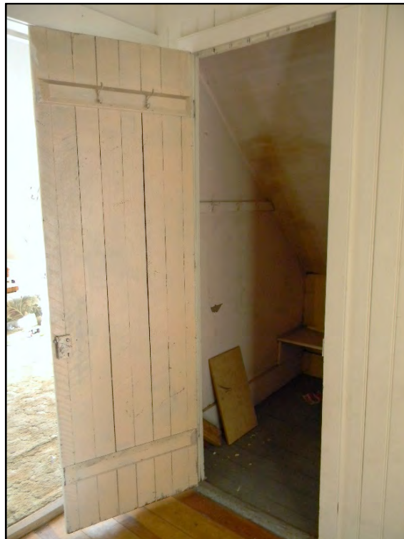
Figure D-362. The larger batten door of the storage closets.
