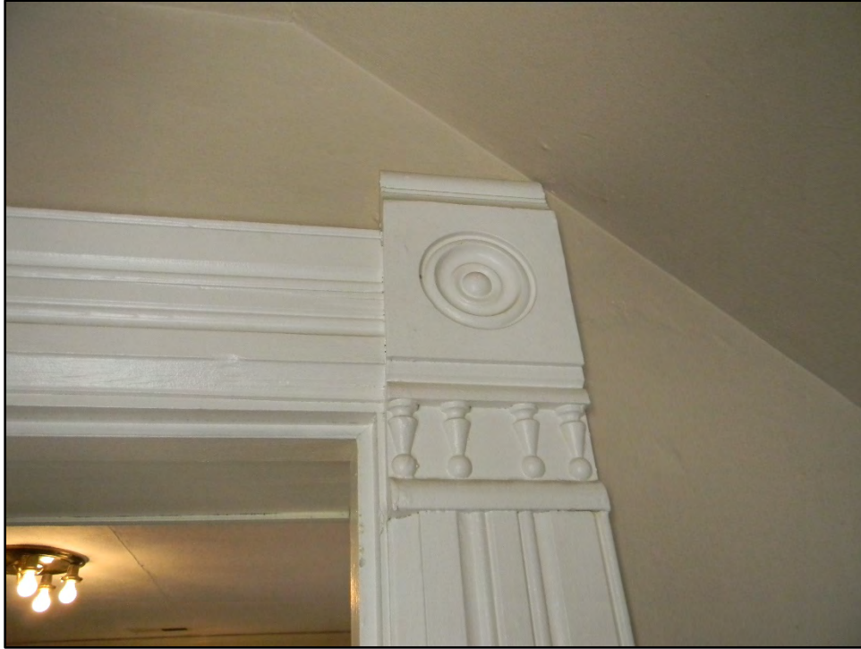
Figure D-383. A close-up view of the architrave and corner block of the connected closet.
