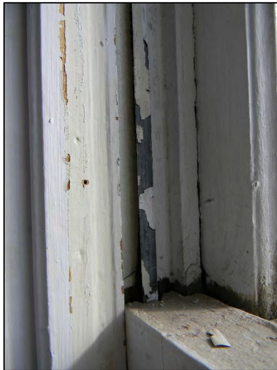
Figure D-378. An even closer look reveals the metal strip mechanism that opens the single-hung window, which is still in working order after 130 years.
