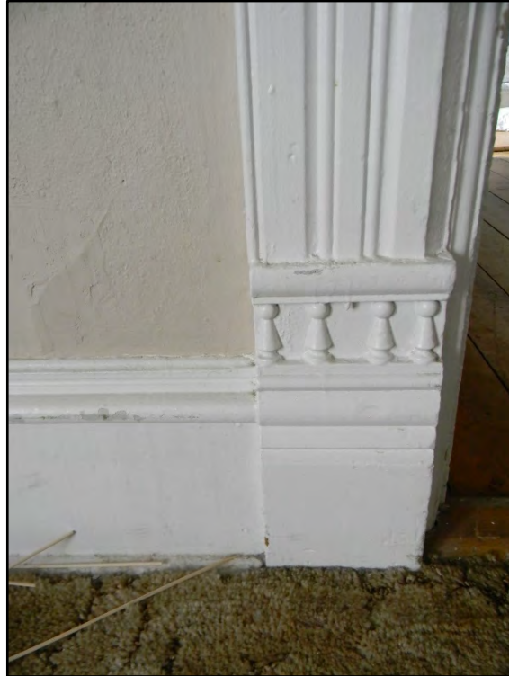
Figure D-371. A close-up view of the decorative wood baseboard and plinth block of the second bedroom.
