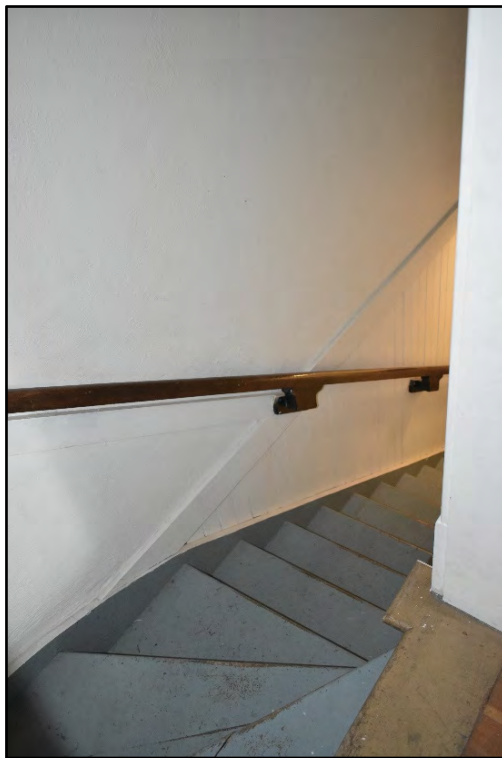
Figure D-336. Alternative view showing the construction of the secondary staircase.
