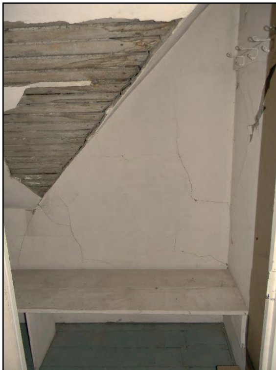
Figure D-360. A peek into the closet reveals a small bench and the lath-and-plaster wall construction that is original to the 1886 residence.
