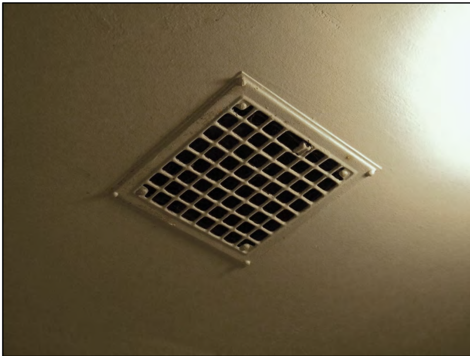
Figure D-286. Detail of the historic-era vent in the ceiling that may indicate this space was used as a bathroom when first constructed (and may be part of the expansion between 1895 and 1901).
