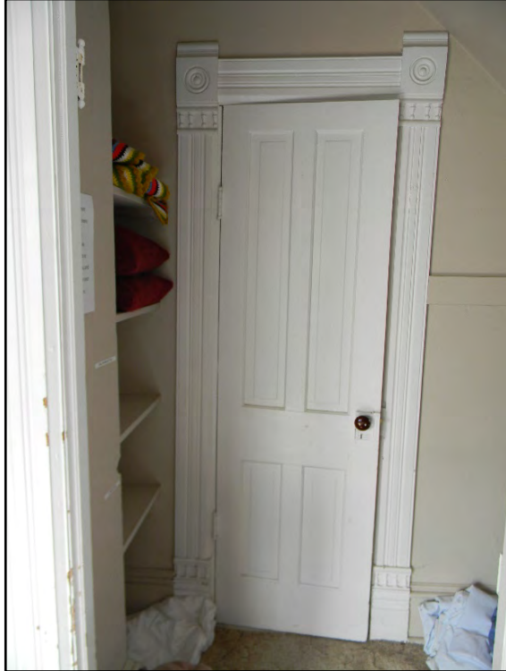
Figure D-387. The small, narrow door of the west side of the connected closet.
