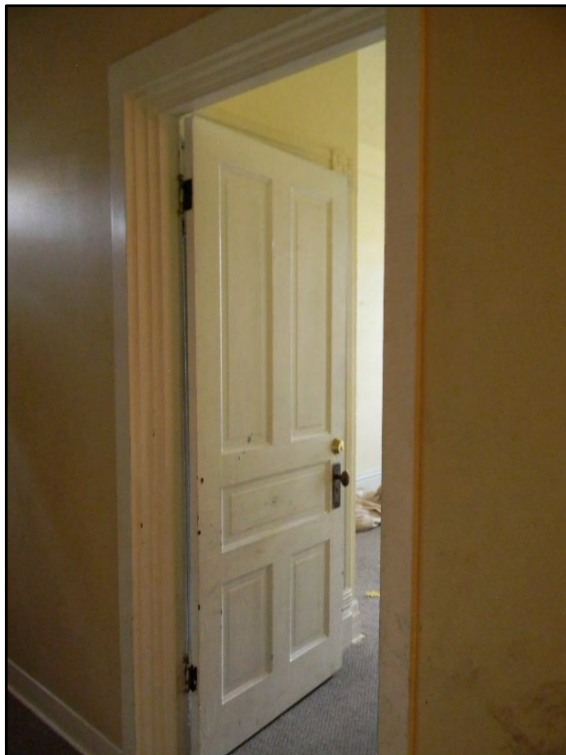
Figure D-254. The solid-core door of the first small bedroom.
