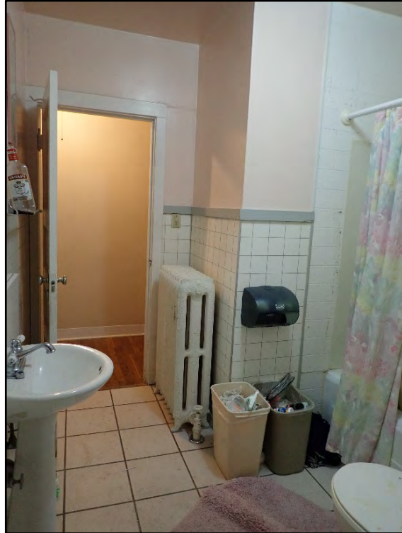
Figure D-297. An interior view of the west side of the connected bath.
