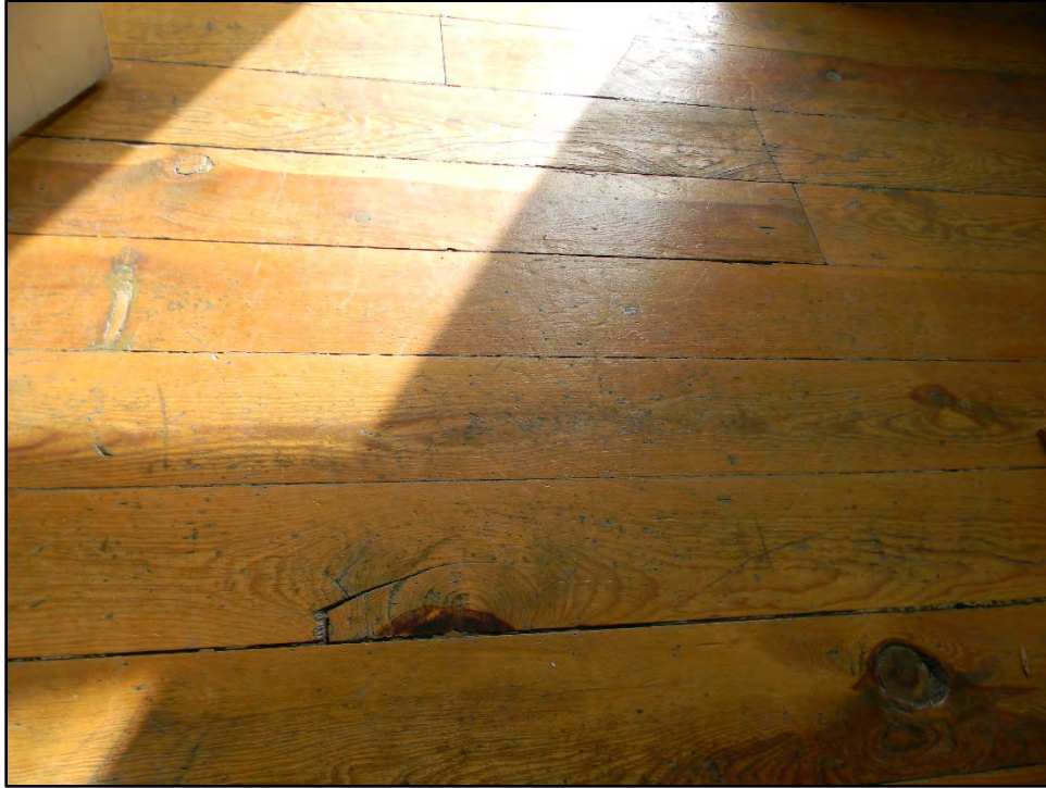
Figure D-353. Detail of the hardwood floors in the first bedroom.
