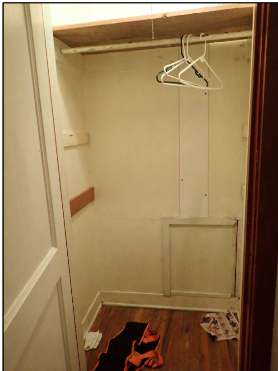
Figure D-316. Detail view of the interior of the closet.
