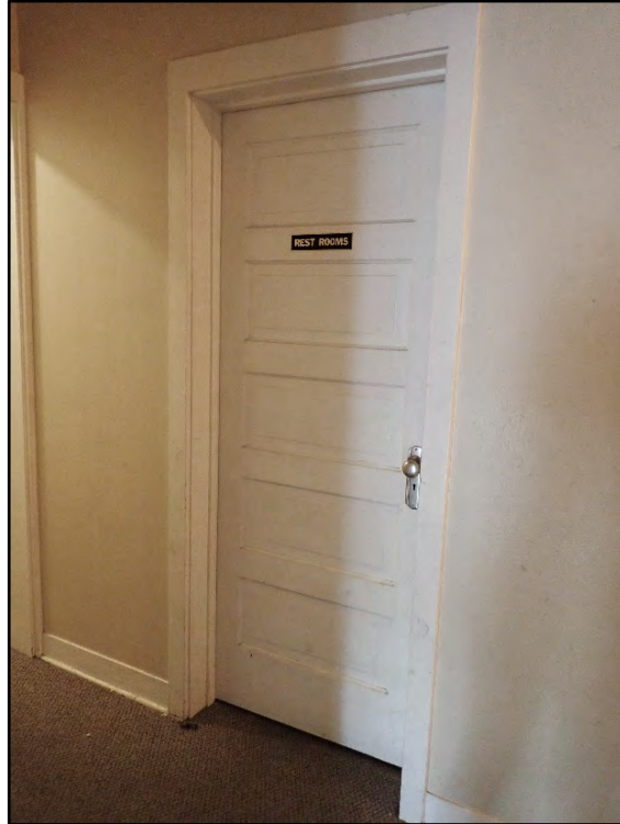
Figure D-291. The wood panel door to the small hall bath.
