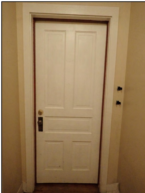
Figure D-320. The original solid-core wood door to the third small bedroom.
