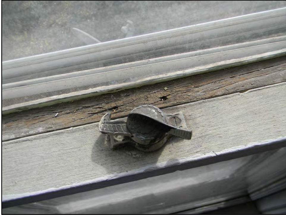
Figure D-377. A close-up view of the carved brass window lock.
