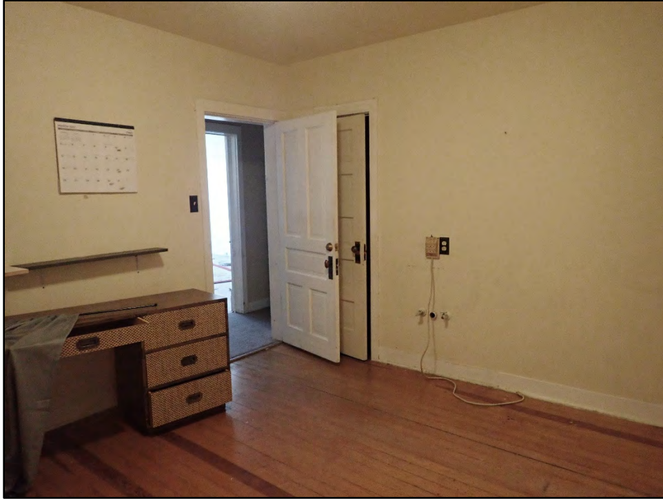
Figure D-271. View of the interior of the second bedroom toward the door and hallway.
