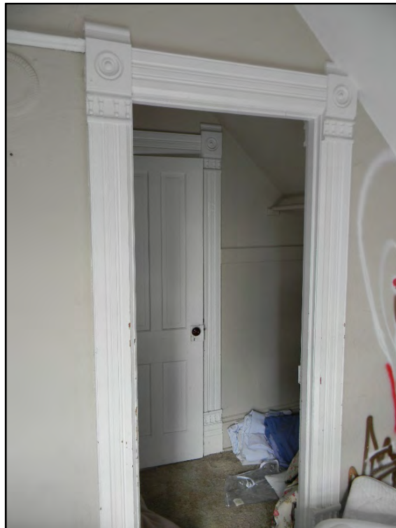
Figure D-382. A peek through the connected closet reveals the same wood trim around the original solid-core wood door.
