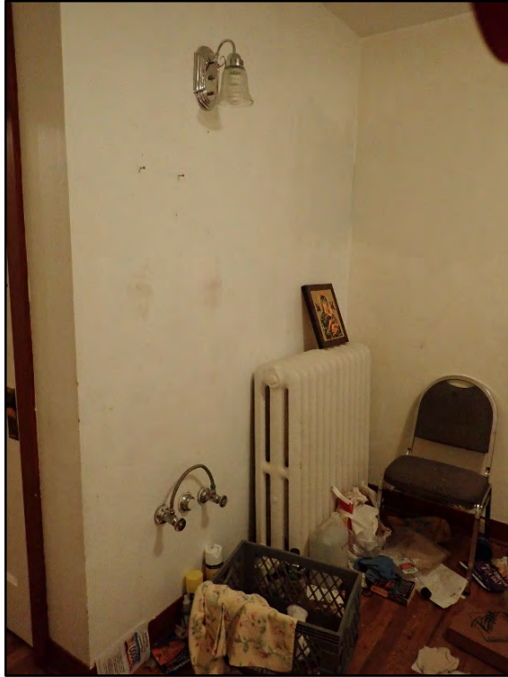
Figure D-313. The decorative radiator in the corner of the bedroom.
