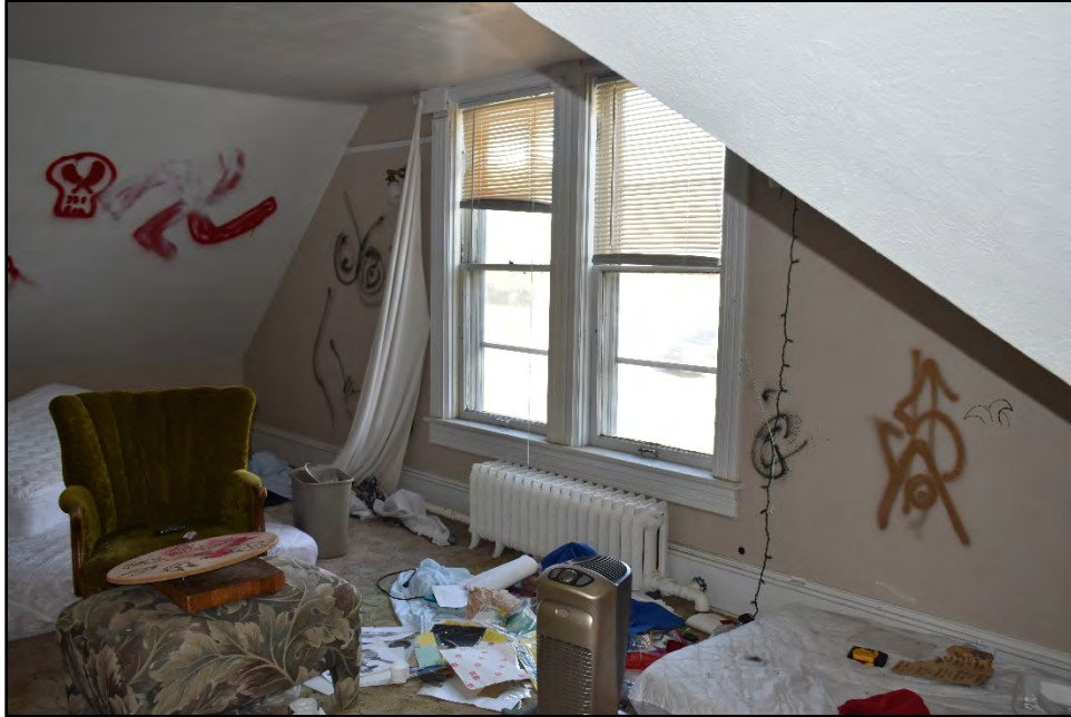
Figure D-367. The vandalism of the second bedroom attempts to distract from the original elements still present in this room (please excuse the inappropriateness of the graffiti in this image).
