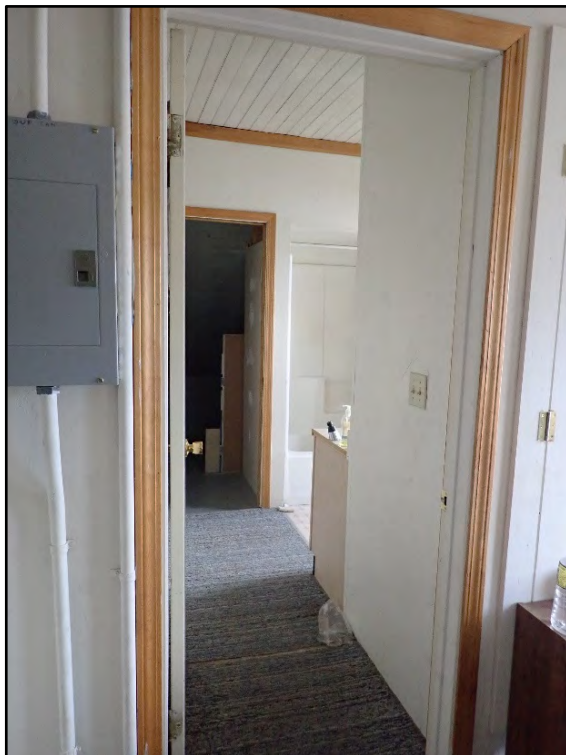
Figure D-488. Looking into the modern bath, which was constructed by dividing up the sleeping porch along the west side of the second floor.
