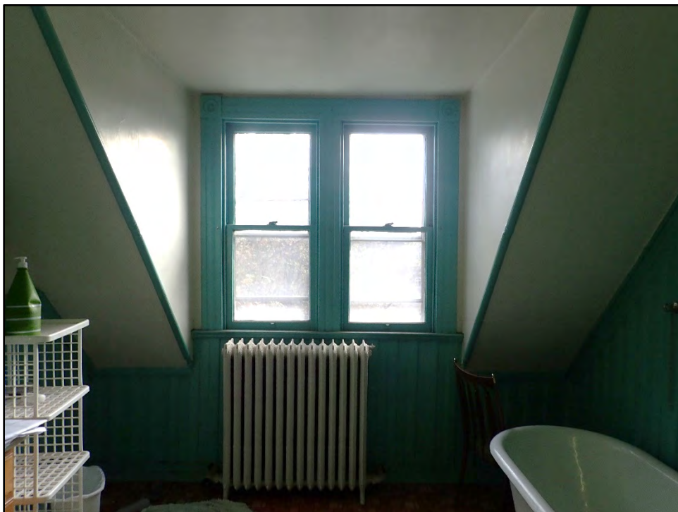
Figure D-536. View of the paired windows in the gable end framed by the shape of the ceilings and walls of the hipped-roof dormer.
