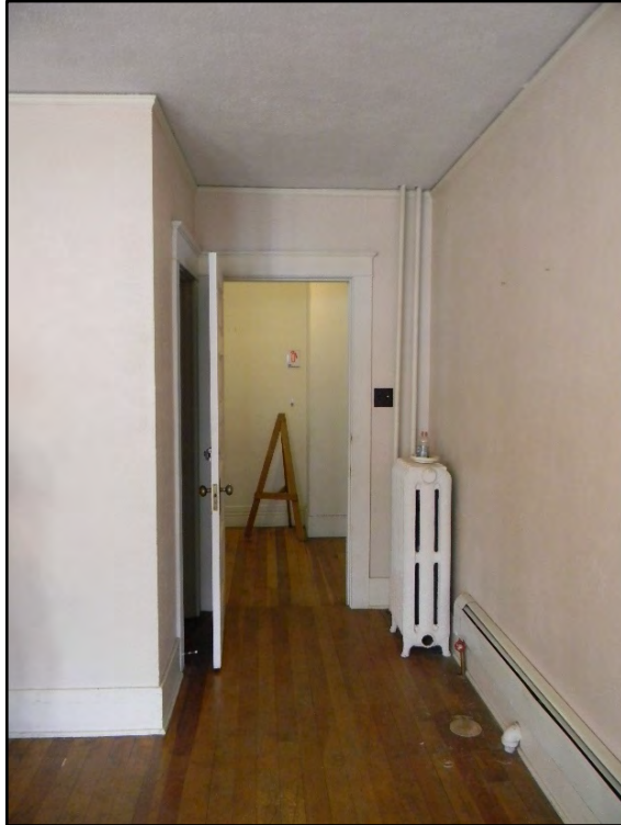
Figure D-395. The main hallway as seen through the bedroom door.
