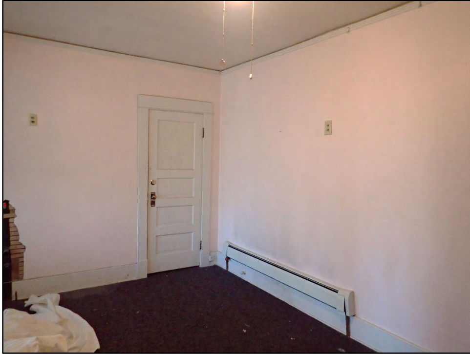
Figure D-425. Alternative view of the interior of the bedroom (this is the door to the interior hallway).
