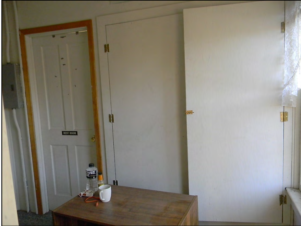
Figure D-483. View of the south wall of the sitting area, which consists of modern materials, with the door to the modern bath at left and storage area for the small furnace and water heater on the right.
