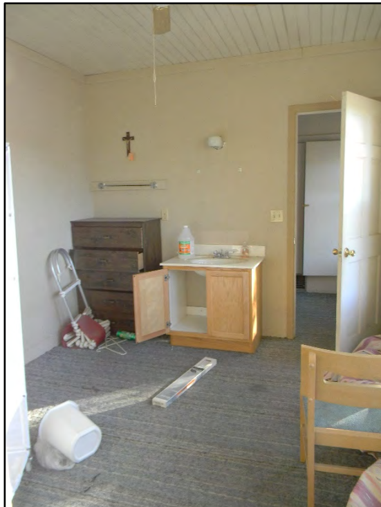
Figure D-478. An overview of the interior of the second small room, looking toward the south wall (the original window of the interior bedroom that are now covered up are under the sheetrock/drywall on the left).
