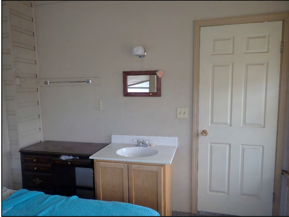
Figure D-473. View of the south wall of the first small room, showing the modern dividing wall, hollow-core door, and other upgraded amenities.
