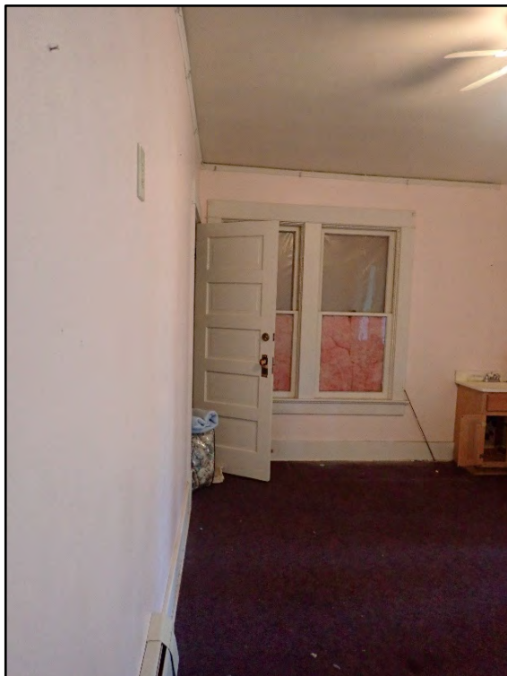
Figure D-418. Looking toward the corner closet and enclosed windows of the interior bedroom from the interior hallway.
