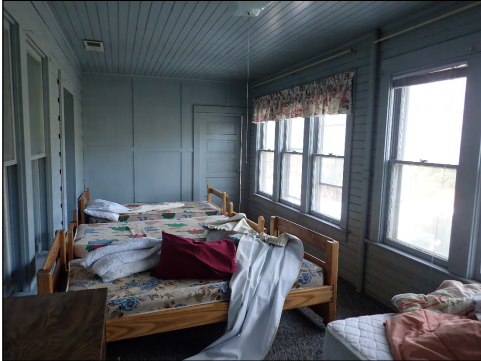
Figure D-459. Overview of the interior of the sleeping porch.
