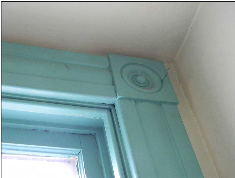
Figure D-534. Close-up view of the window casings and corner block in the large bath.
