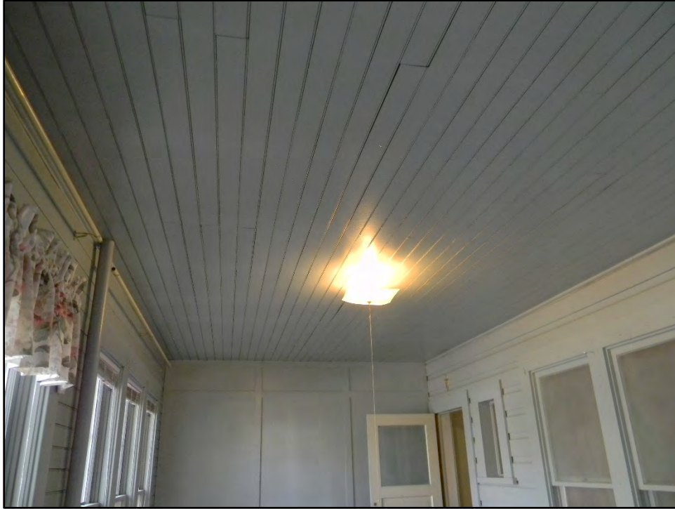
Figure D-467. Detail of the wood panel ceiling of the sleeping porch.
