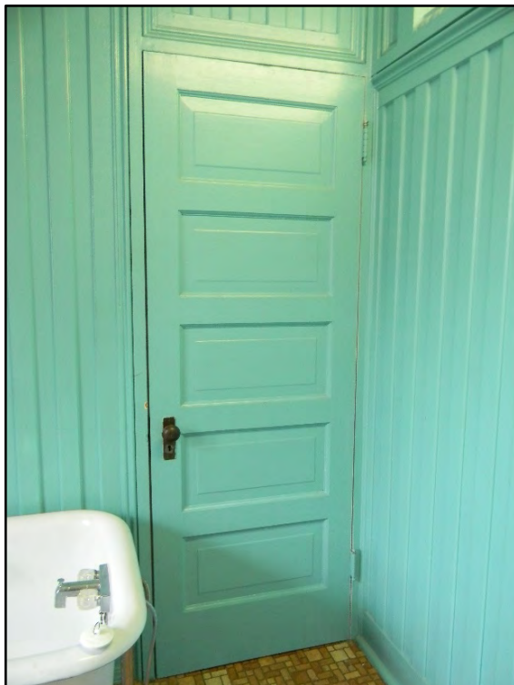
Figure D-522. View of the original door to what is now a separate shower.
