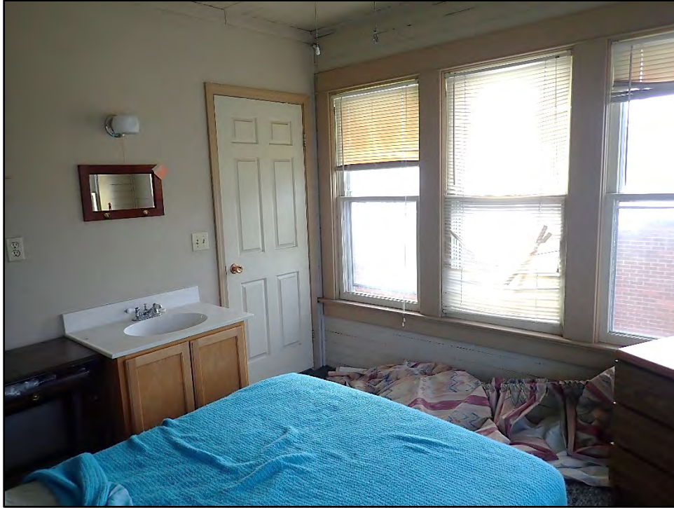
Figure D-471. Overview of the first small room, with the modern sheetrock/drywall on the left installed to divide up the sleeping porch on this side of the house.
