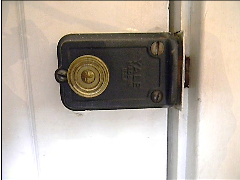
Figure D-399. A close-up view of a historic-era Yale deadbolt lock on the door to the third bedroom.
