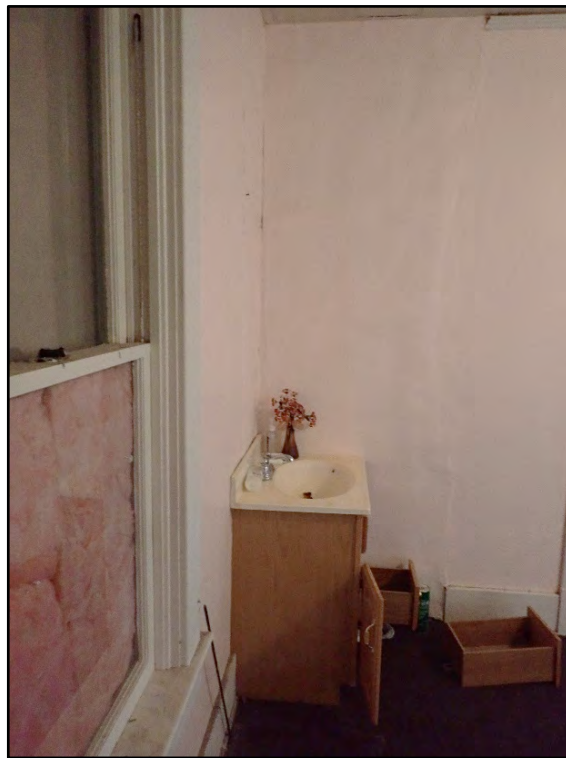
Figure D-434. A view of northwest corner of the interior bedroom.
