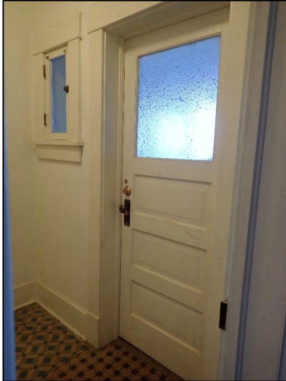
Figure D-443. The door to the sleeping porch also has an upper panel of privacy glass.
