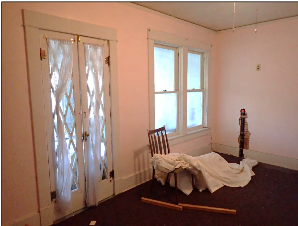
Figure D-426. Overview of the French doors and windows to the sleeping porch.
