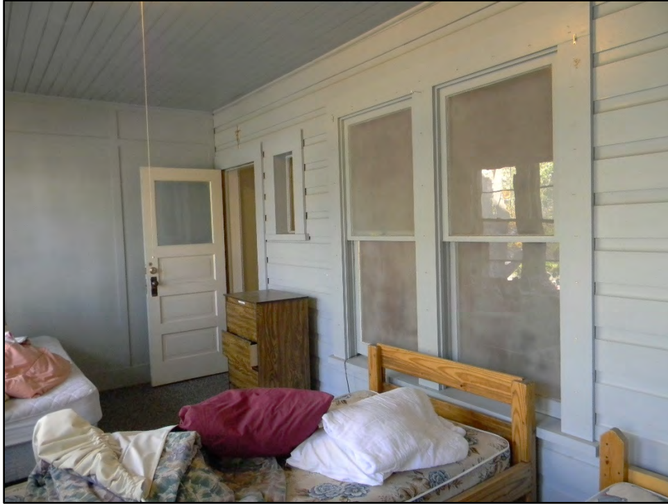
Figure D-461. Overview of the interior of the sleeping porch looking back toward the laundry room door, showing the original drop siding of the expansion completed between 1910 and 1916 by David Babbitt.
