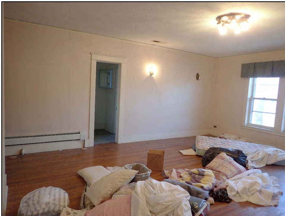
Figure D-410. A view toward the laundry room, which is located on the west side of the third bedroom (note the modern electric baseboard heater and ceiling register in this room).
