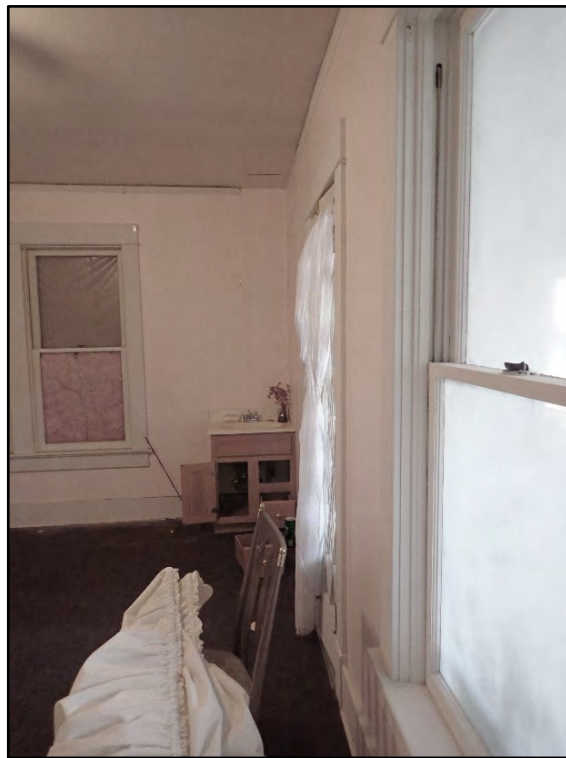
Figure D-422. View along the north wall of the interior bedroom.
