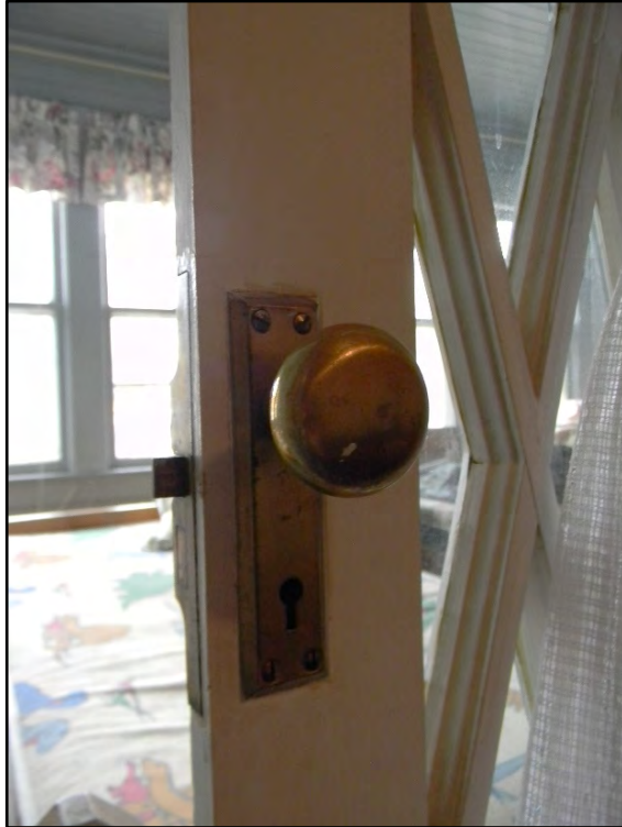
Figure D-429. A close-up view of the original doorknob of the French doors to the sleeping porch.
