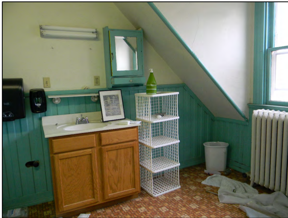
Figure D-528. View of the large bath (east wall), showing the wood wainscoting and other decorative details original to the bathroom when constructed by 1901.
