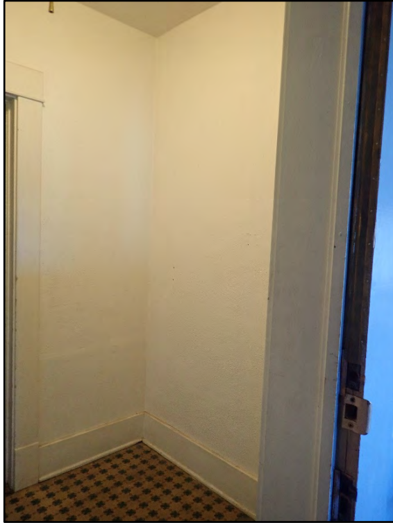
Figure D-447. The southwest corner of the laundry room (door jamb of the interior hallway to the left).
