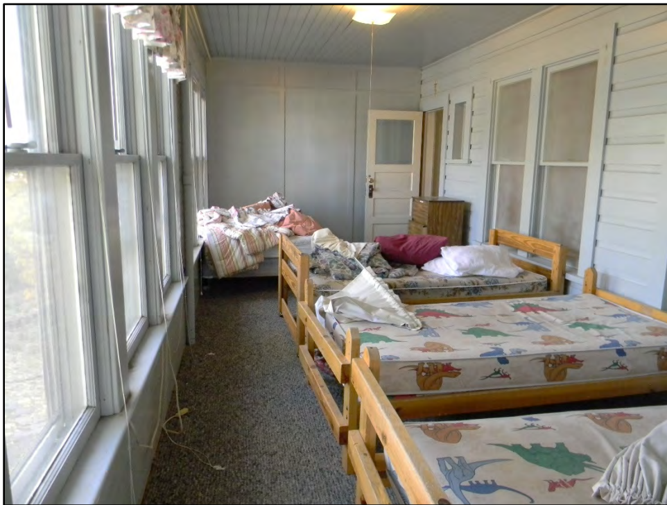
Figure D-466. View back toward the east side of the sleeping porch.
