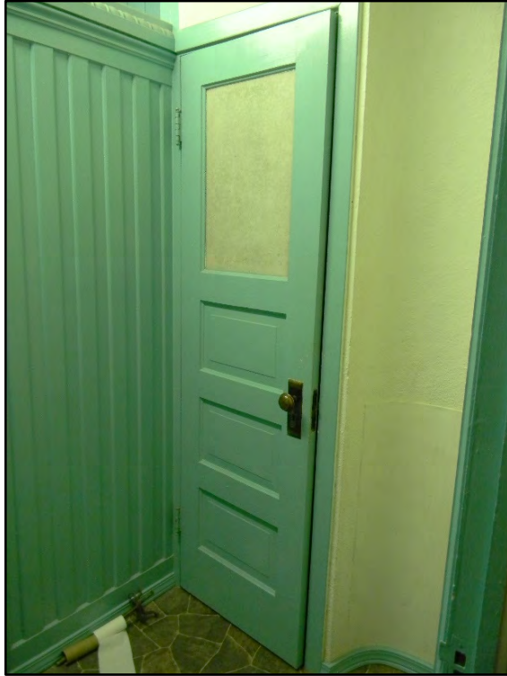
Figure D-513. A view of the door to the small toilet area, which is part of the original construction of the large bath (completed by 1901).
