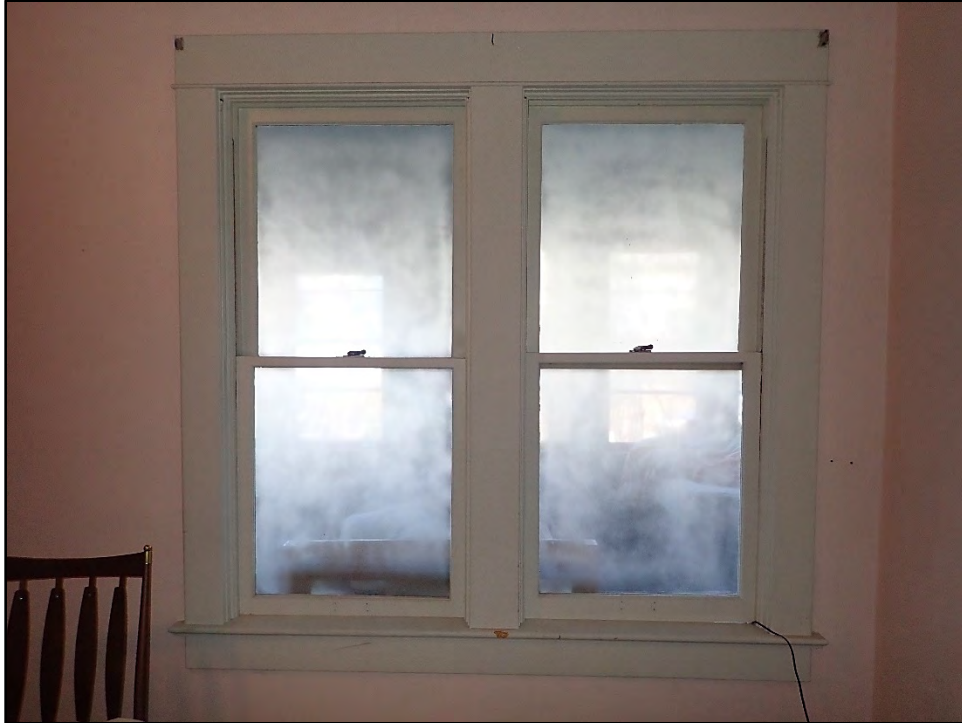
Figure D-421. Detail view of the formerly exterior, wood-frame windows of the interior bedroom, spray painted over to obscure the view.
