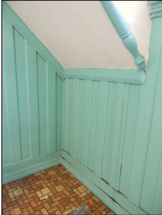
Figure D-529. Detail view of the decorative wainscot panels and corner accents.
