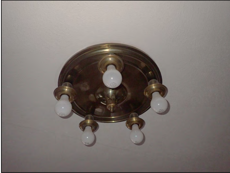
Figure D-407. The brass ceiling light fixture in the third bedroom.
