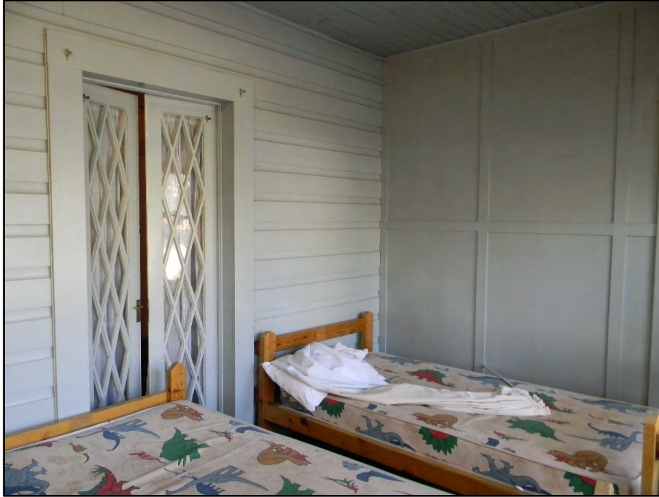
Figure D-465. View of the corner of the sleeping porch, revealing the wood construction as built between 1910 and 1916.
