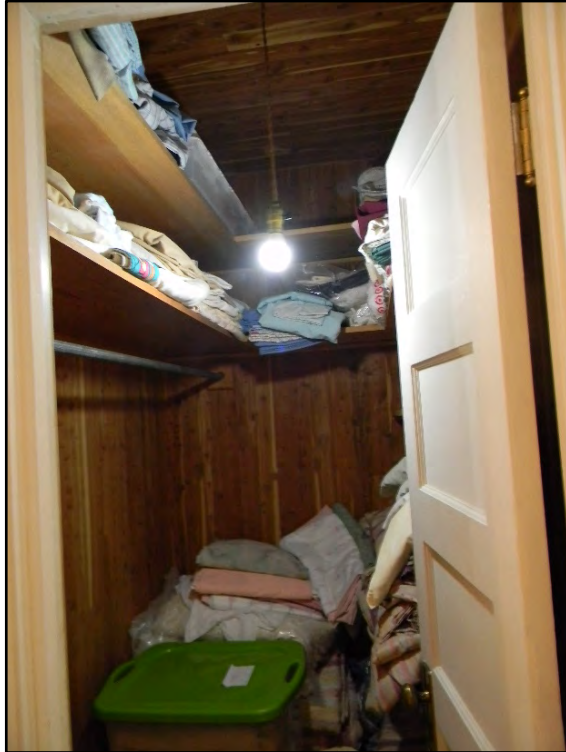
Figure D-401. Unlike the other closets, the interior of this one is unfinished and highlights its wood construction.
