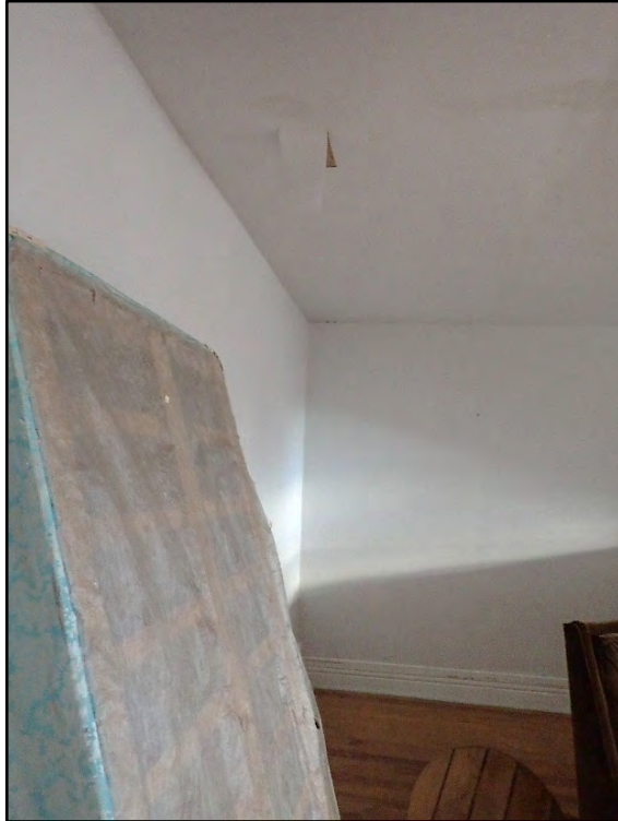
Figure D-551. A view of the opposite corner on the east wall of the bedroom.
