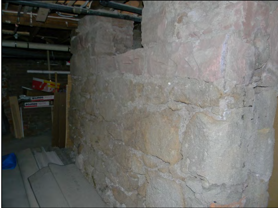
Figure D-647. Another section of masonry wall in the basement representing the extent of the house as seen in the 1906 photographs in Appendix B.
