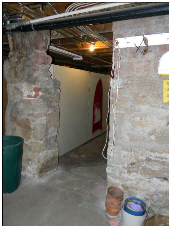
Figure D-642. An opening through the original sandstone masonry walls that were completed by 1901 when David Babbitt expanded his residence.
