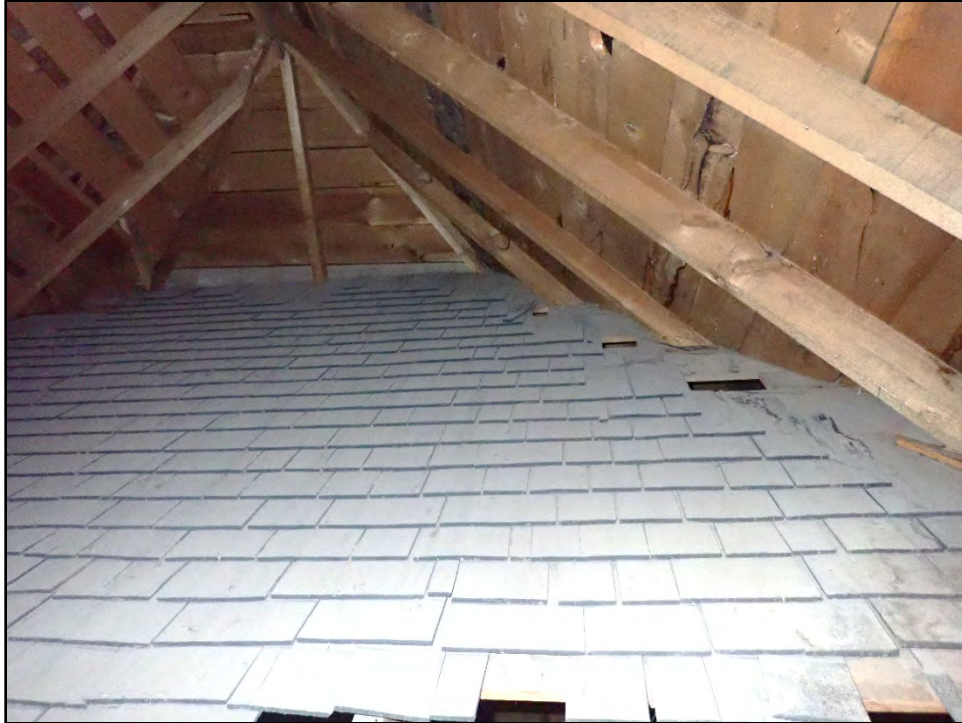
Figure D-593. The original hipped roof and wood shingles seen in the 1906 photographs (see Appendix B) hide beneath the roof expansion that was completed by 1916.
