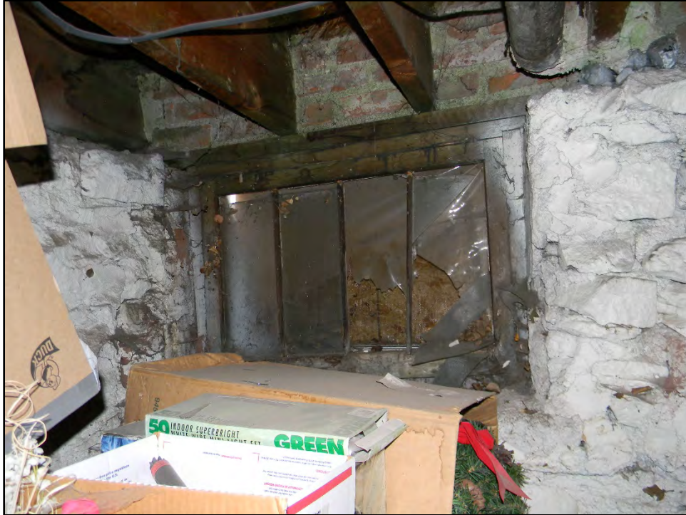
Figure D-635. A detail view of the former exterior window now boarded up below the dining room area (note the brick stem wall above).
