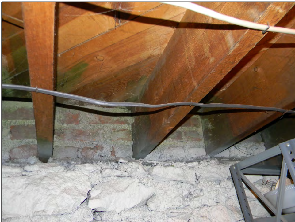
Figure D-636. Alternative view of the brick stem wall supporting the floor joists of the dining room.
