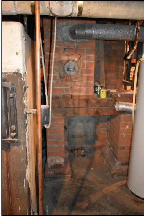
Figure D-617. The chimney that extends down to the basement as seen on the third floor terminates here, behind the metal door at the center of this image.
