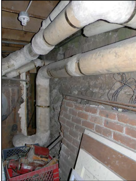
Figure D-623. Areas of the basement also exhibit sections of brick retaining walls, as seen here.
