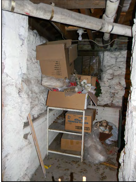
Figure D-633. A portion of the basement below what is now the dining room.
