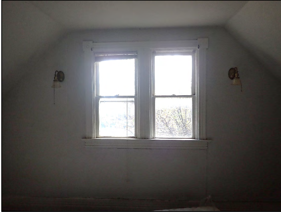
Figure D-571. A detail view of the windows of the large upper gable.
