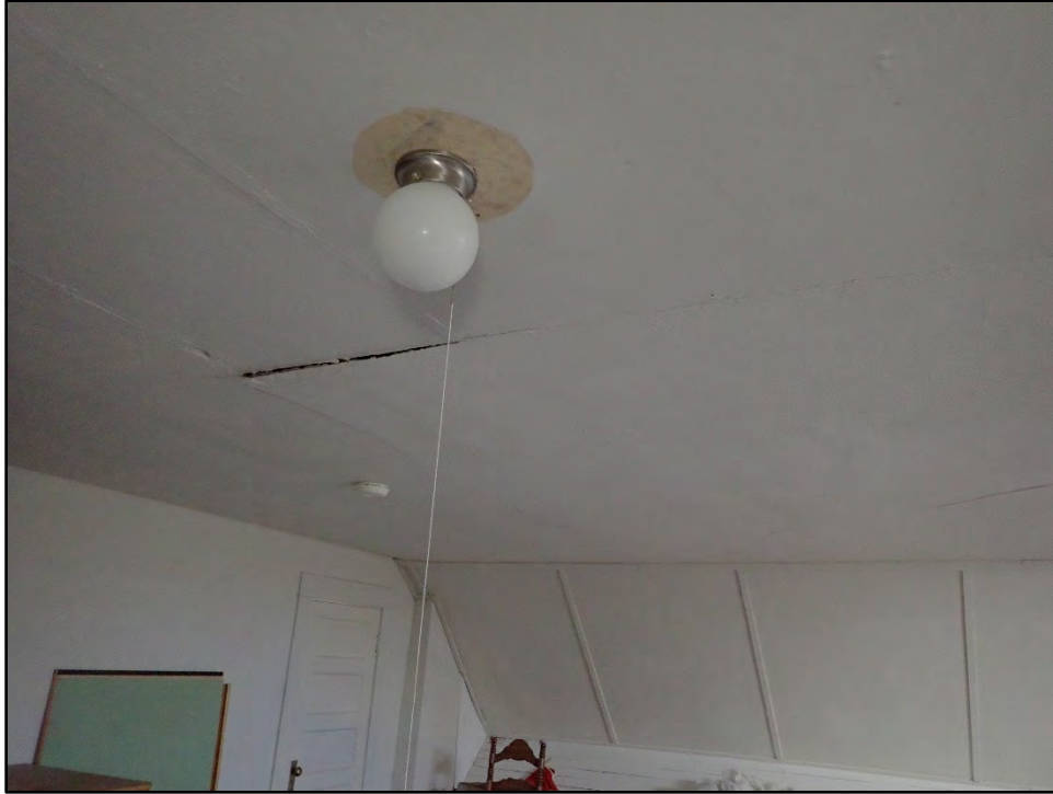
Figure D-603. View of the ceiling and the modern light fixture at the center of the room.
