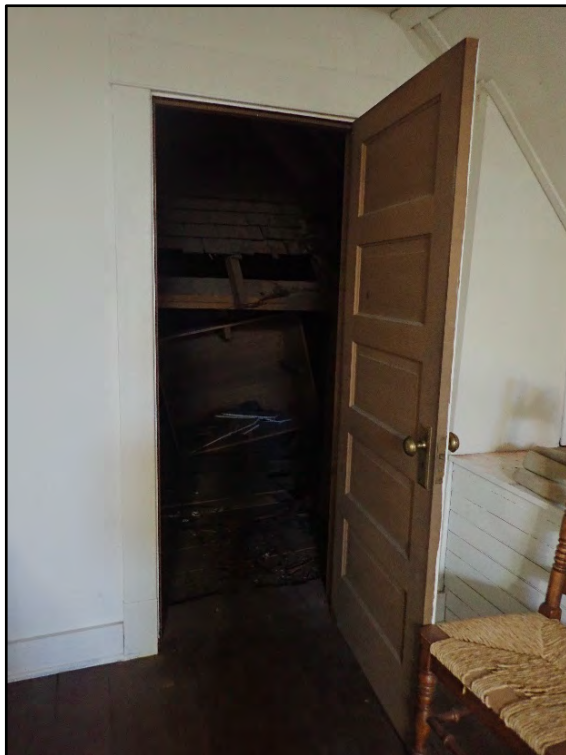
Figure D-592. A peek into the dark void of the third floor.
