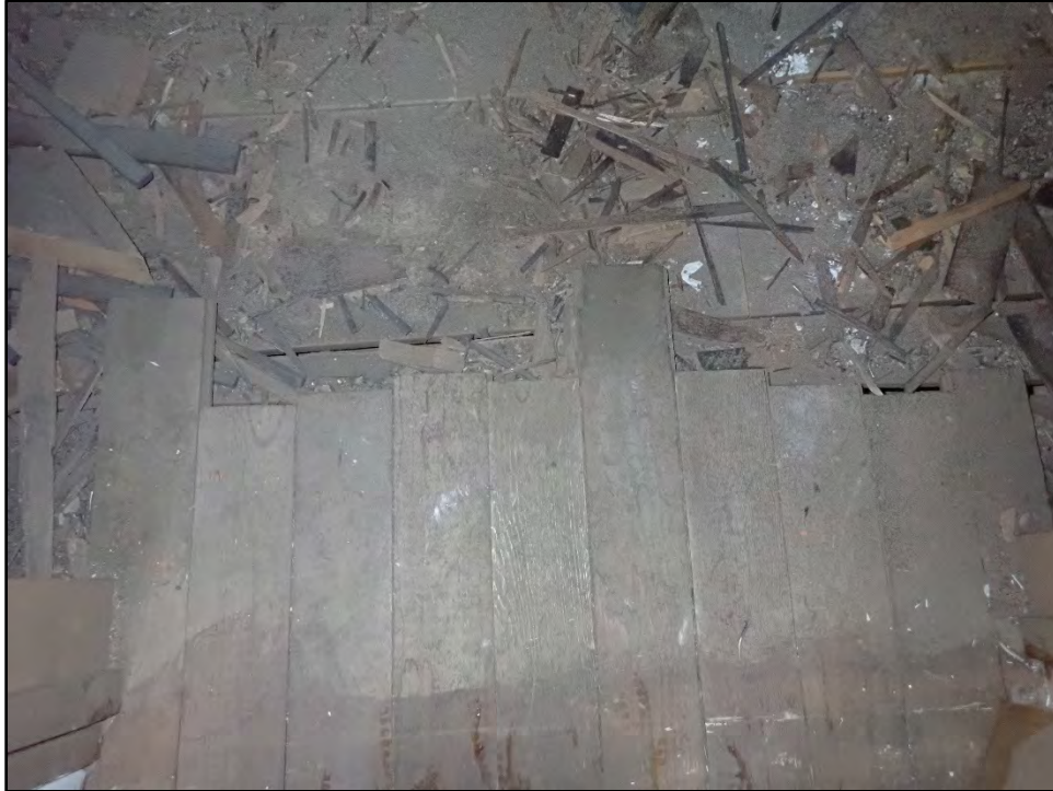
Figure D-599. Detail view of the original hardwood floor of the third floor as it extends into the attic space.
