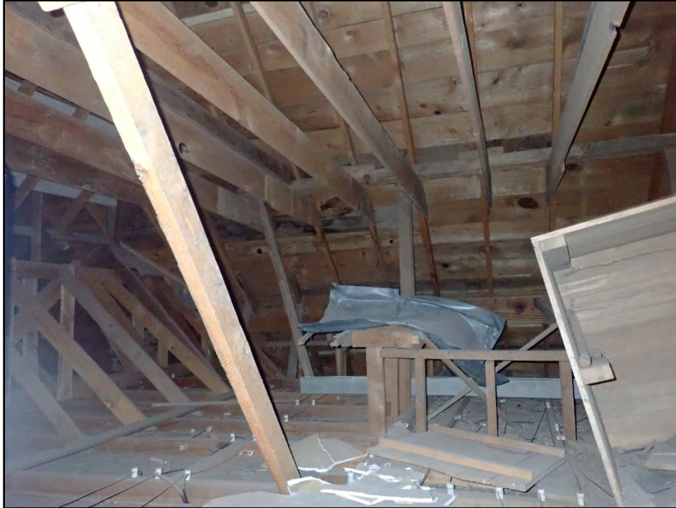
Figure D-595. Additional view of the roof framing as well as the historic-era electrical wiring in the attic space.
