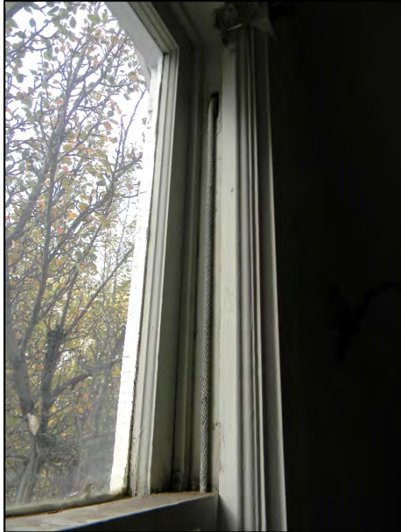
Figure D-573. A close-up view of the window mechanism that opens the lower sash via a rope.
