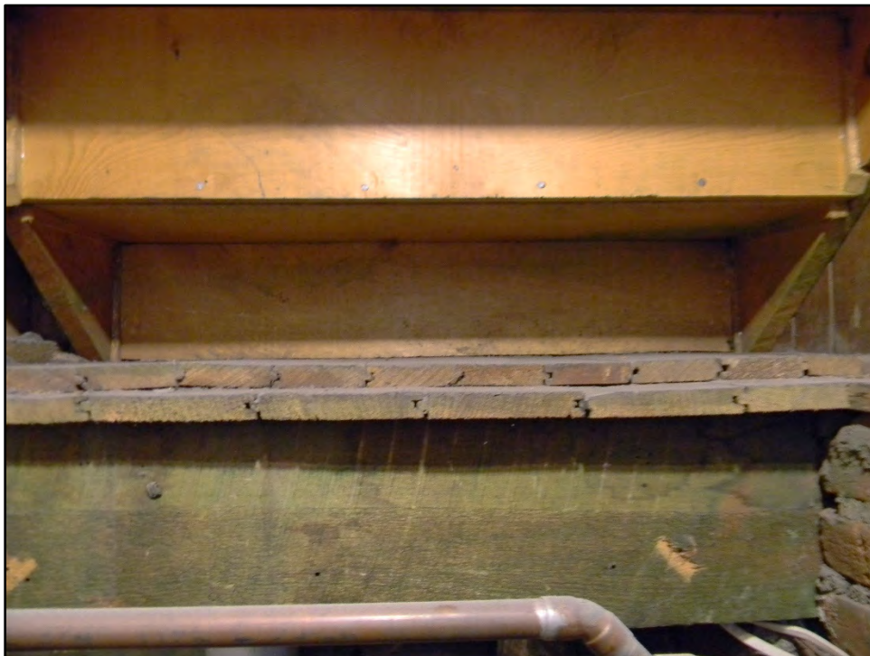
Figure D-614. Close-up view of the original hardwood floors of the entrance hall as extended under the main staircase.
