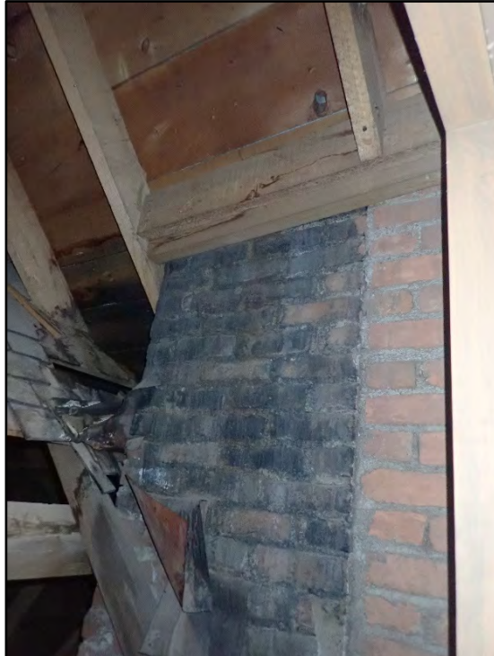
Figure D-597. A view of the double chimney that is visible in the 1906 photographs (one on the left goes to the basement while the other is for the fireplace in the formal living room).
