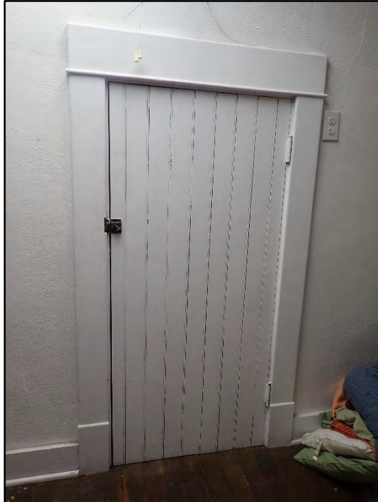
Figure D-579. The batten door at the top of the stairs, also trimmed with care.
