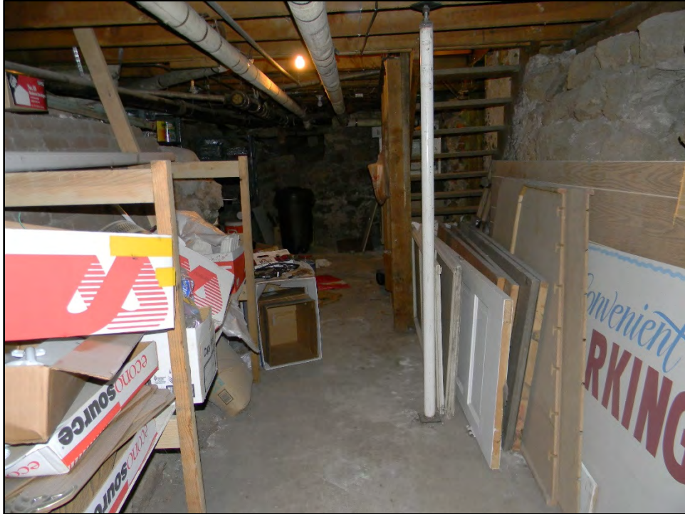
Figure D-655. View toward the center of the residence (eastern portion of the partial basement) with the stairs up to the first floor shown.
