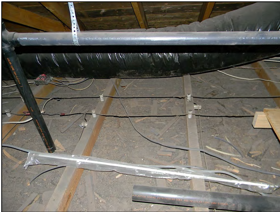
Figure D-584. The original twentieth century electrical wiring is visible here.
