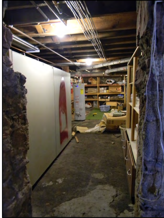
Figure D-643. An additional view through the same wall opening toward the east side of the partial basement.
