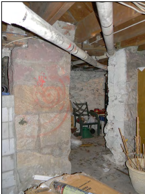
Figure D-632. The structural sandstone walls likely constructed when the house was expanded between 1895 and 1901.
