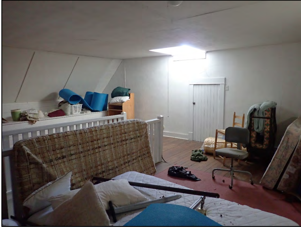
Figure D-601. Overview of the interior as seen from the northeast corner.
