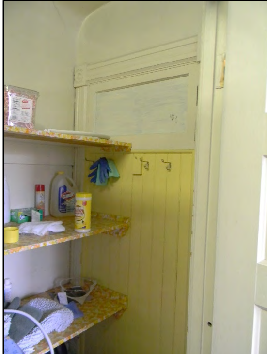
Figure D-541. The far wall of the small closet reveals what was once a door with an upper glass pane, which now leads to a small hall closet in the main hallway.
