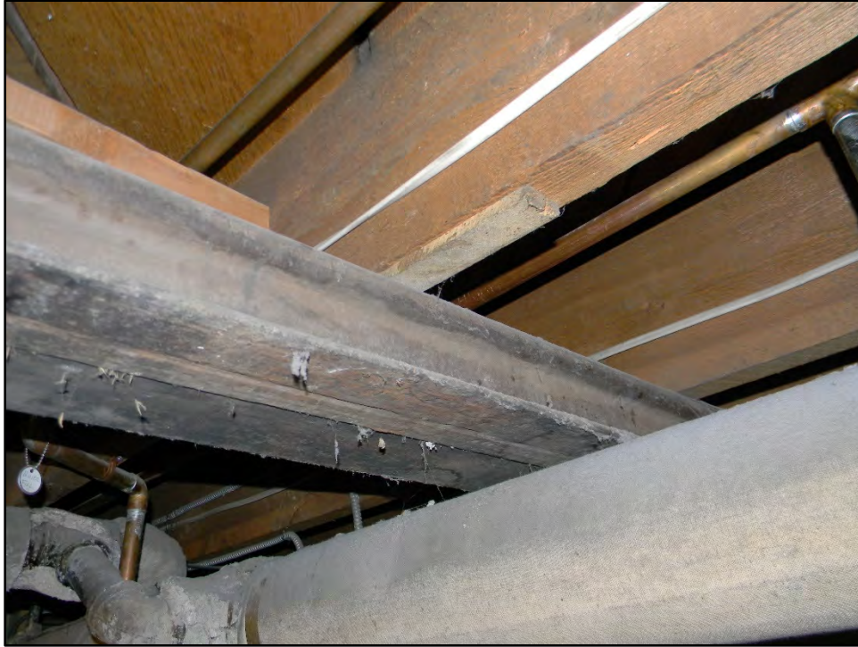
Figure D-625. Sections of steel rail have been incorporated into the structural framework of the basement.
