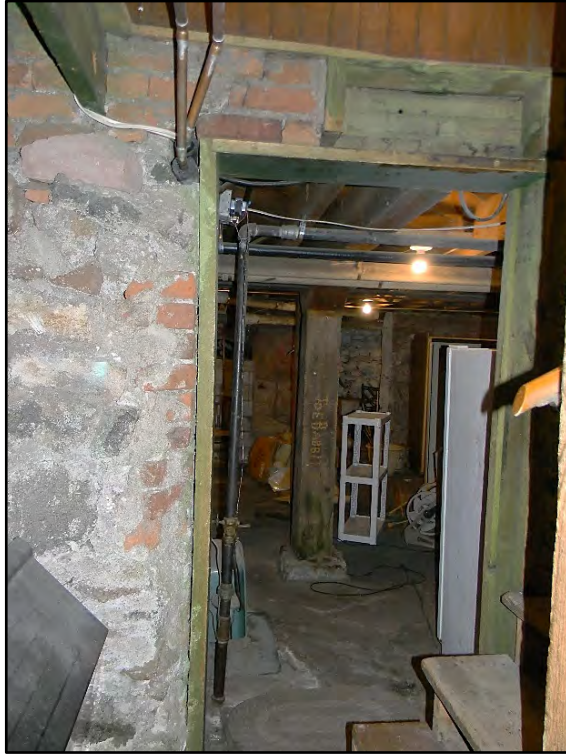
Figure D-615. A peek into the main area of the partial basement beyond the stairs.
