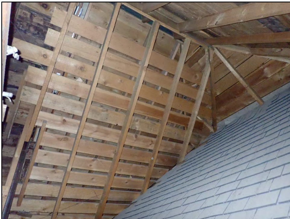
Figure D-594. The plank-and-rafter construction of the roof as completed between 1910 and 1916 when David Babbitt expanded his residence, which has protected the original roof for well over 100 years.
