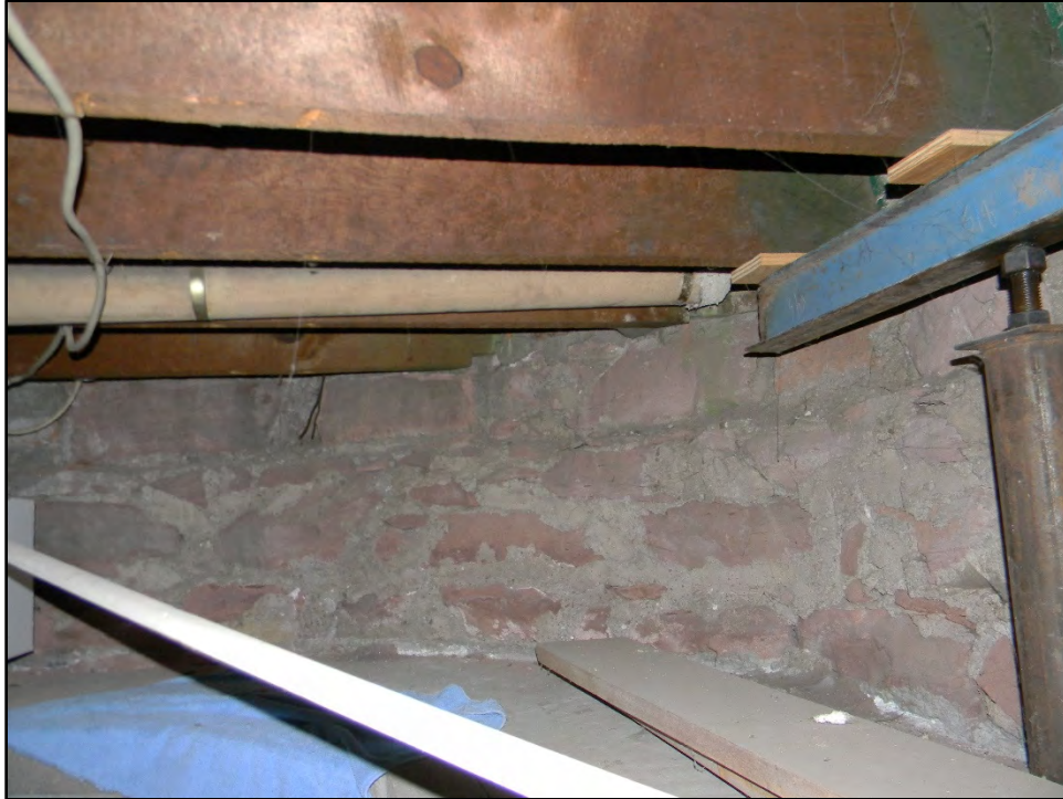
Figure D-629. A peek behind the Moenkopi red sandstone stem wall of the cant bay window that supports the floor system of the formal living room.
