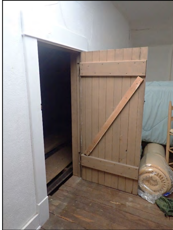
Figure D-583. The batten door with diagonal bracing that provides a peek into the construction of the home between 1910 and 1916.
