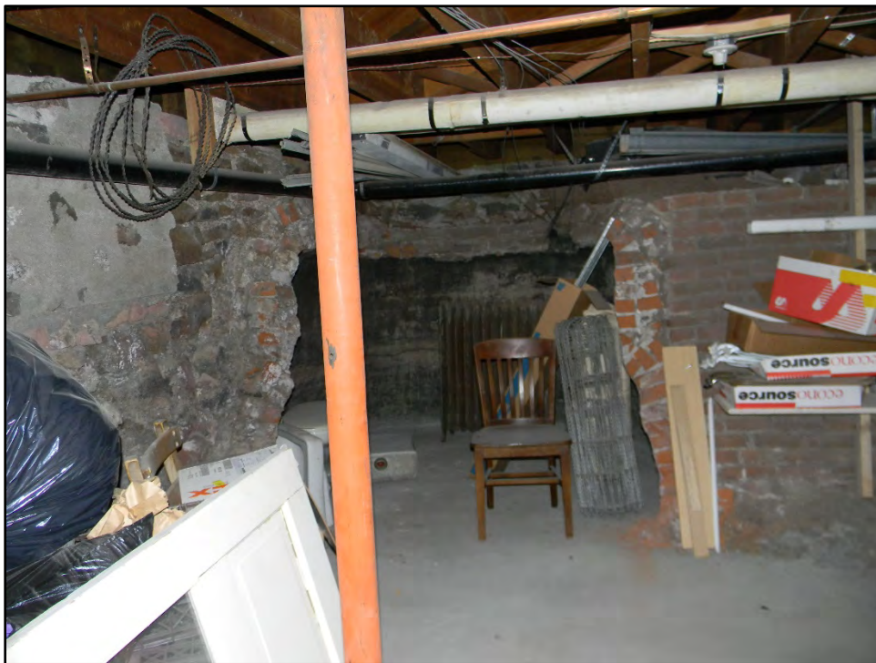
Figure D-648. A view facing what is likely the circular well/cistern seen on the 1895 Sanborn map on the west side of the residence.
