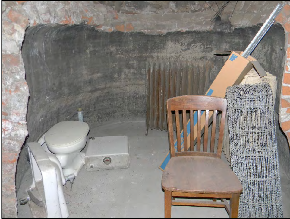
Figure D-649. Detail view of what may have been the original well, now filled in with concrete and covered up by the last major extension of the residential footprint (completed by 1916).
