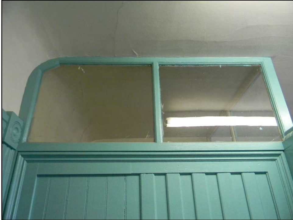
Figure D-539. Detail view of the upper glass panels of the small closet, indicating the space was likely intended to be used and occupied because of the need for interior light.
