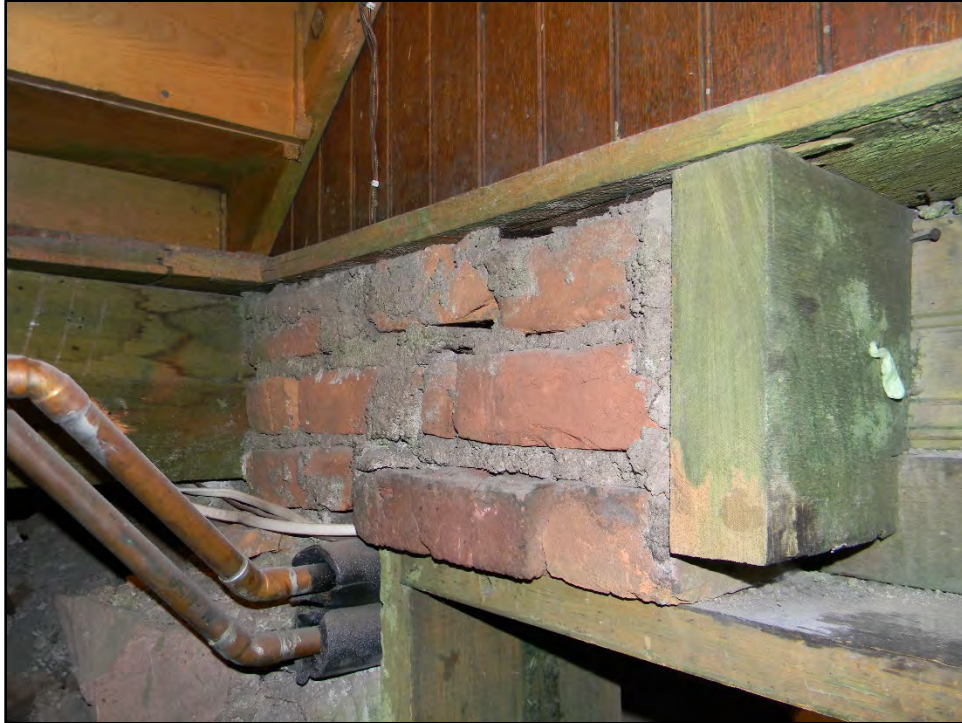
Figure D-613. A close-up view of the wood framing and brick construction under the main staircase to the second floor as seen within the basement.
