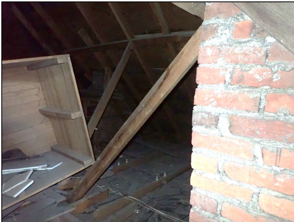
Figure D-596. A look behind the chimney into the southern portion of the third floor attic space.
