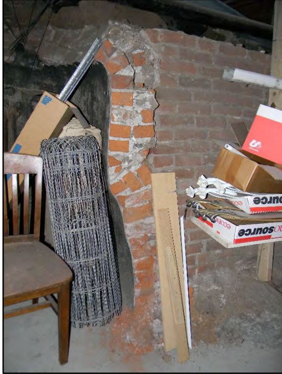
Figure D-653. The intriguing profile of the walls of the former well/cistern are evident here, as is the historic-era brick construction adjacent.
