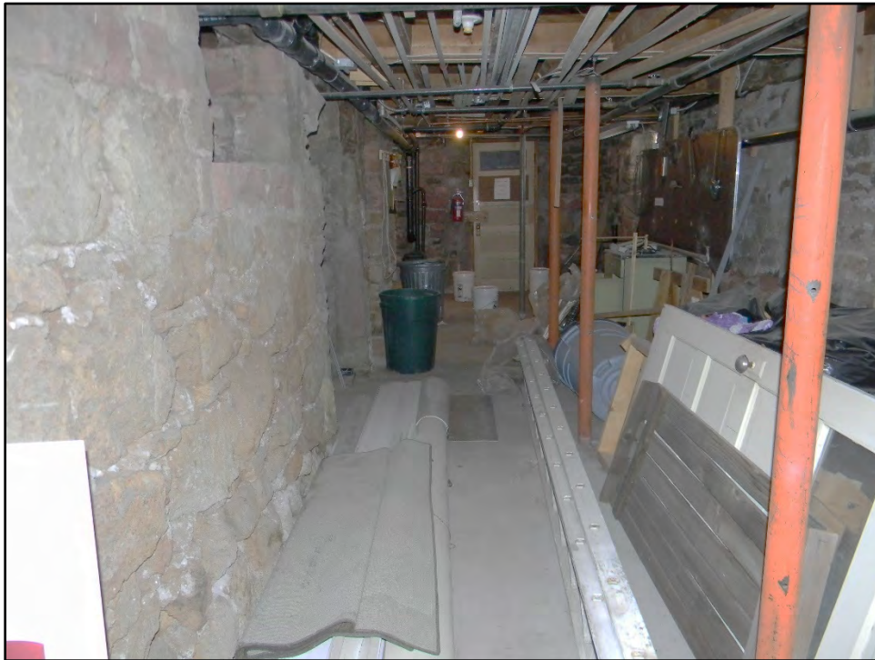
Figure D-654. A glance back down the west side of the residence as seen in the basement, with the 1901 extent of the house on the left in this image.
