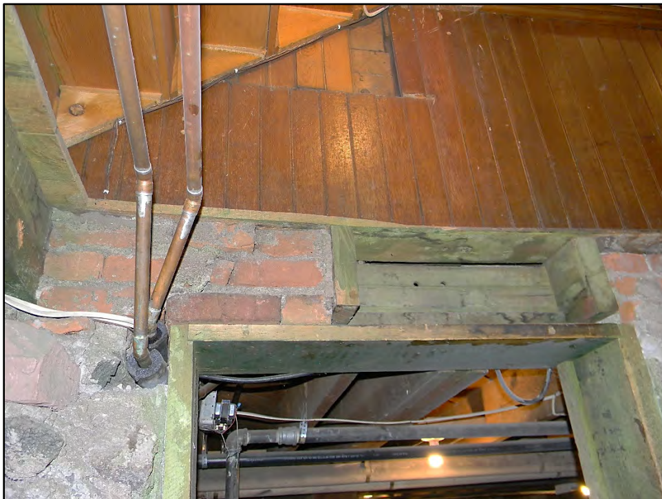
Figure D-612. A look at the framing and building materials of the partial basement and under the main staircase.
