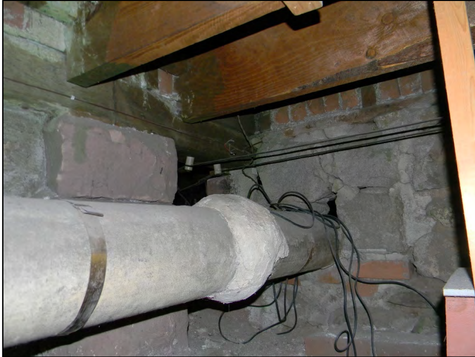
Figure D-621. A hodgepodge of old and new as seen in the basement.
