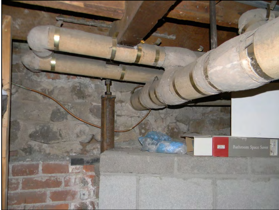
Figure D-627. The patchwork of materials is also illustrated here with the historic-era wood, rubble-and-mortar, and brickwork, with the modern concrete block retaining wall (note the shoring jack at the back).
