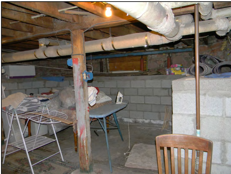
Figure D-628. The shape of the cant bay above of the formal living room can be seen here in the basement, which has been reinforced by a modern concrete block retaining wall.
