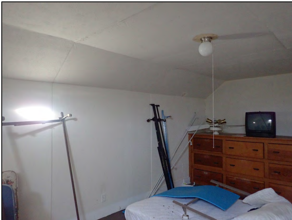
Figure D-604. The removal of a substantial section of original wall on the third floor is indicated by the outline of the modern drywall, upgraded electrical outlet and ceiling light fixture.
