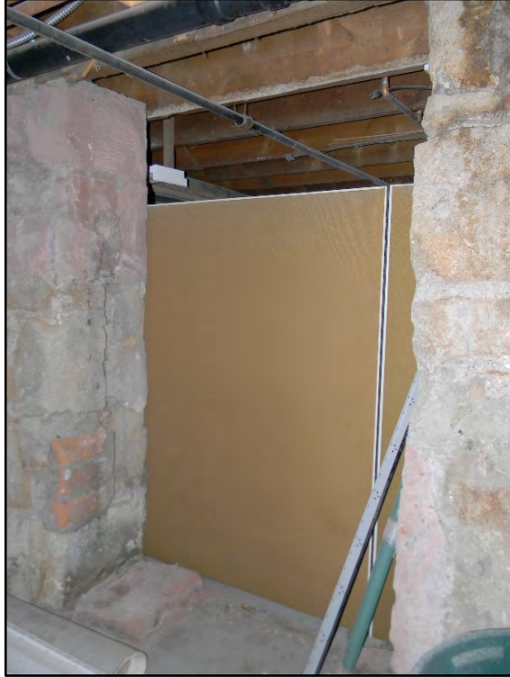
Figure D-645. A modular wall is seen through an opening in the 1895–1901 basement wall.
