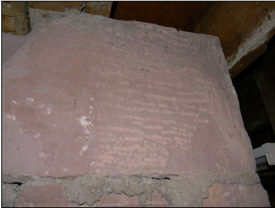
Figure D-646. The workmanship of the construction of this portion of the basement (completed by 1901) is still clearly visible today.
