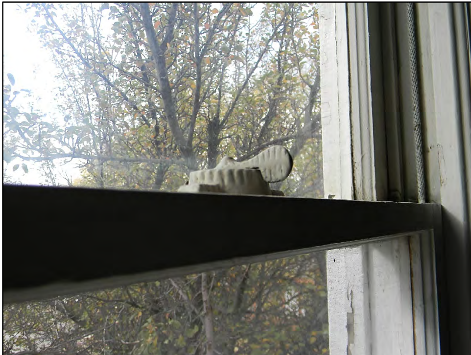
Figure D-572. A close-up view of the brass window latch.
