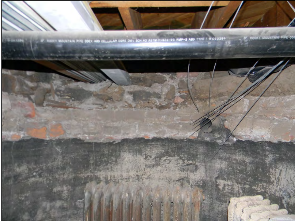
Figure D-651. An additional detailed view of the upper portions of the circular well/cistern in the basement.
