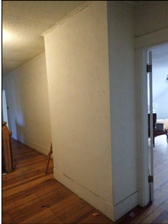
Figure D-547. Turning to the right, this wall represents two chimneys, one of which goes to the formal living room (the other down to the basement), with the door to the fourth bedroom on the right.
