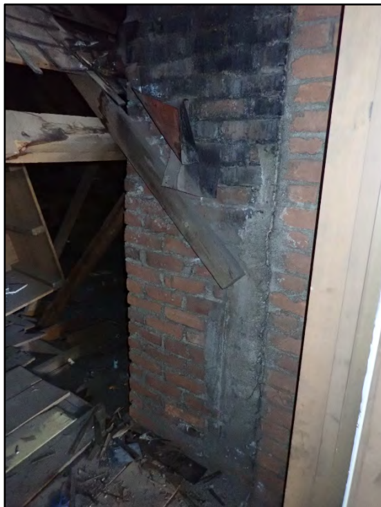
Figure D-598. This image shows how the original 1886 hipped roof (seen in some of the 1906 photographs) was configured.
