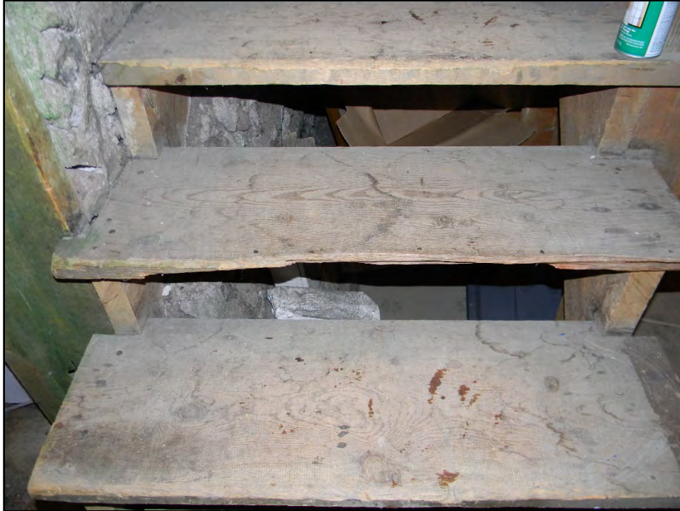
Figure D-611. Detail view of the stair treads, that likely date to the original construction of the home in 1886.
