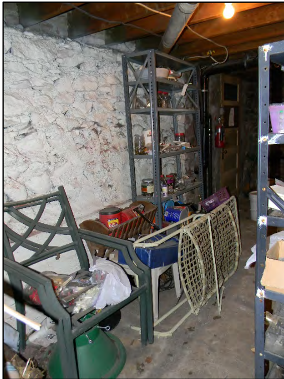
Figure D-634. Additional view of the space below the dining room (the masonry walls are painted).
