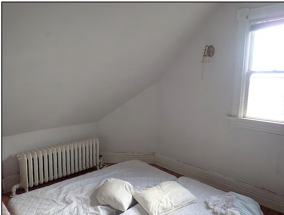
Figure D-554. View of the opposite corner, revealing the same canted shape, with the decorative trim around the windows and baseboards.
