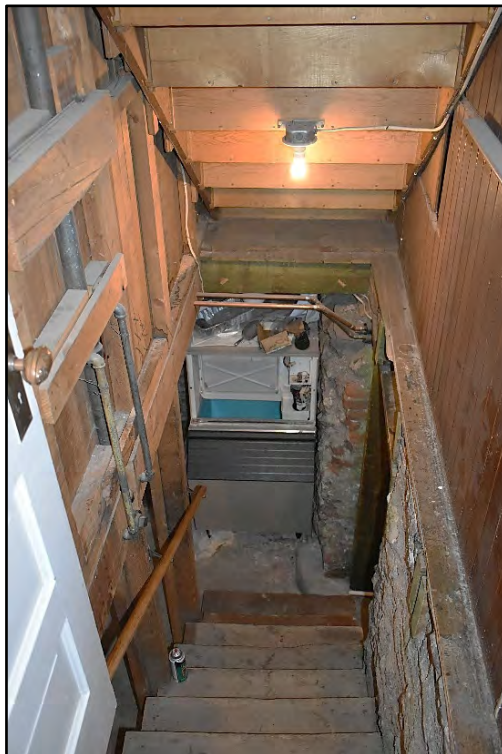
Figure D-610. The steps descending down into the partial basement.
