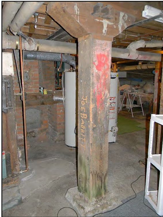
Figure D-616. The main basement support at the center of the basement.
