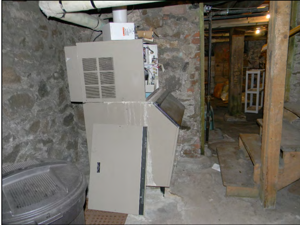
Figure D-667. An ice machine sits at the bottom of the stairs at the corner of the original basement wall dating to 1886.
