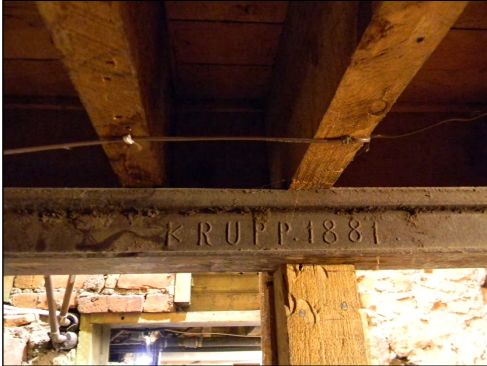
Figure D-669. A segment of steel rail from the Atlantic & Pacific railroad that first came through Flagstaff beginning in August 1882, incorporated into the post-and-beam construction of the 1886 residence.
