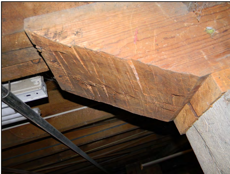
Figure D-670. A close-up view of the main basement support still shows the mark of the ax which shaped it over 130 years ago.
