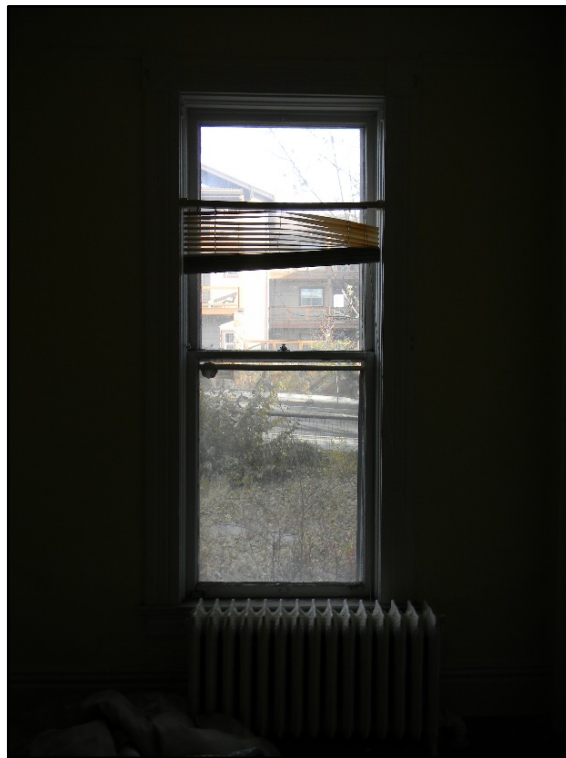
Figure E-24. The condominium complex (completed in 2018) is clearly visible through the window of the small corner bedroom (constructed in 1886) on the first floor.
