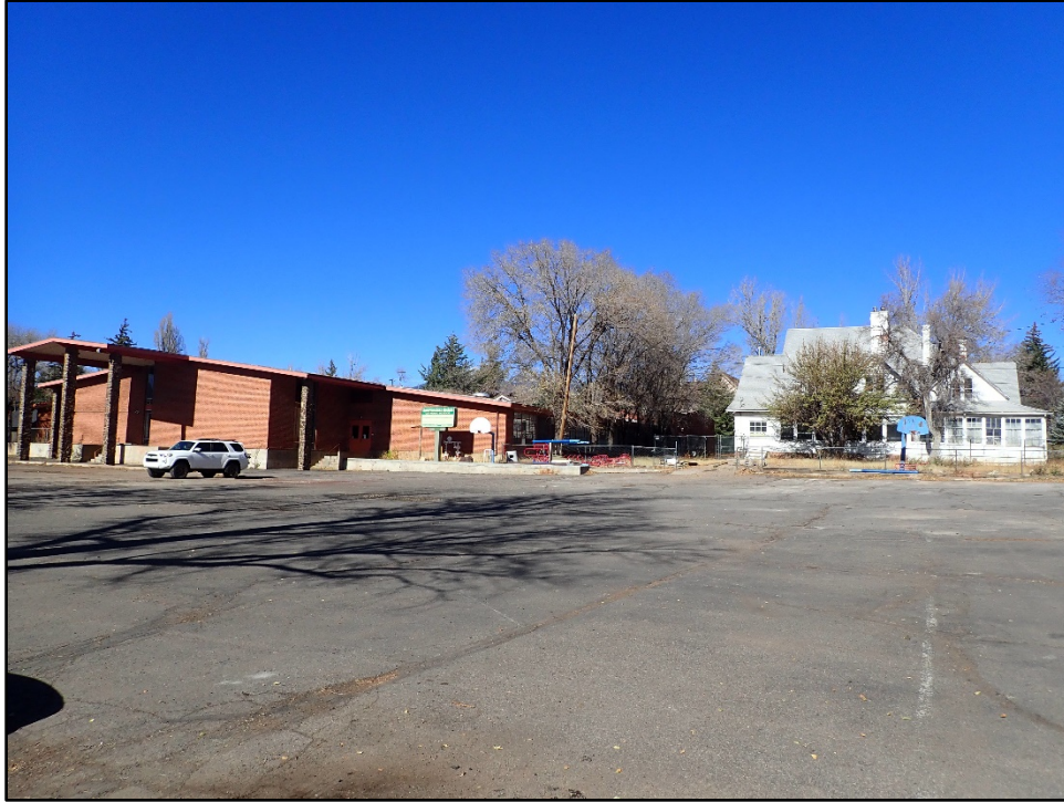
Figure E-13. Overview of the former Catholic school and the residence as seen from the large parking lot the extends over the entire south half of the block.
