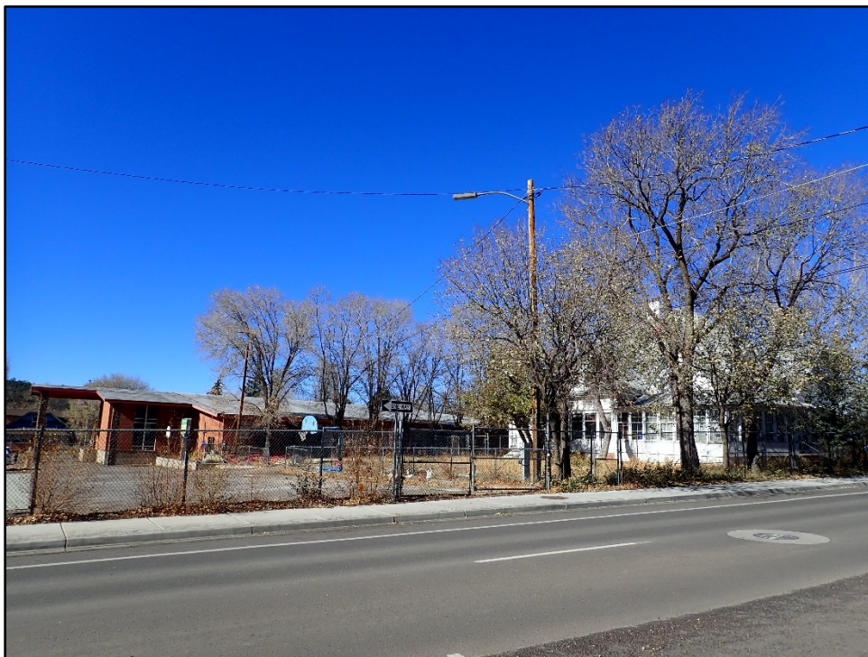
Figure E-4. Overview of the former Catholic school and the David Babbitt House as seen from the east side of North Beaver Street.
