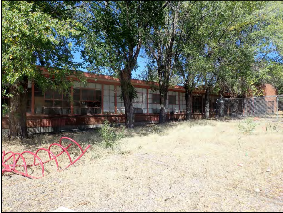
Figure 15. East elevation of the school building, showing the 1950s multiple-light metal windows that once lighted the classrooms.
