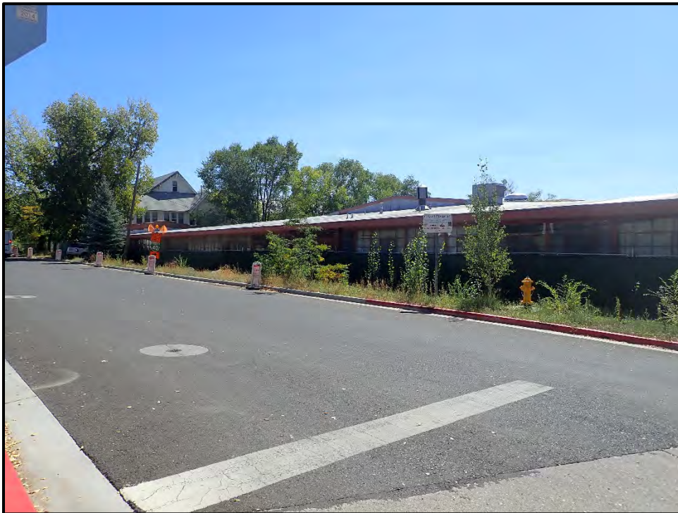
Figure 18. North elevation of the former school along West Dale Avenue.
