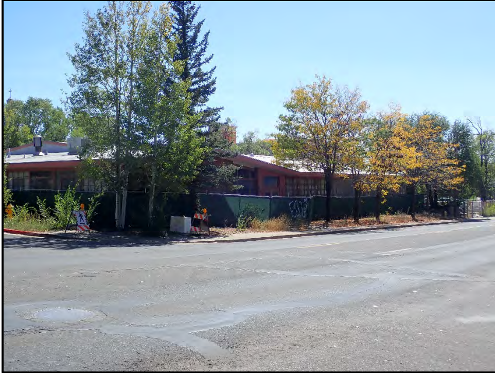
Figure 19. Portions of the north and west elevations of the school as seen from the intersection of West Dale Avenue and North Humphreys Street.
