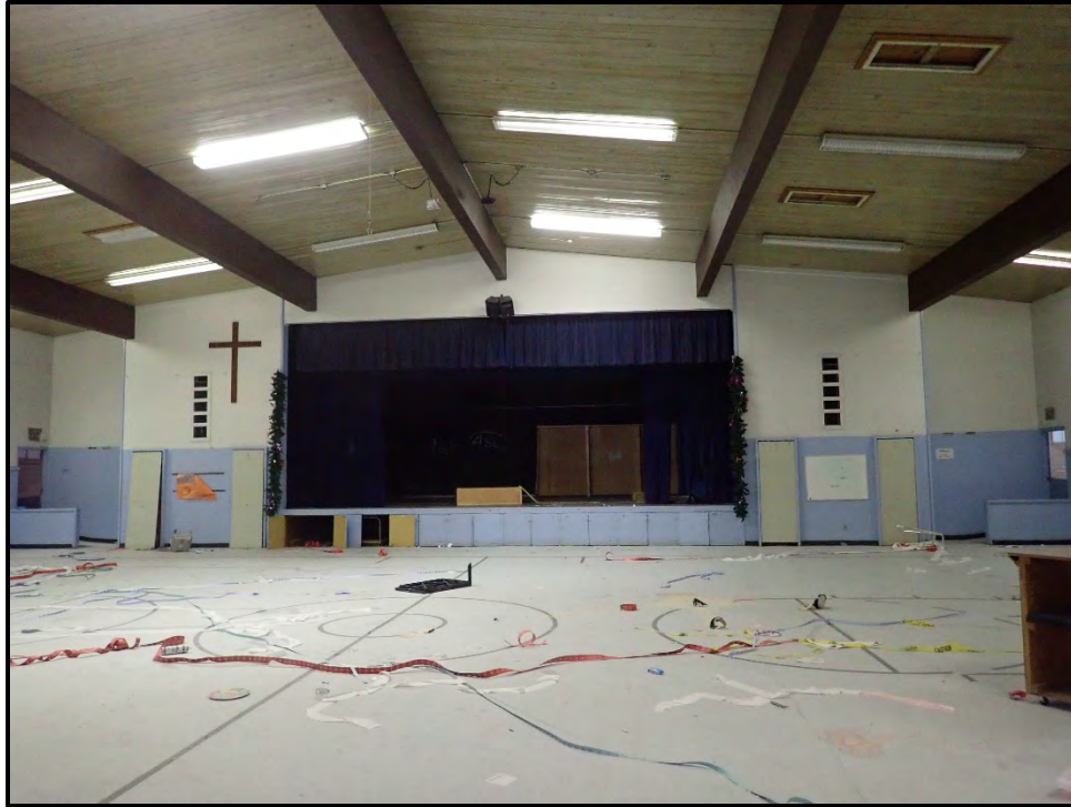
Figure 29. View of the theatre stage and the expansive interior of the full-size gymnasium that was constructed to convert the former classroom annex into St. Mary's Catholic School.
