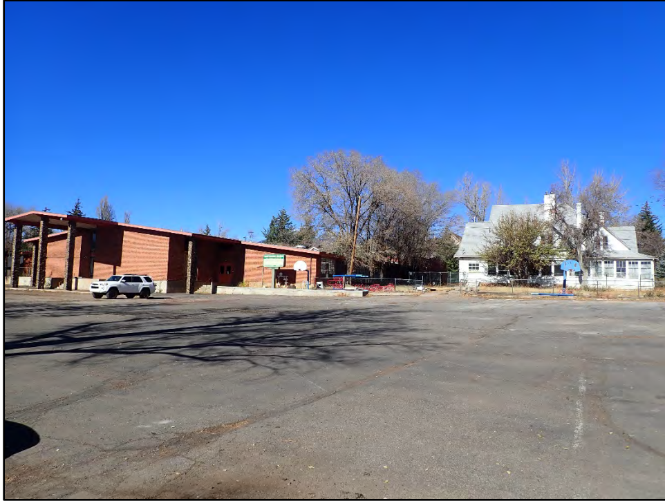
Figure B-19. Overview of the former Catholic School and David Babbitt House as seen from the parking lot.
