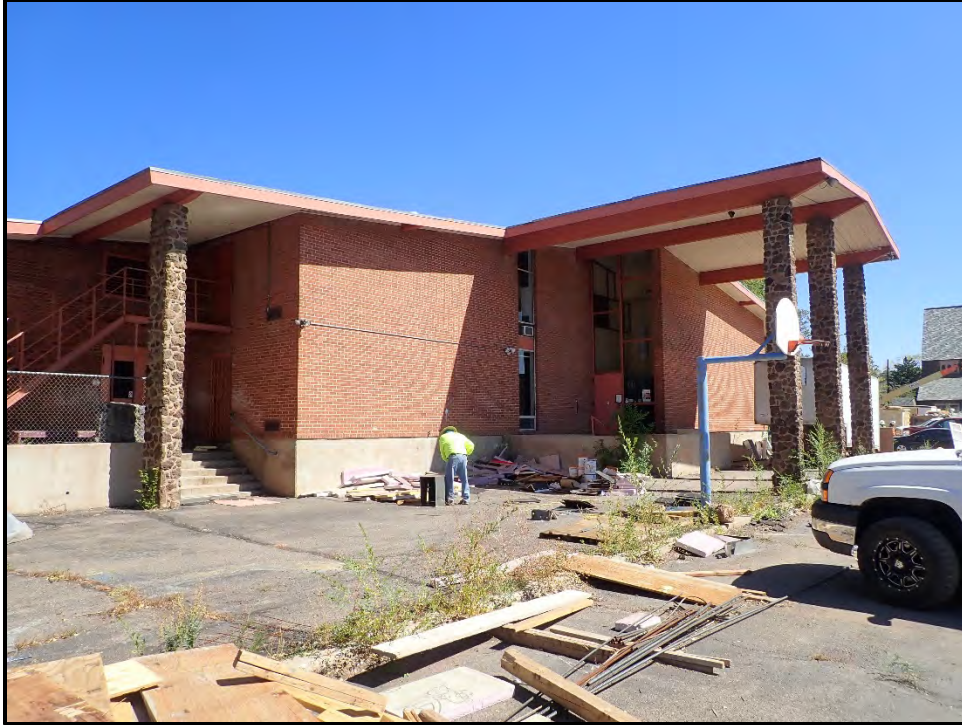
Figure 9. South elevation of the Catholic School building.
