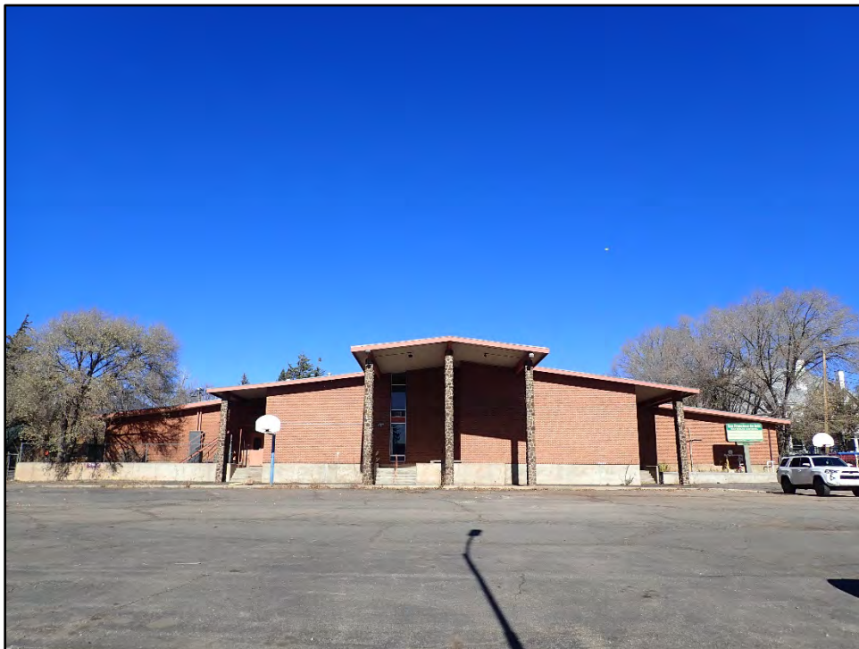
Figure B-16. A view of the south elevation of the former St. Mary's Catholic School with the parking lot now cleared of construction equipment and materials.
