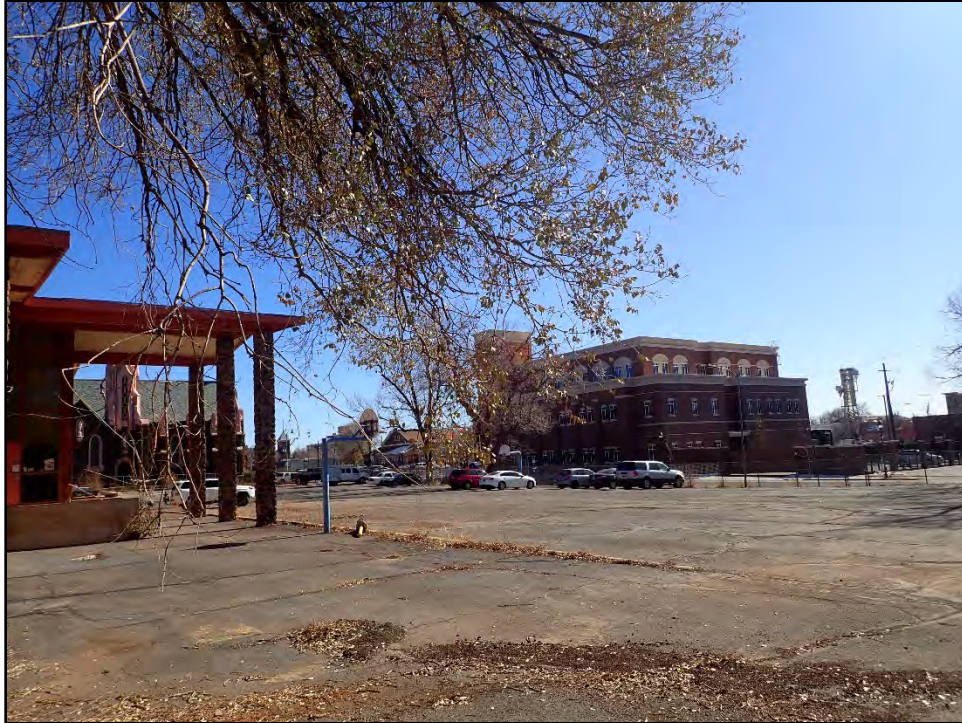
Figure B-11. An overview of the former Catholic school parking lot where the grand St. Anthony's Academy once stood until it was demolished in the late 1950s–early 1960s.
