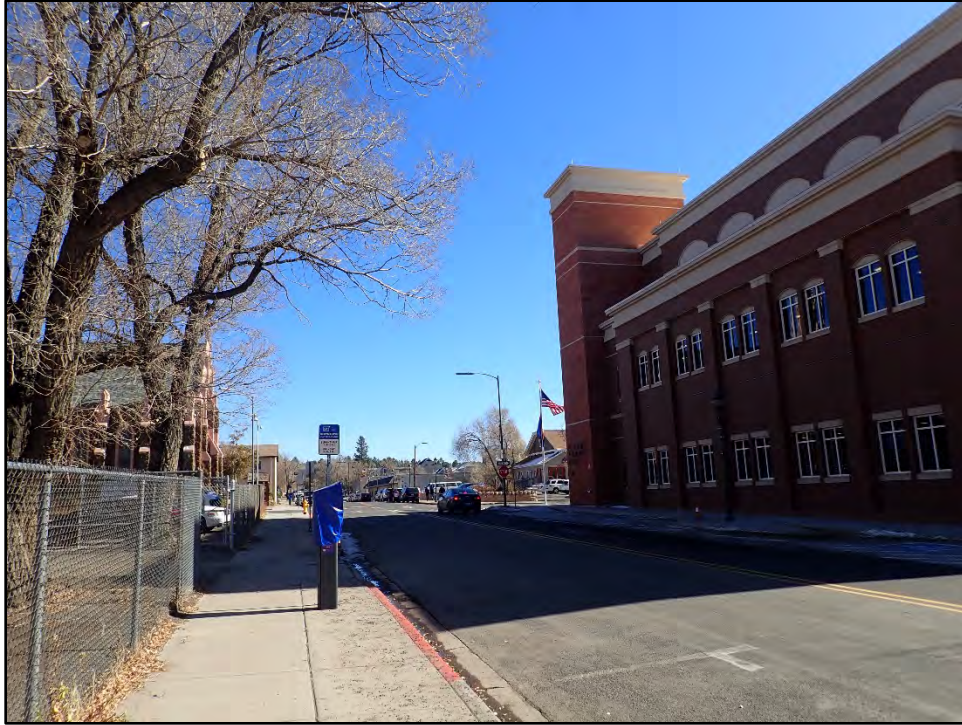
Figure B-17. West Cherry Avenue is now cast in shadow because of the new, multiple-story courthouse facility on the corner.
