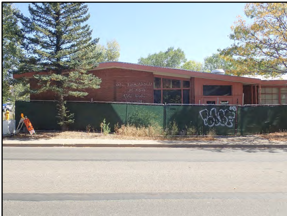
Figure 22. View of the entrance along North Humphreys Street, showing the low-pitched roof, window wall, and expanse of brick characteristic of the Contemporary style.
