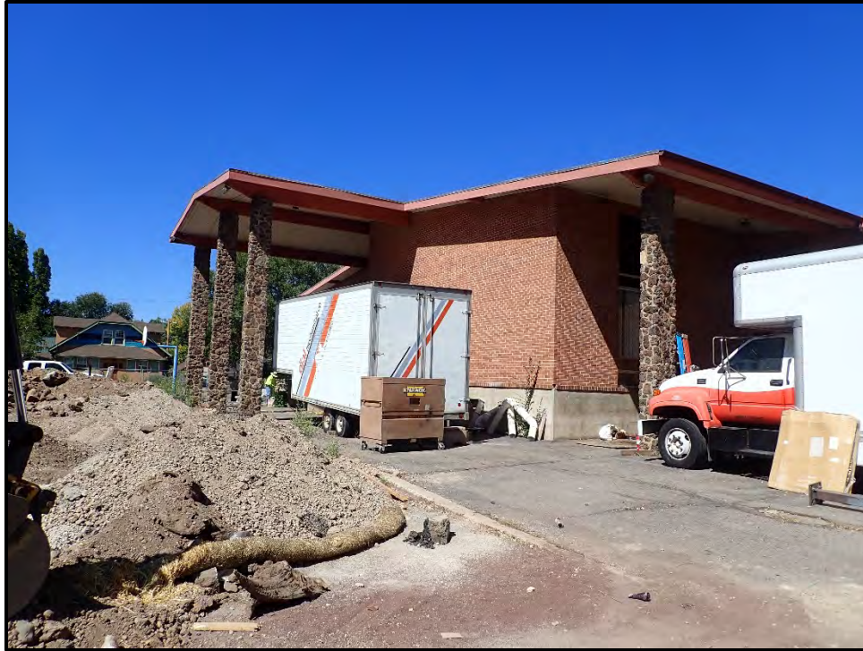
Figure 11. South elevation of the school building, showing the local malpais columns supporting the low-pitched, elevated roof of the entrance.
