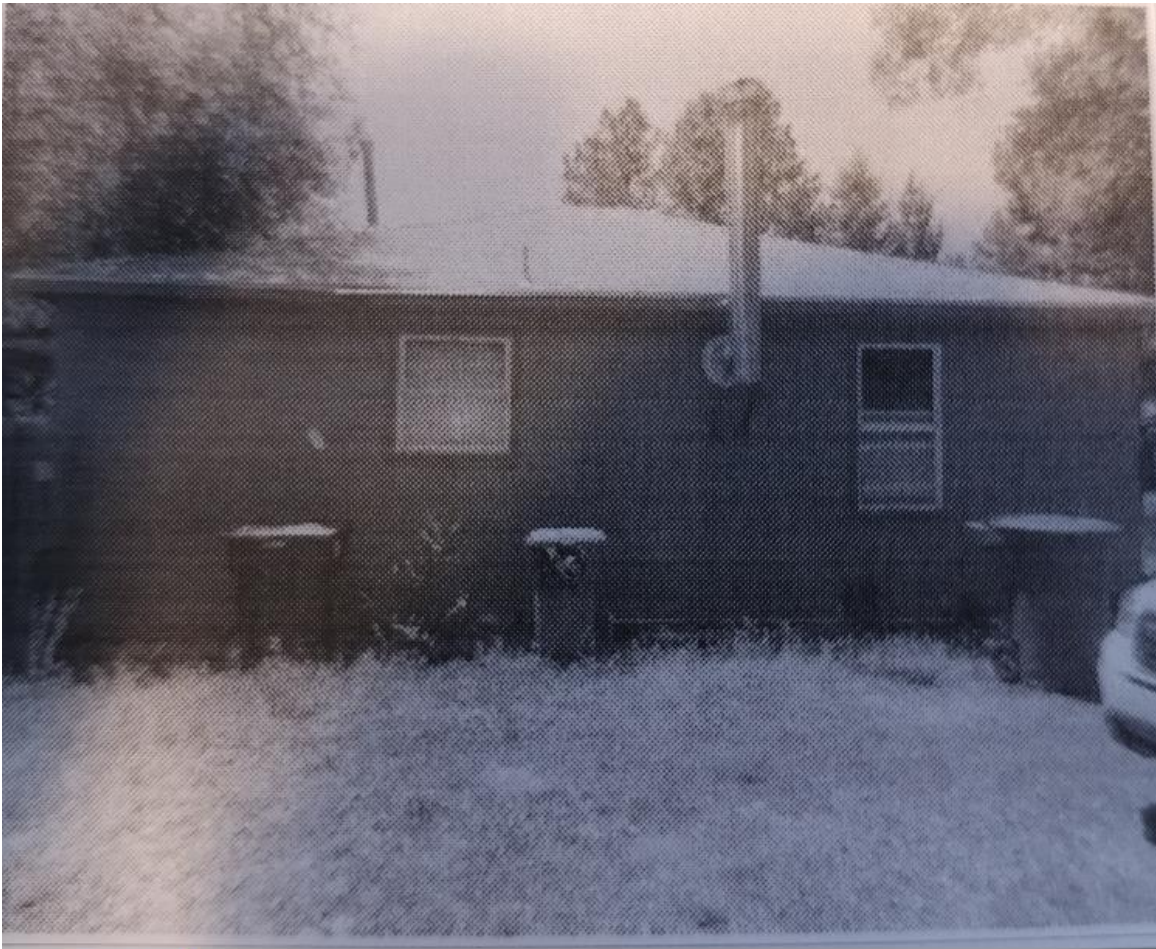
North side of house
