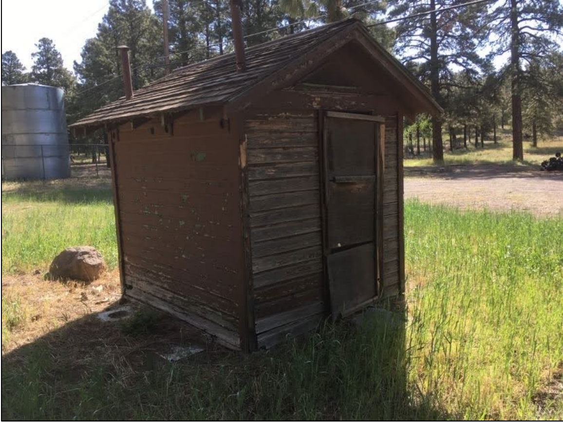
Figure 11. Overview of outhouse structure, looking east.
