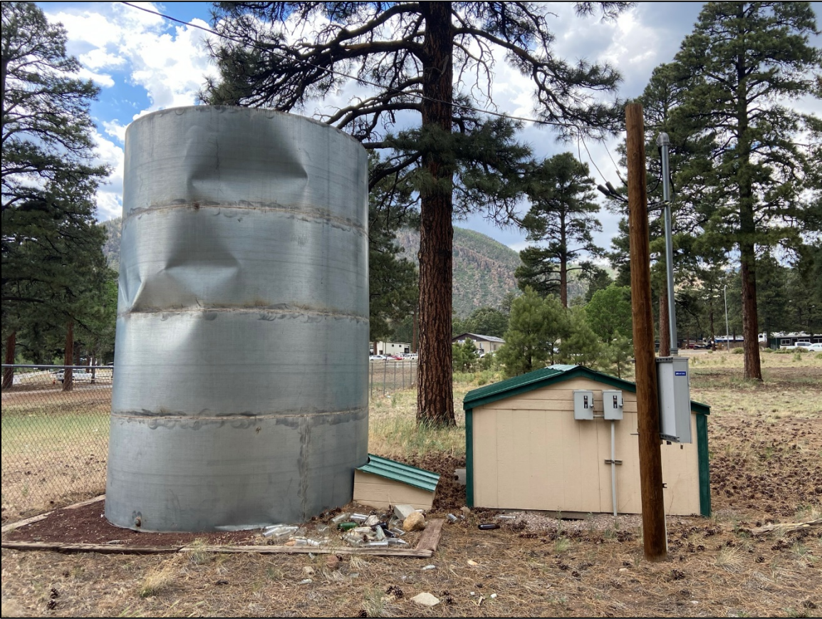
Figure 10. Overview of water tank, looking west.
