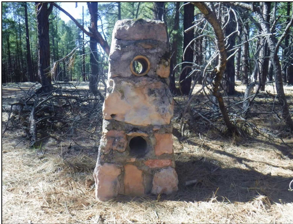
Figure 3. CW1, Detail of complete stone and mortar fencepost. 4/1/2021
