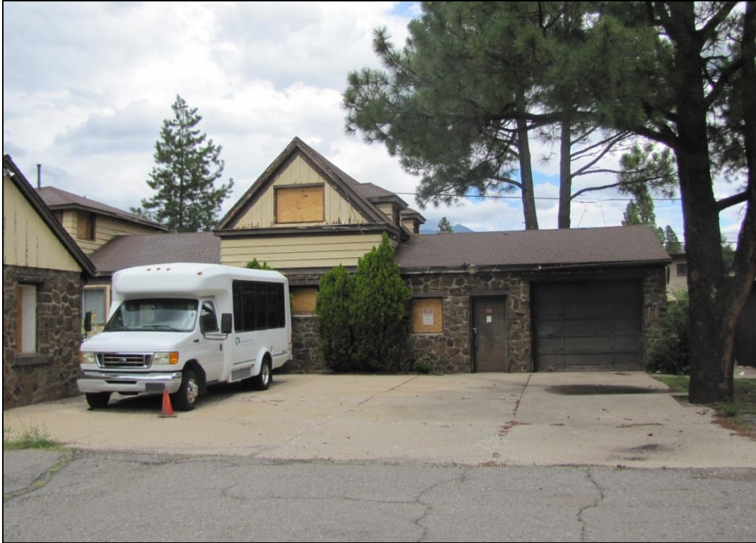
Photograph 21. East end of Main Building, facing north.
