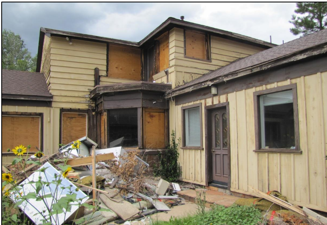
Photograph 18. Main Building and courtyard, facing northwest.
