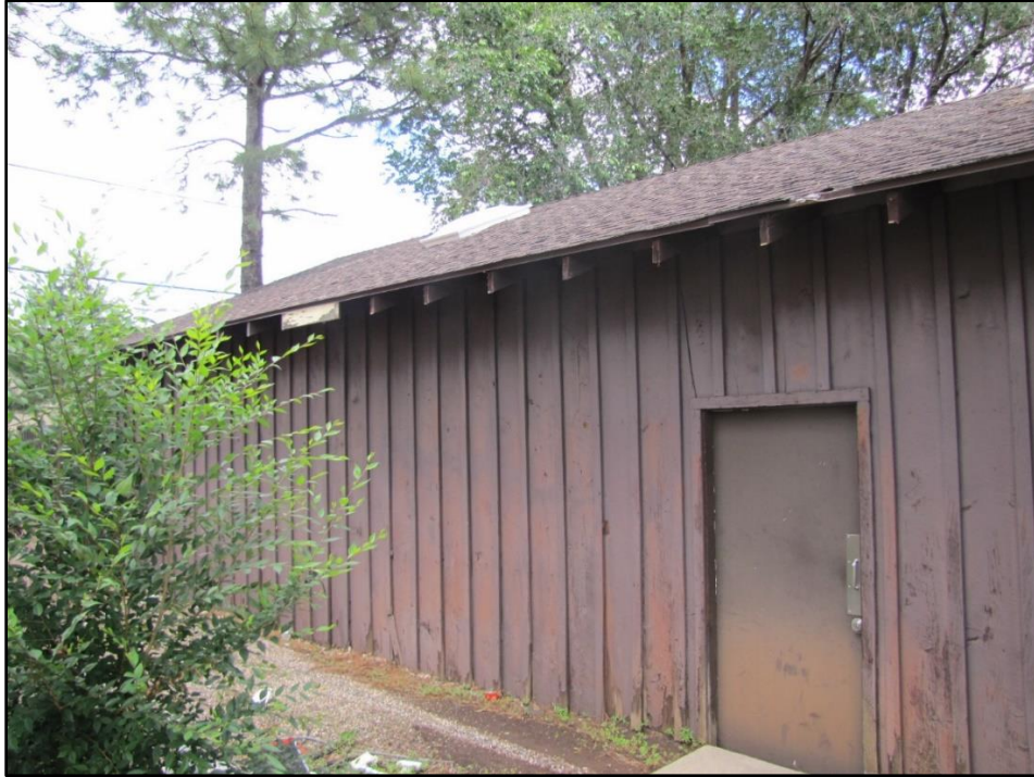
Photograph 30. West side of the Detached Garage, facing northeast.
