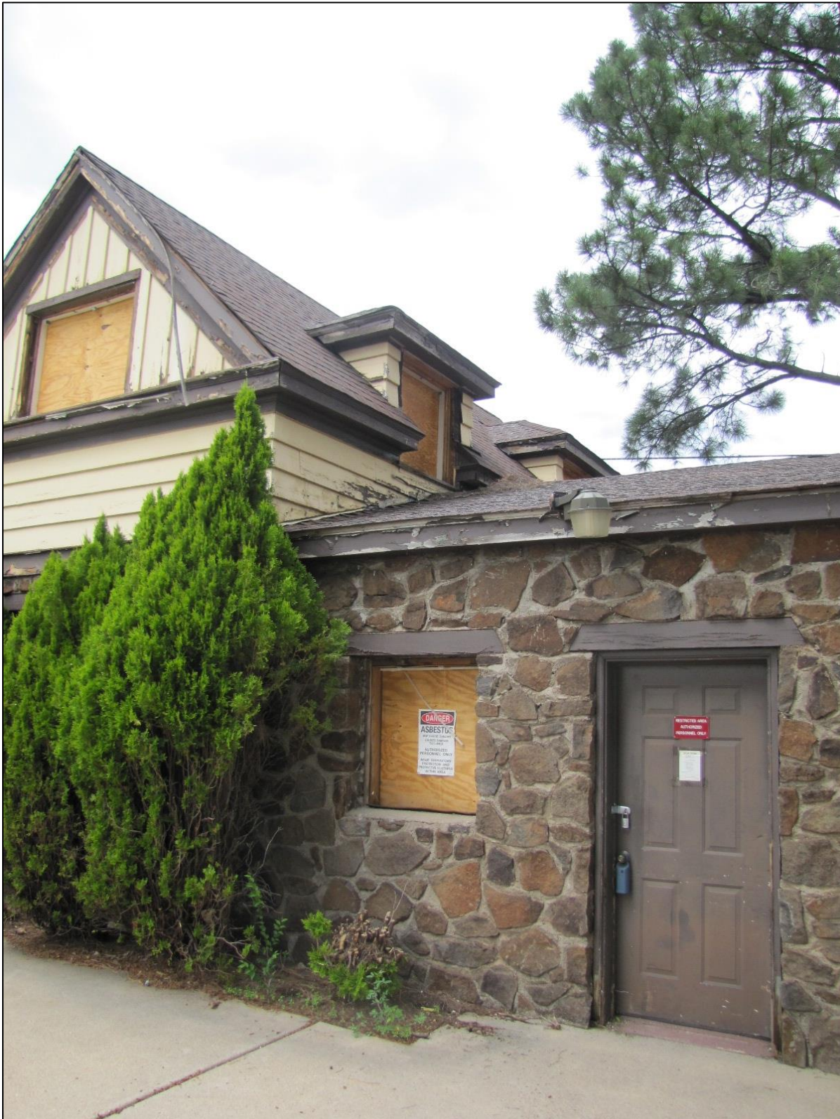
Photograph 23. Morgue Preparation Room and east second floor apartment, facing northwest.
