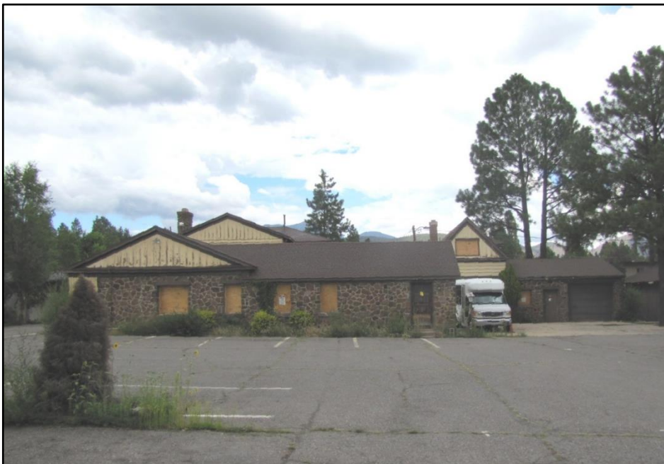
Photograph 8. Full façade of Chapel and Main Building, facing north.
