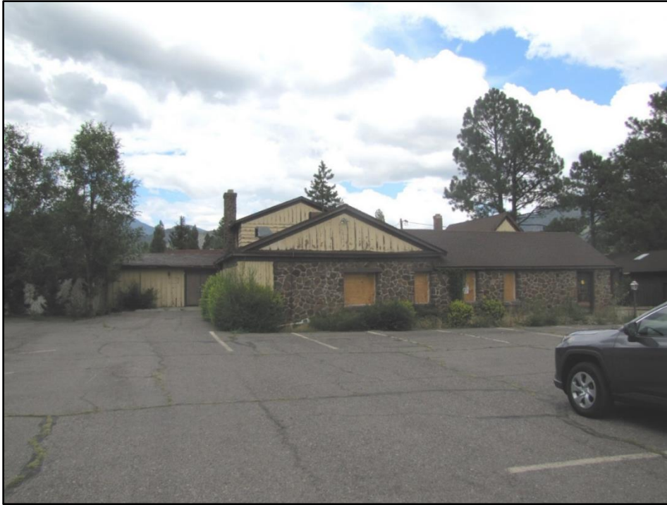
Photograph 7. Central and western façade of Chapel and Main Building, facing north.
