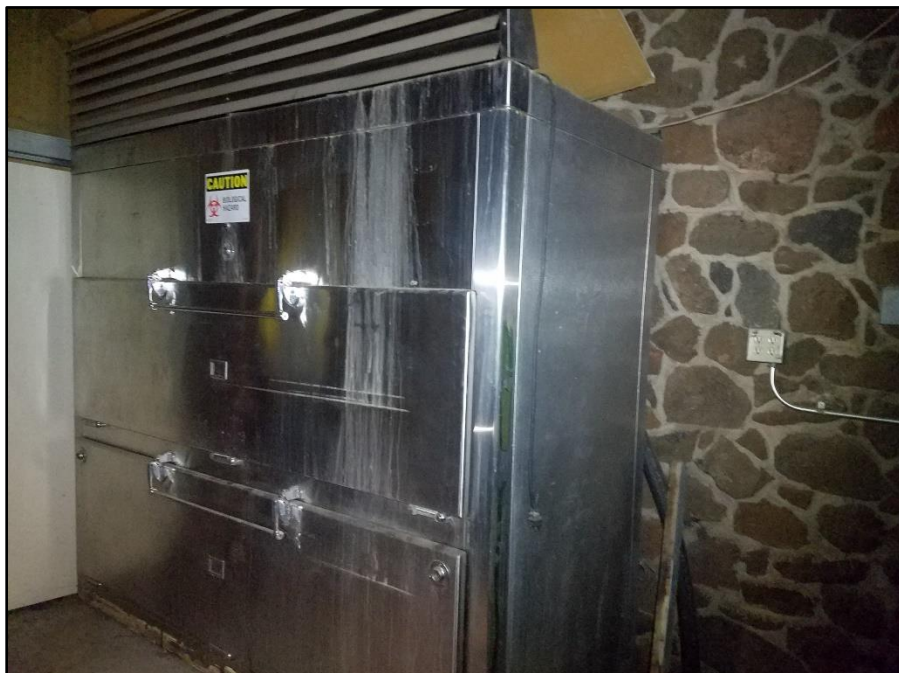
Photograph 4. Crematorium on 10/27/2021, facing south by southwest.
