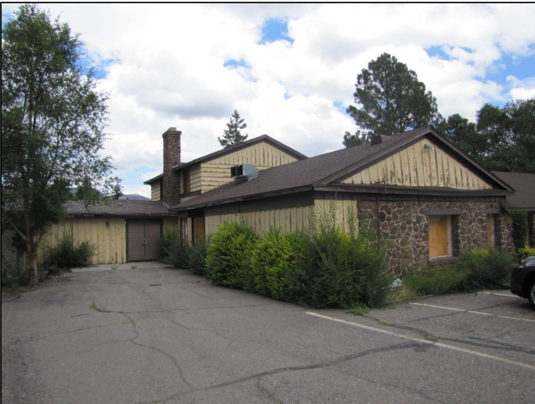
Photograph 27. Chapel, west side of Main Building and Northwest Addition, facing northeast.
