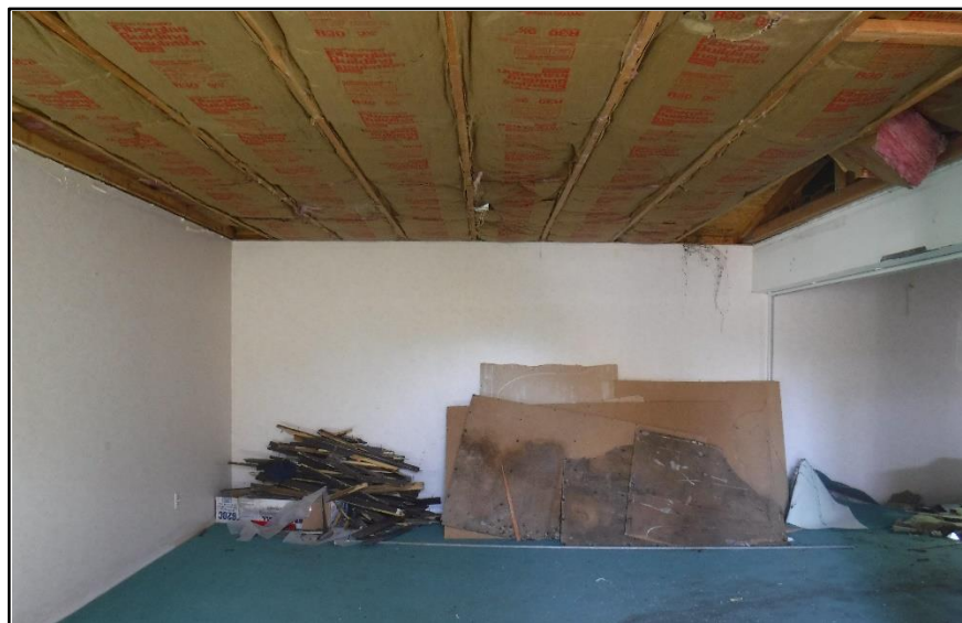
Photograph 5. Interior of casket display room addition on 10/27/2021, facing north.
