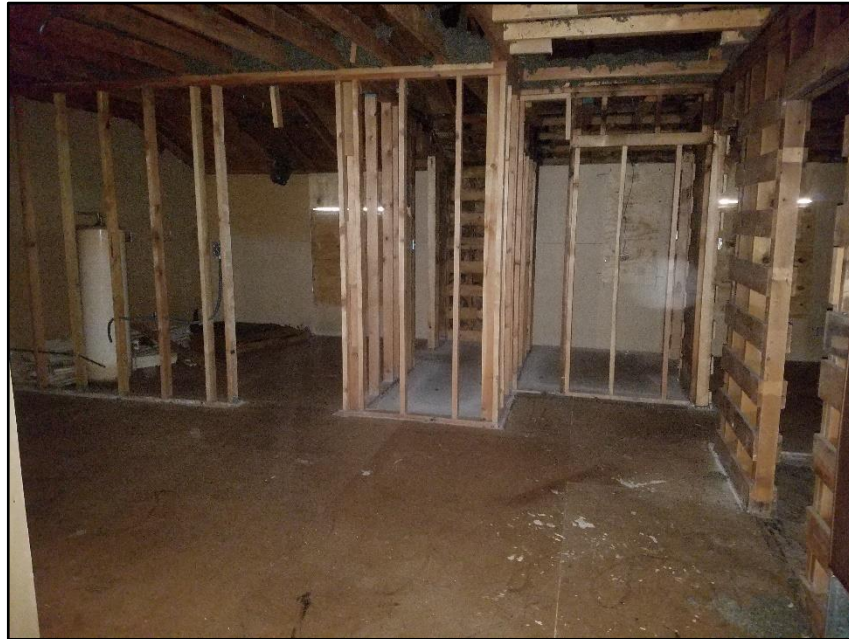
Photograph 24. Interior of second floor west apartment, facing southwest.
