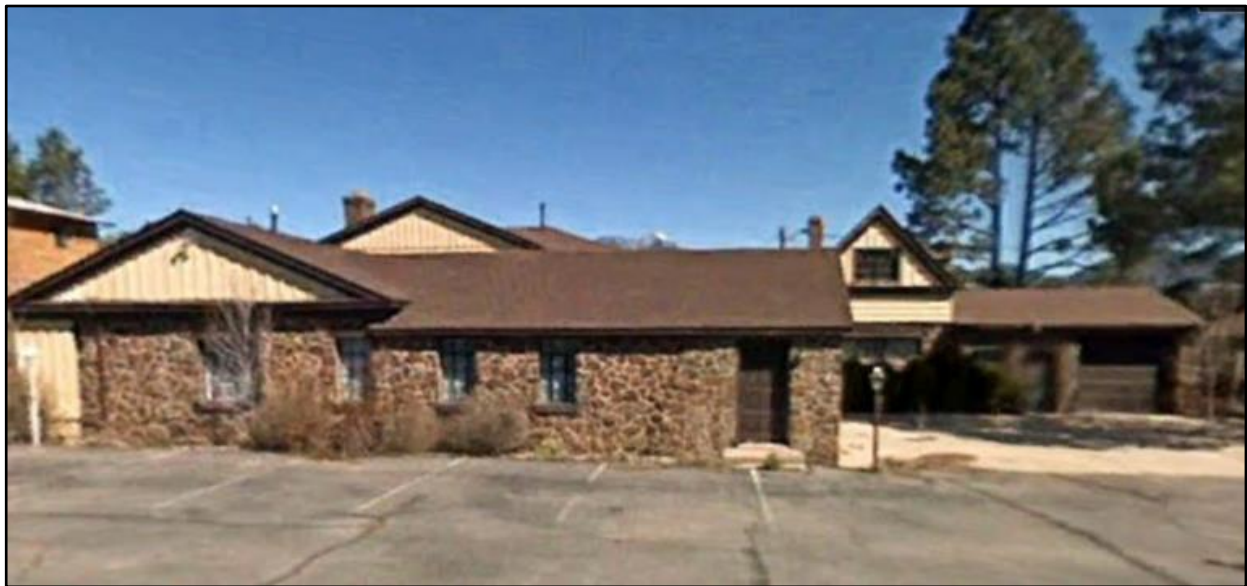
Photograph 10. Google Earth image off full façade of Chapel and Main Building, facing north.
