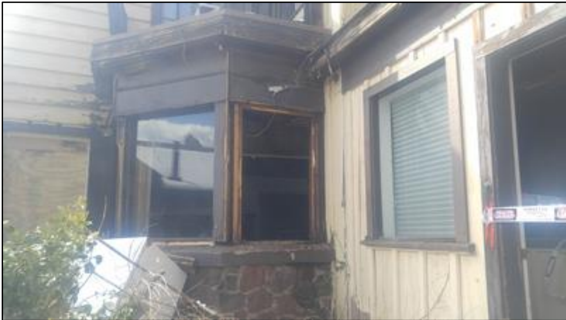
Photograph 36. Main Building and courtyard, facing northwest
