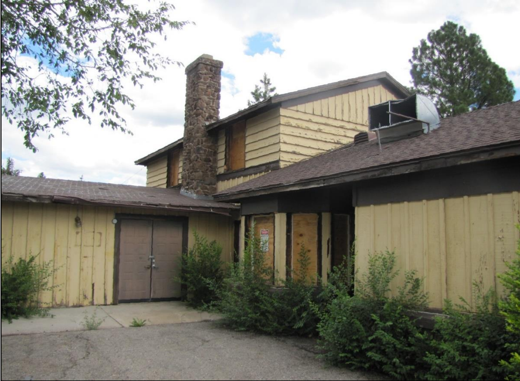
Photograph 26. West side of Main Building and Northwest Addition, facing northeast.
