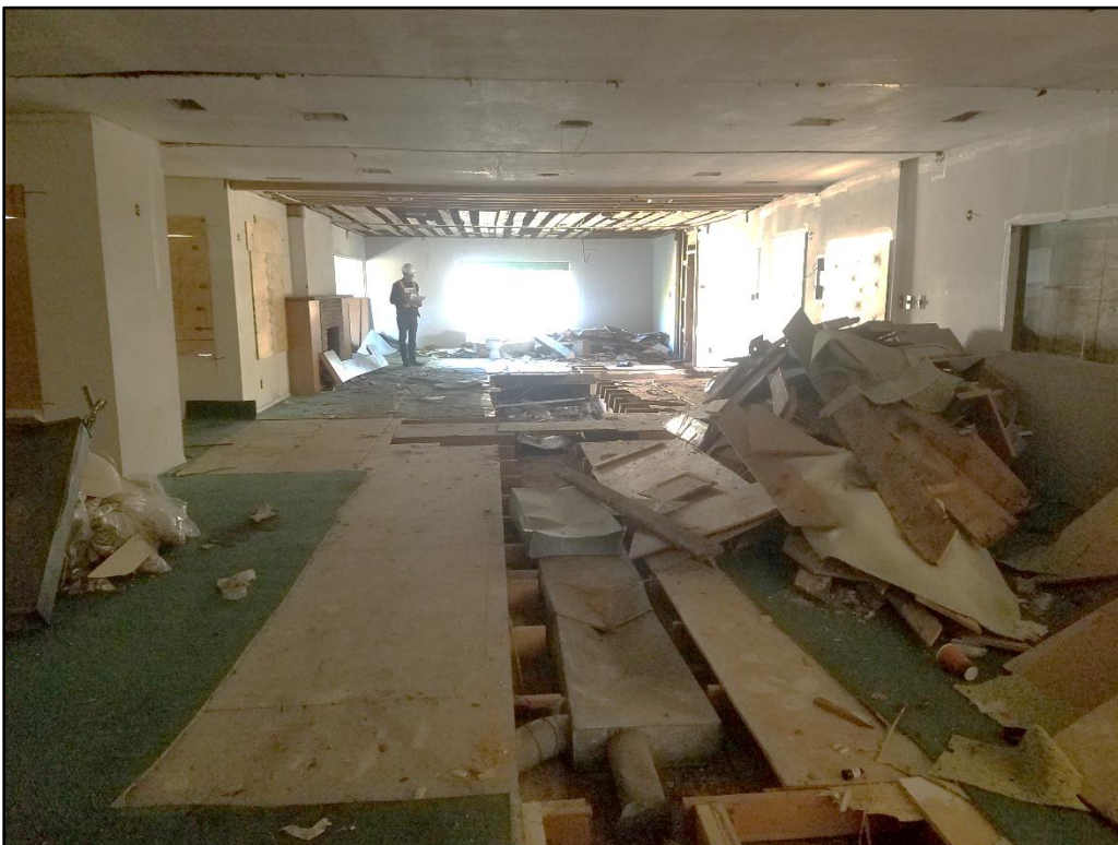
Photograph 2. Interior of viewing rooms on 10/27, facing south.
