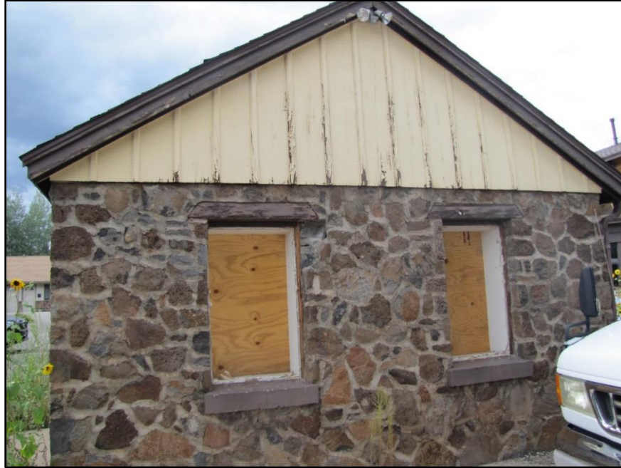
Photograph 15. East side of Chapel, facing west.
