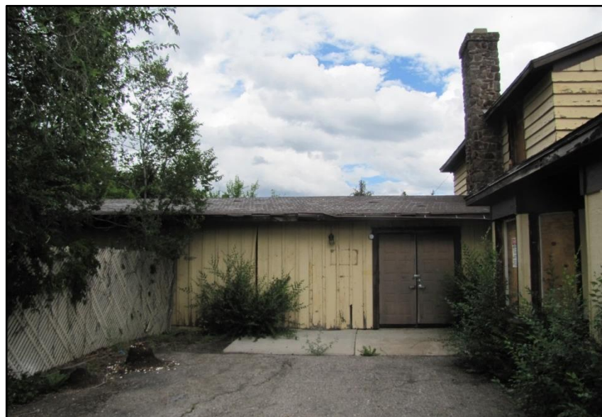
Photograph 25. Northwest Addition, facing north.
