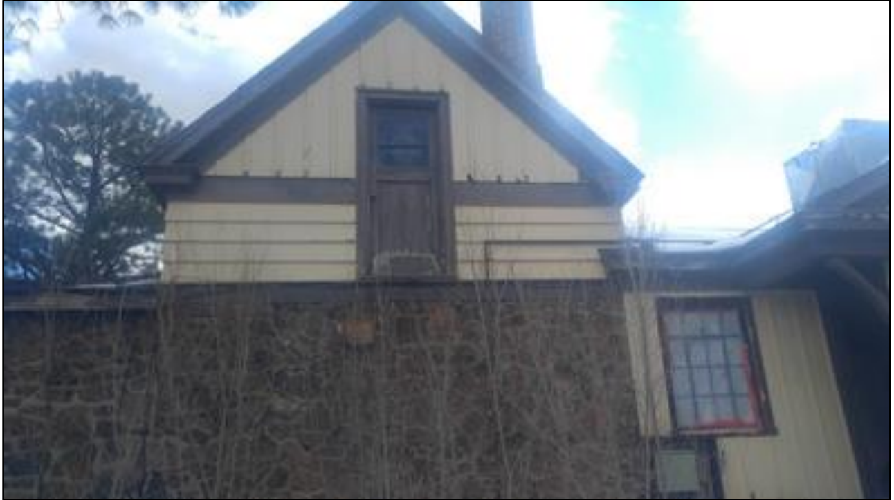
Photograph 34. Back of Main Building and east second-floor apartment, facing south.
