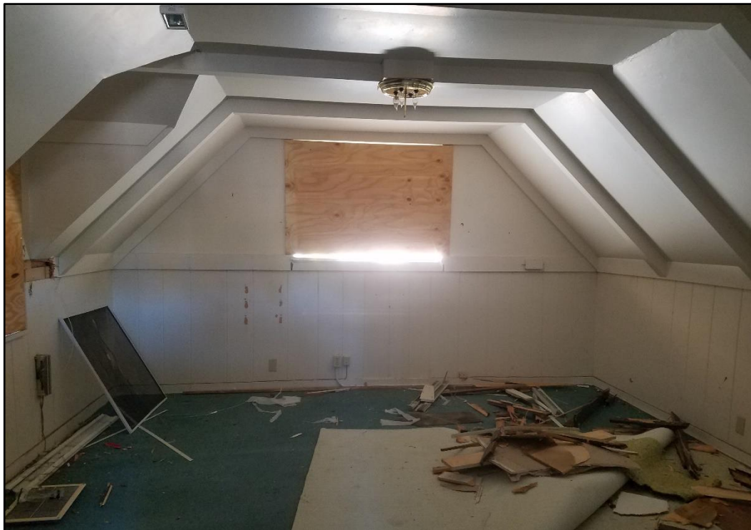
Photograph 22. Interior of second floor east apartment on 10/27/2021, facing south.
