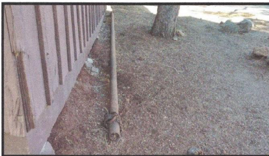
Photo# 9: Disconnected 3-inch gas line that was reportedly used to reach a 1,600-1,800 F temperature to fuel the crematorium. Viewing down, and to the west.
