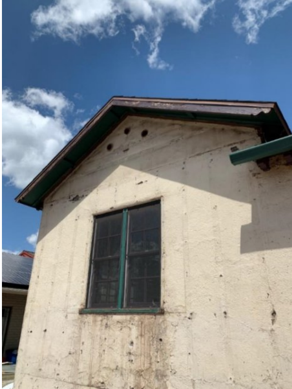
Stripped added stucco layer
