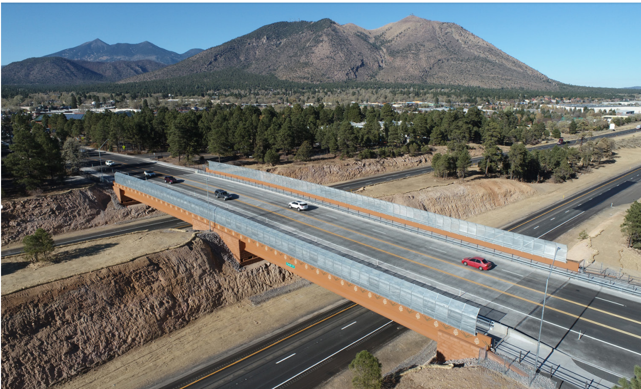
2020 Fourth Street Bridge After Completion: The project utilized an innovative bridge slide method that significantly reduced closures of Fourth St from 3-4 months with traditional methods to 17 days.
