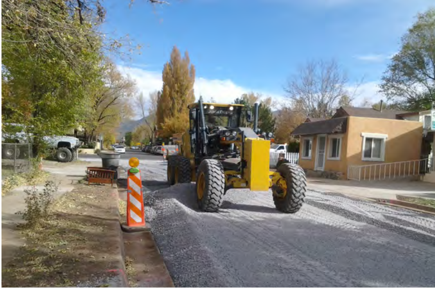
Photo credit: City of Flagstaff
