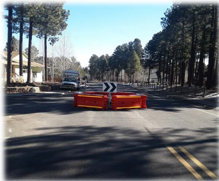
Eastbound View of the Temporary Traffic Circle
