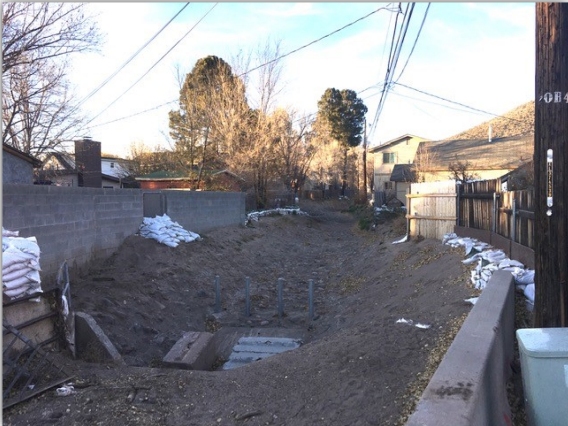
Spruce Wash north of Dortha Avenue
