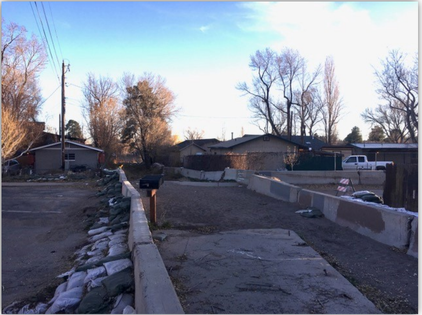
Spruce Wash – looking south at Dortha Avenue
