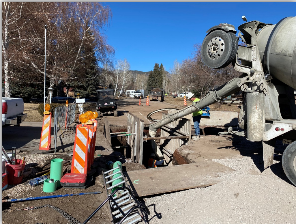
Navajo Dr. at Whiting Rd., looking north the sewer main installations.
