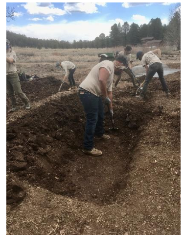
ACE crew digging beds
