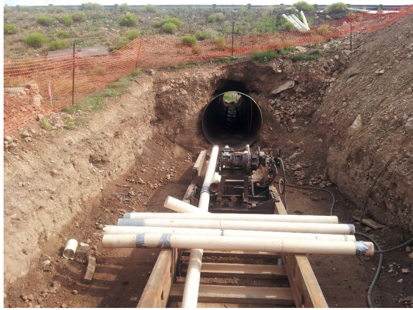
2013: E. Route 66 culvert replacement
