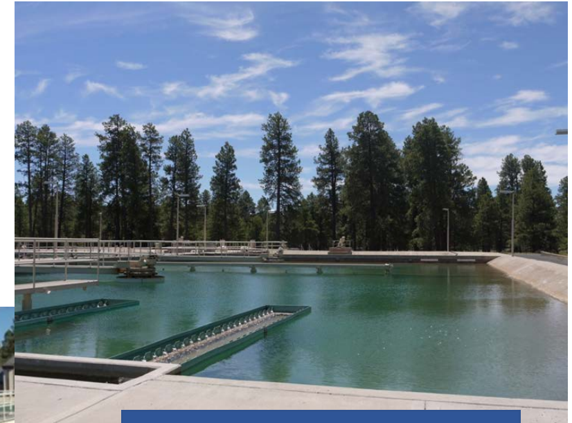
Lake Mary WTP Basins
