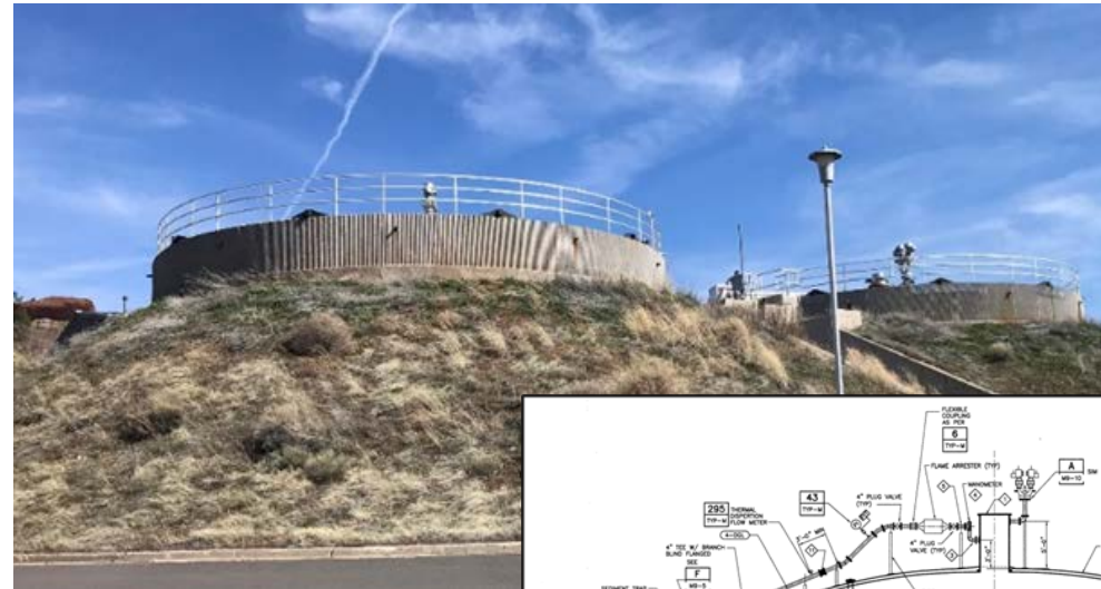
Existing Anaerobic Digesters at WHWRP
