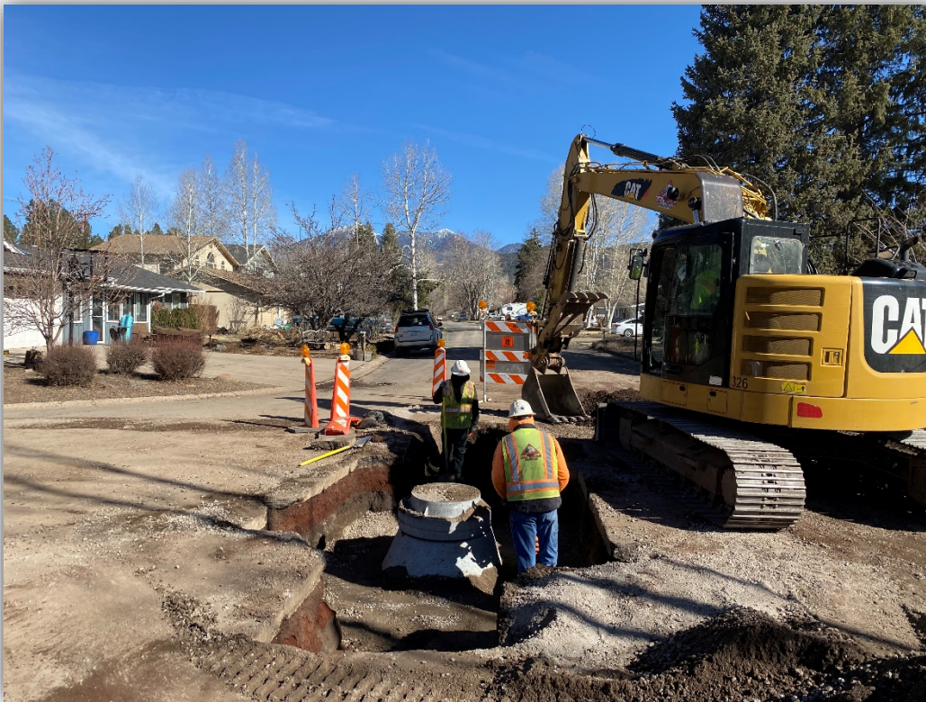
Navajo Dr. at Anderson Dr., looking north the sewer main installations.
