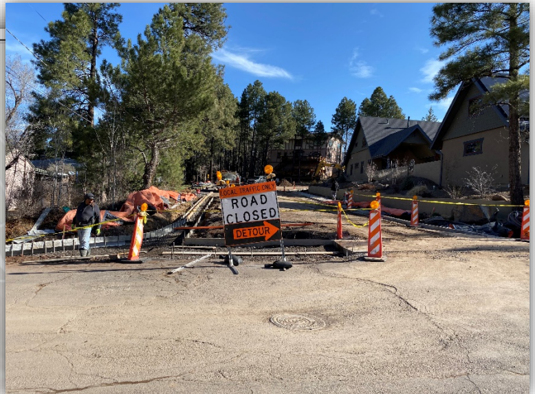
Hutcheson/Fine, looking north at Hutcheson concrete work.
