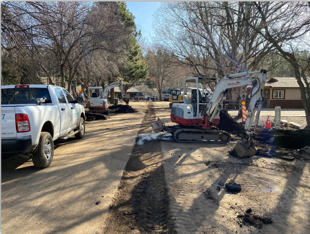
Hazel/Talkington intersection, looking east at sewer installations.
