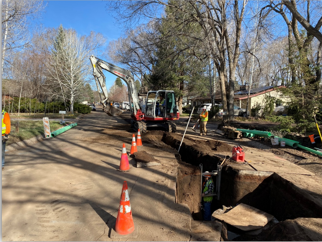
Talkington north of Davis, looking north at sewer installations.
