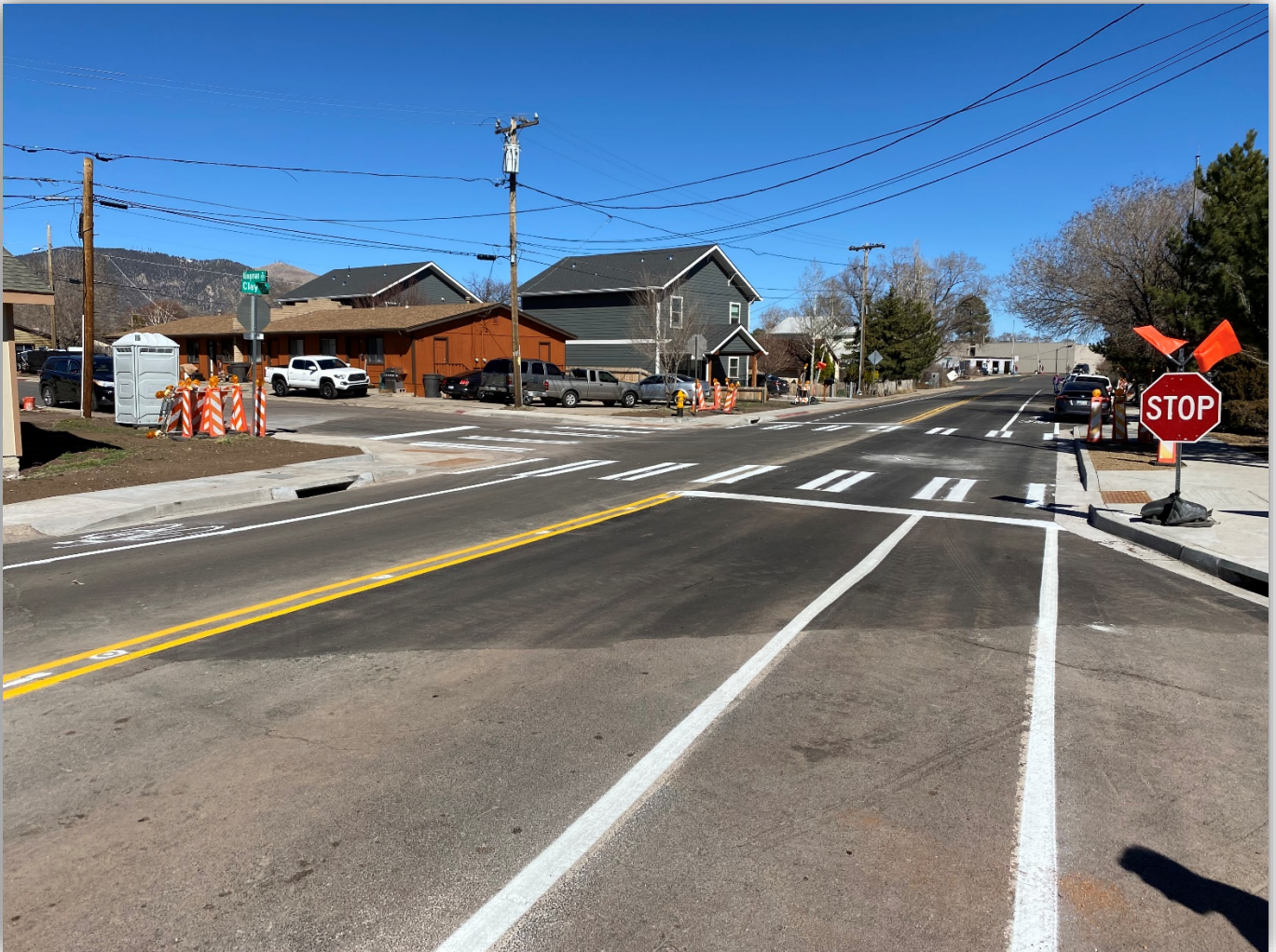
Kingman/Clay intersection looking east at final pavement markings.
