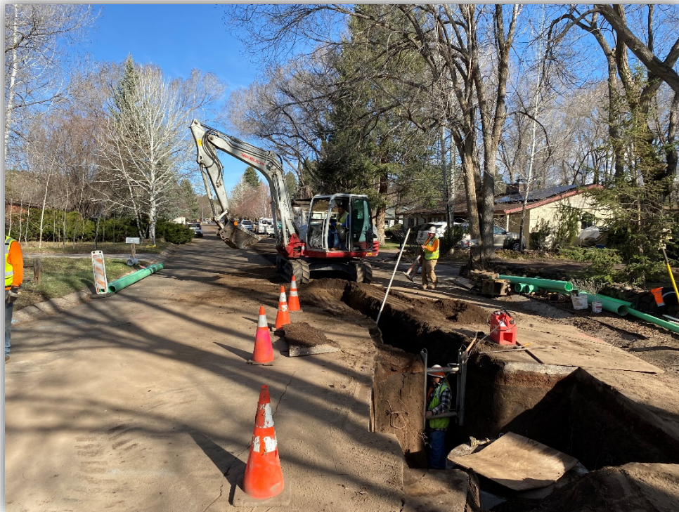
Hazel/Talkington intersection, looking east at sewer installations.
