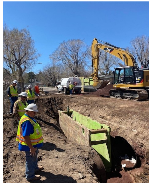
Utility relocation trenching and shoring in Dortha Avenue
