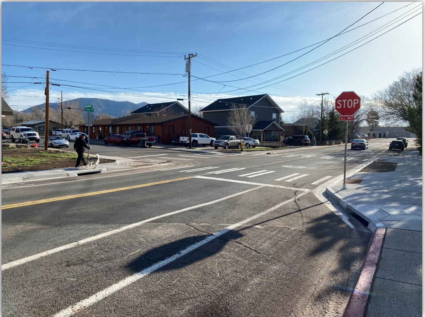
Kingman/Clay intersection looking east at completed improvements.
