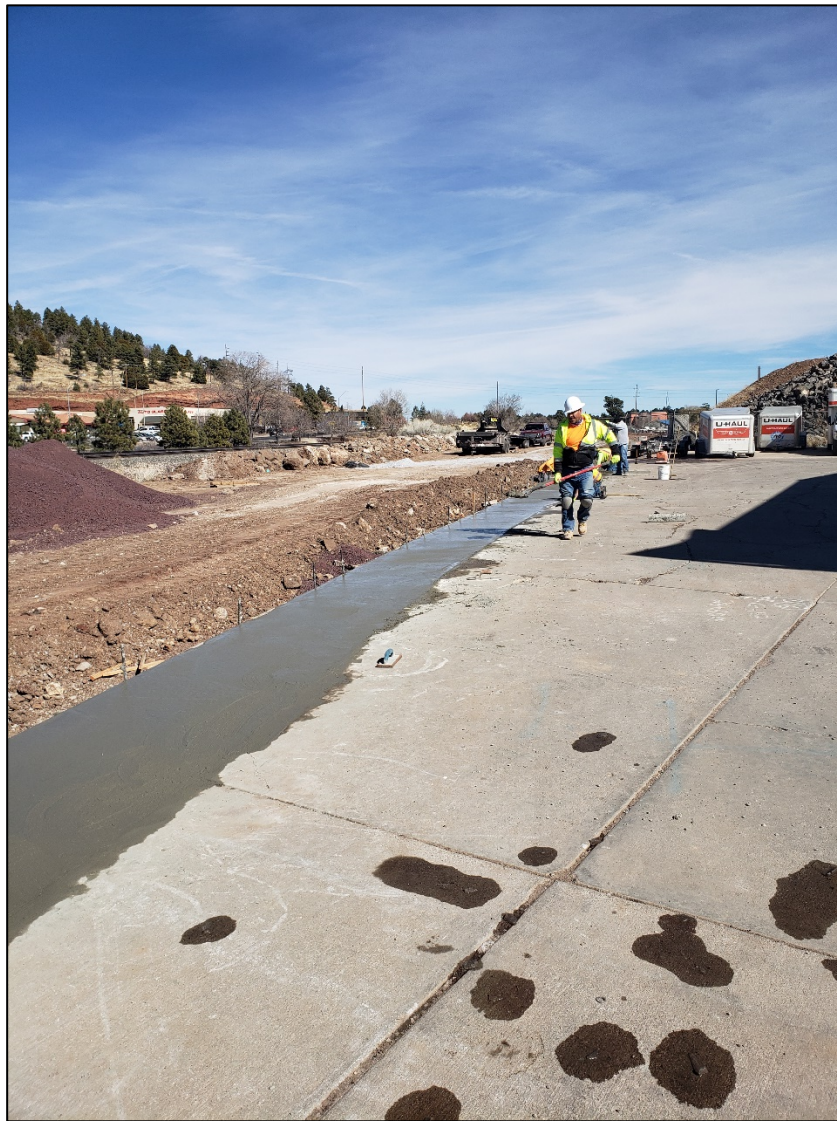
Huntington Waterline Replacement, crews working to finish concrete work at U-Haul related to the waterline replacement
