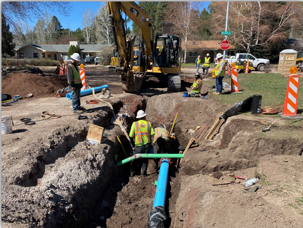
Navajo Dr. at Murray Rd., looking at water and sewer installations.
