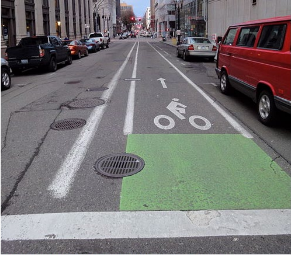
A buffered bicycle lane on downtown Portland's Southwest Stark Street
