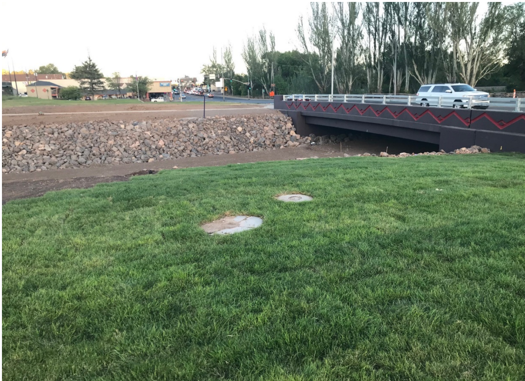
Upstream channel protection and turf replacement
