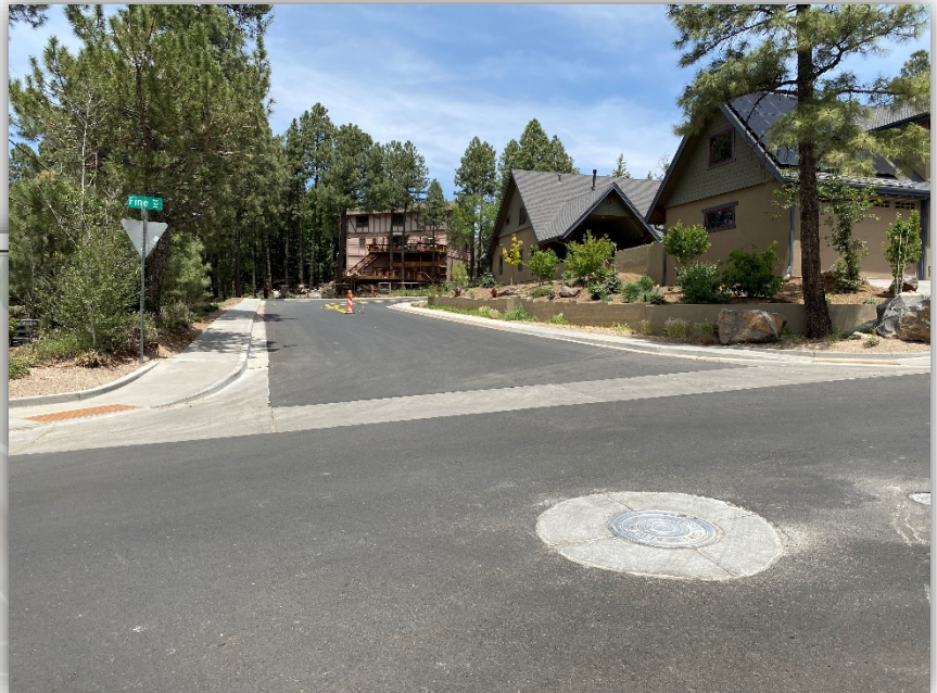
Fine, looking north at final striping on Hutcheson.
