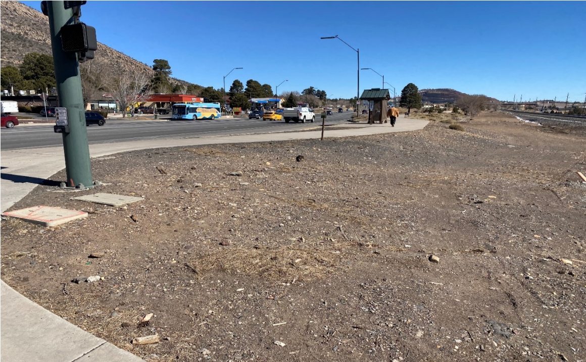
Rte. 66 At Fanning Landscaping-Existing Conditions
