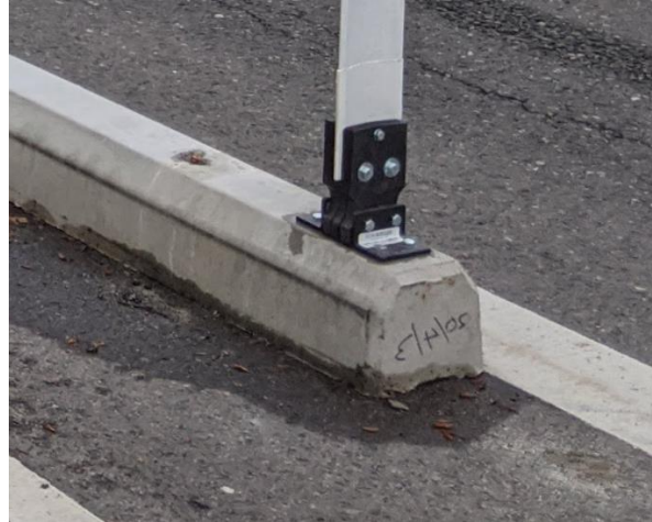
Figure 9: Delineator Hardware - Final Solution
