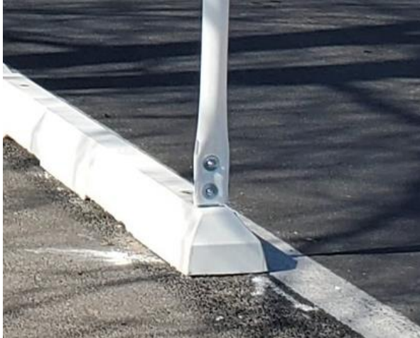
Figure 8: Delineator Hardware - First Attempt
