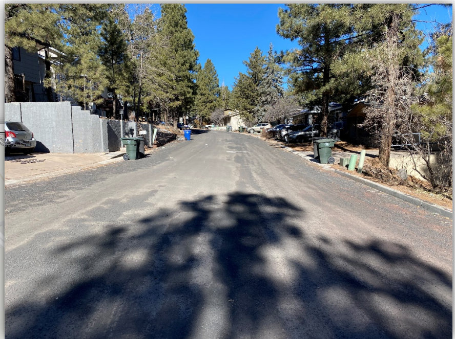
Canyon Terrace Dr, looking north at the completed project.
