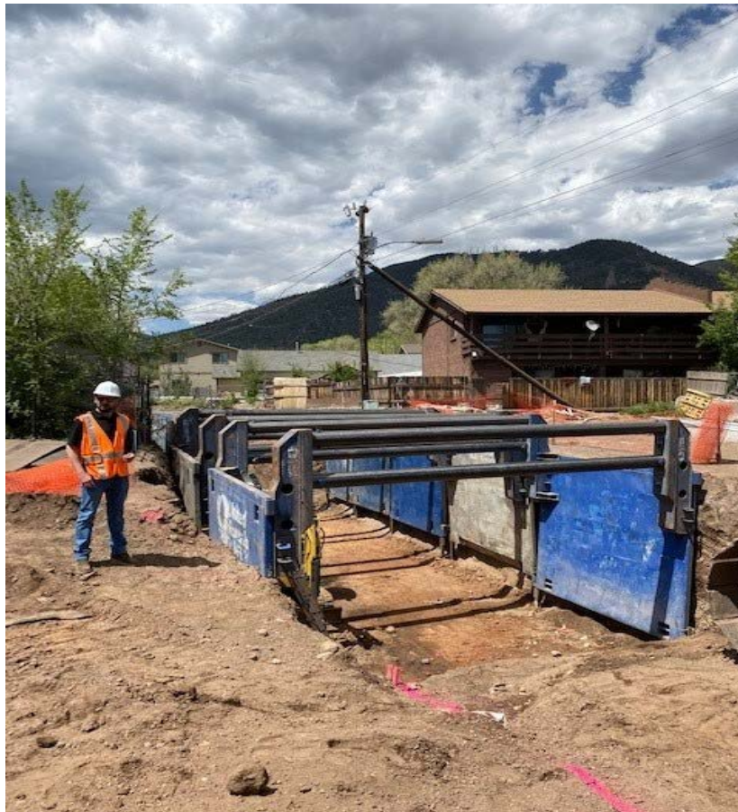
Shoring installation - looking north
