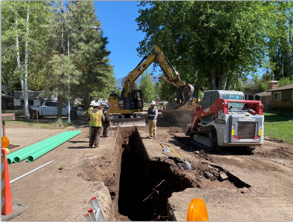
Navajo Dr. at Whiting Rd., looking north at the concrete curb and gutter installations.
