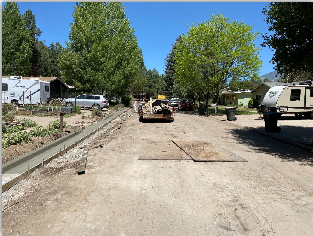
Crescent south of Venus intersection, looking north at concrete curb installations.
