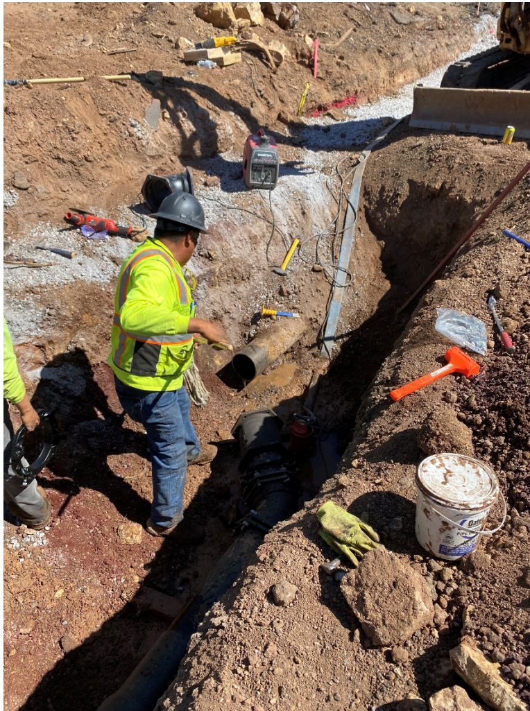
El Paso Flagstaff Rd, crews connecting the new 8” waterline to existing
