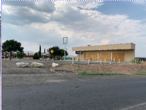
Site #2. Former Circle K (Camp Verde)
