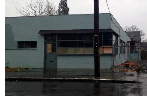
Vacant Commercial Building
