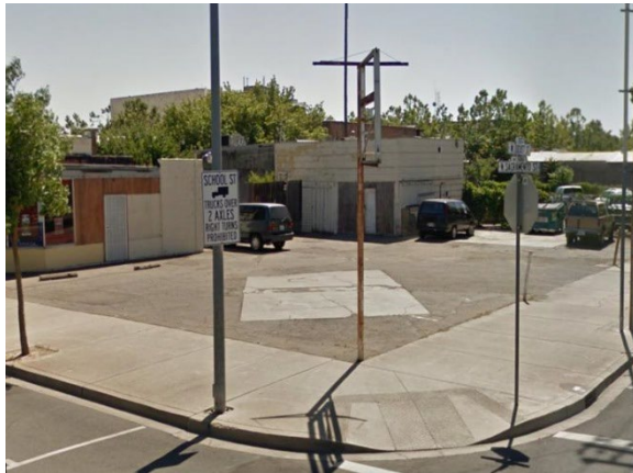
Former Gas Station
