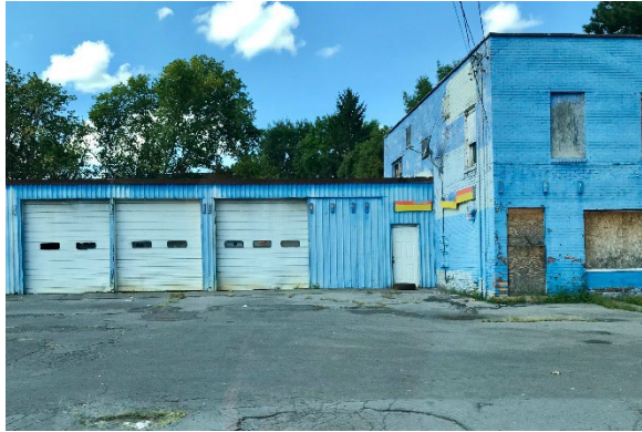
Former Auto Repair Shop
