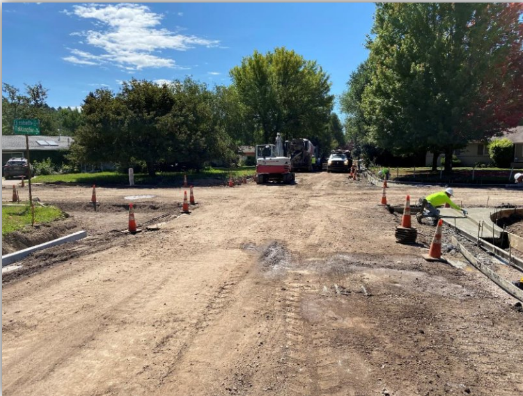
Talkington/Elizabeth intersection, looking south at concrete curb installations
