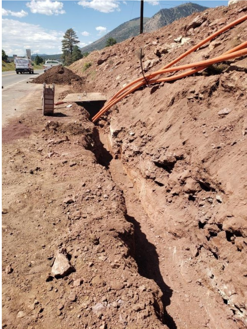
E. Rt. 66, Installation of fiber conduit bank for IT's Fiber Masterplan
