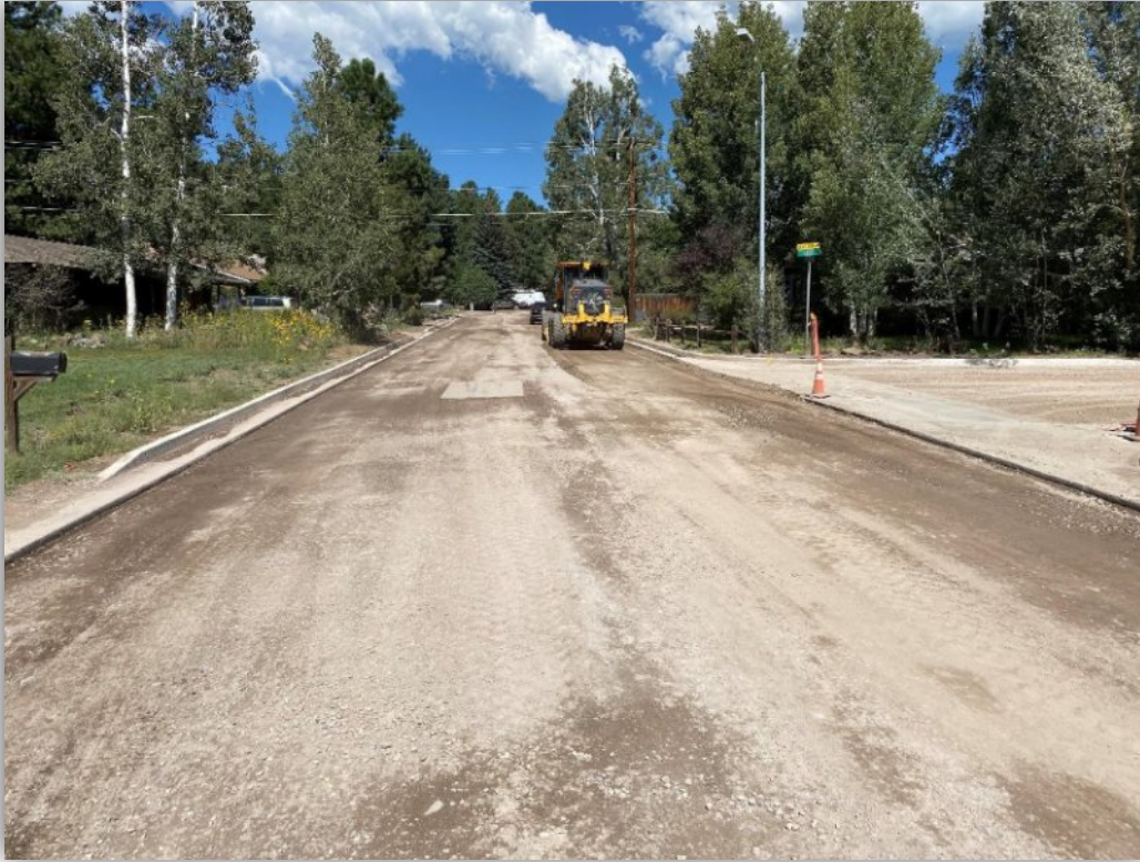
Crescent/Azure intersection, looking north at final roadway grading prior to roadway paving on September 7-9
