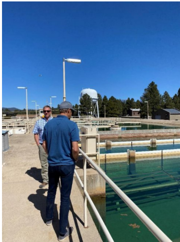
Staff and Brown and Caldwell taking a tour of the LMWTP basins
