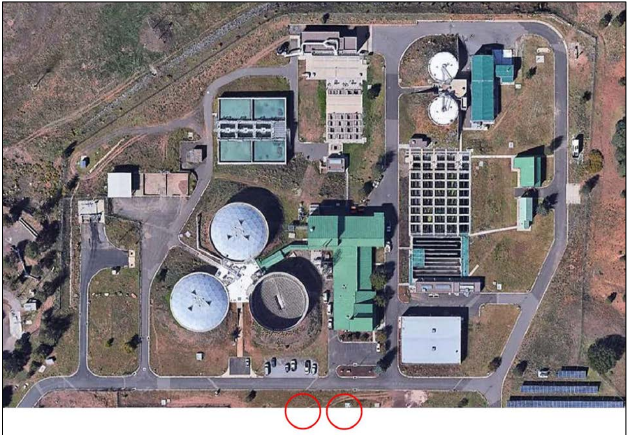
Existing Wildcat Plant, red circles represent possible locations of the new digester
