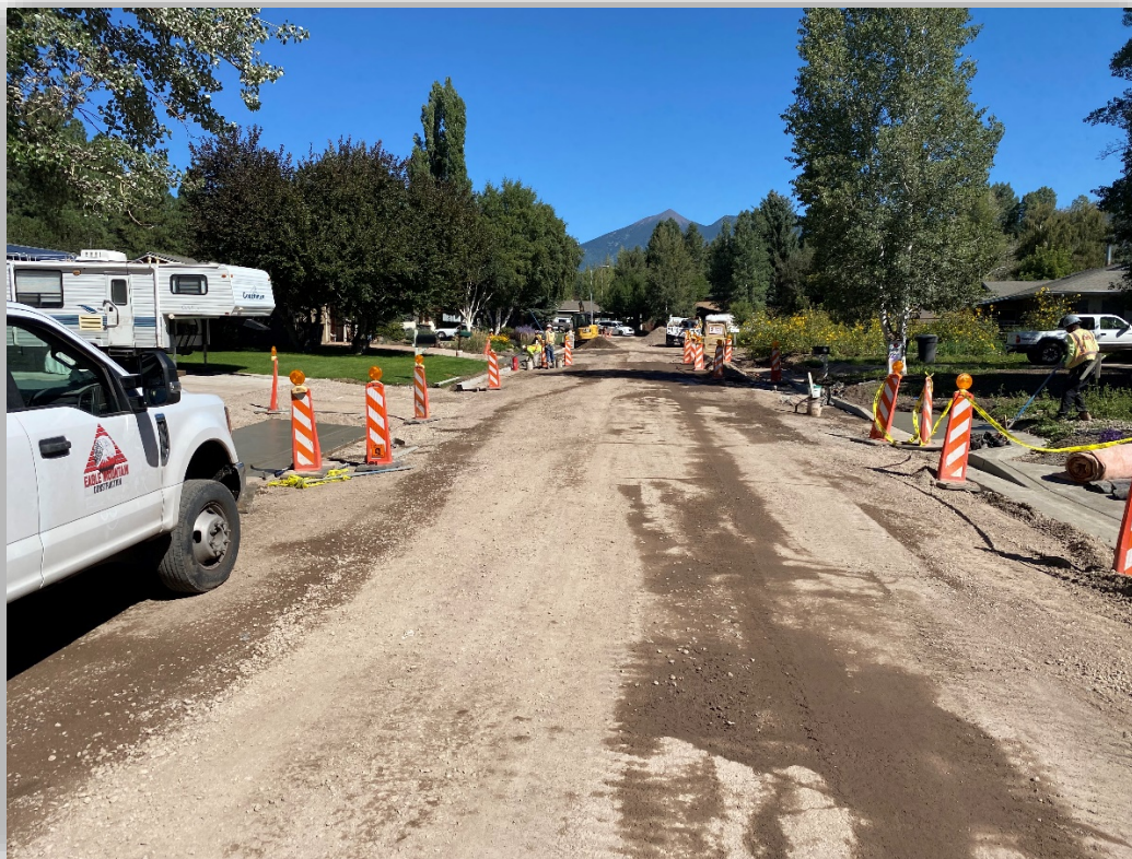
N Navajo Dr. at Murray Rd., looking north at completed curb installations up to Murray.
