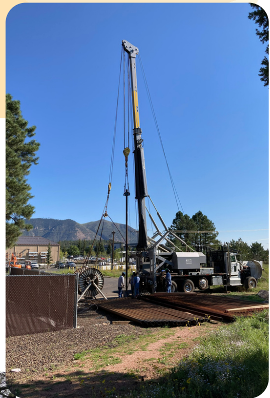
Re-equipping Rio Well
