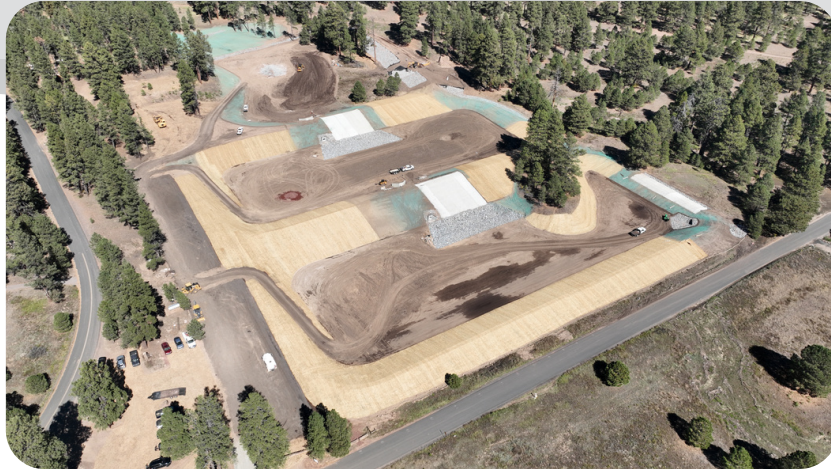
Schultz Creek Flood and Sediment Detention Basins
