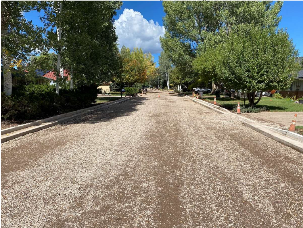
Navajo, looking north at roadway prepared for roadway asphalt paving
