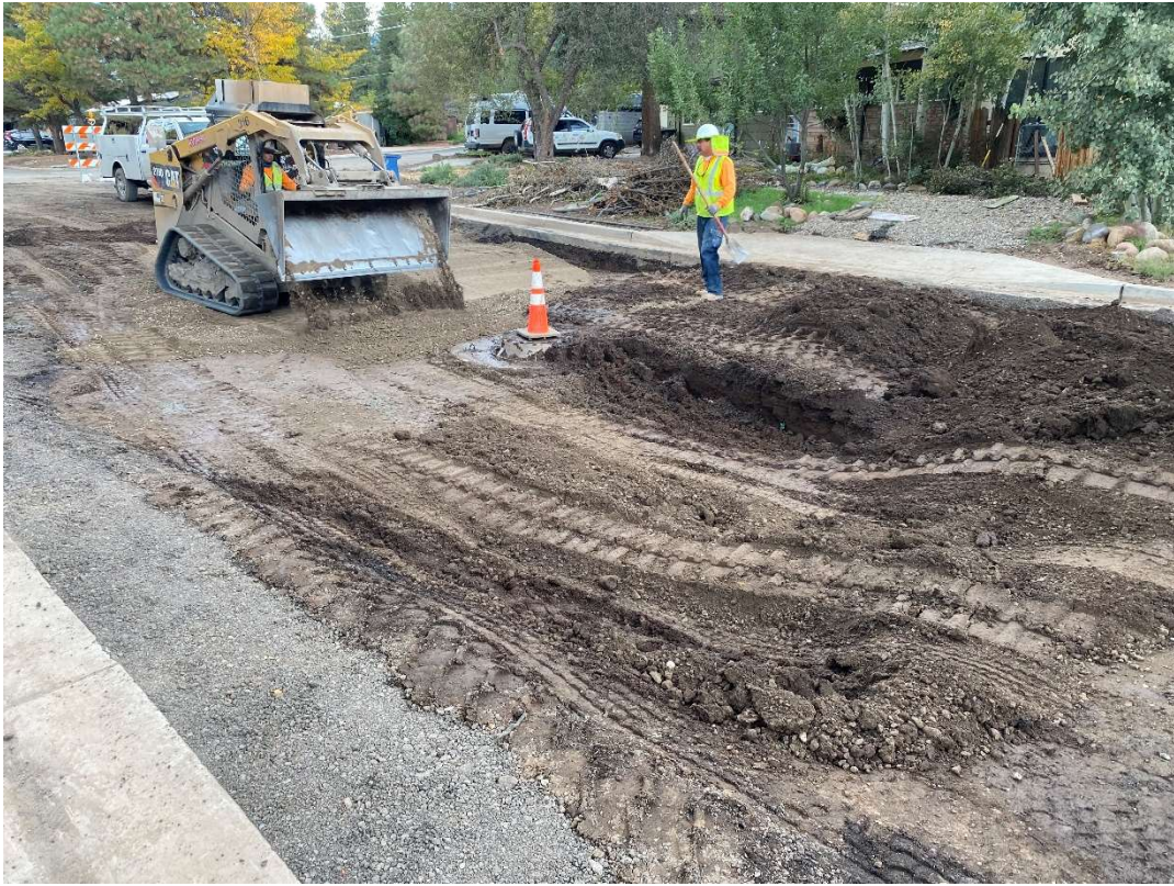
Talkington/Louise intersection, looking north at subgrade stabilization
