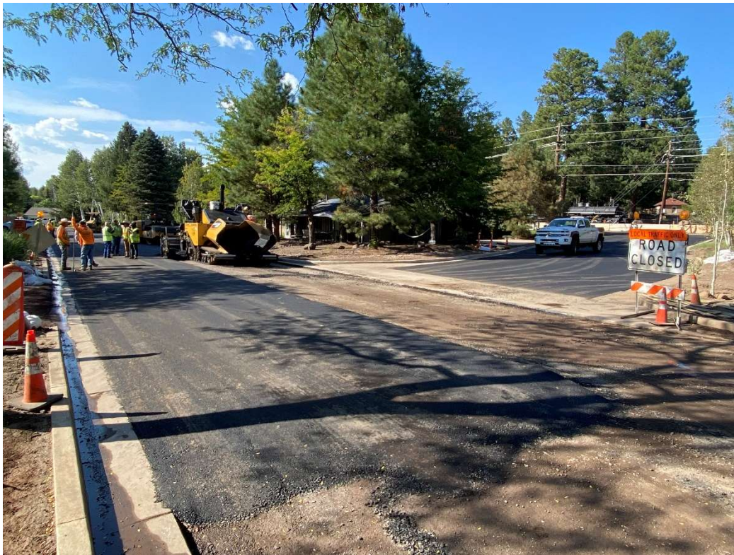
Talkington/Louise intersection, looking north at roadway asphalt paving
