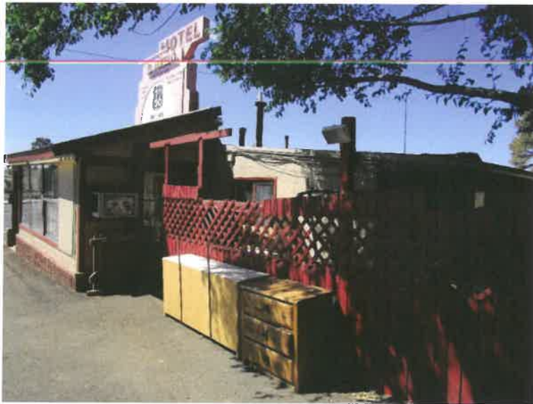
Additions to the office Building
