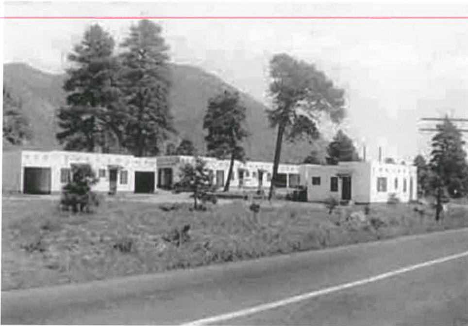
1940 Photograph (Cline Library) with Added Room
