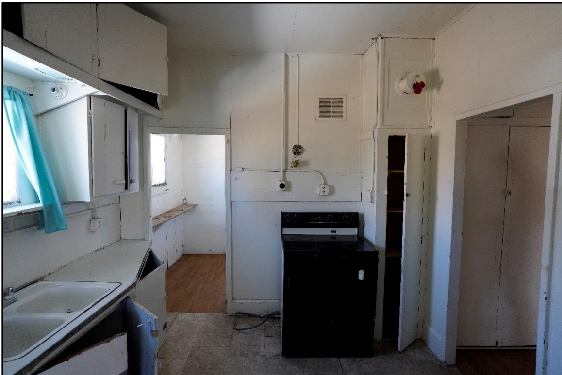
Appendix A- 10. Photograph of kitchen, facing east.
