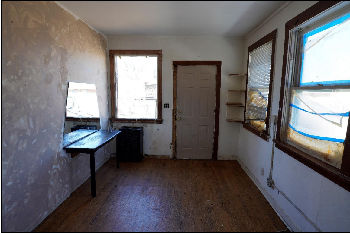
Appendix A- 7. Photograph of bedroom 2, facing west.
