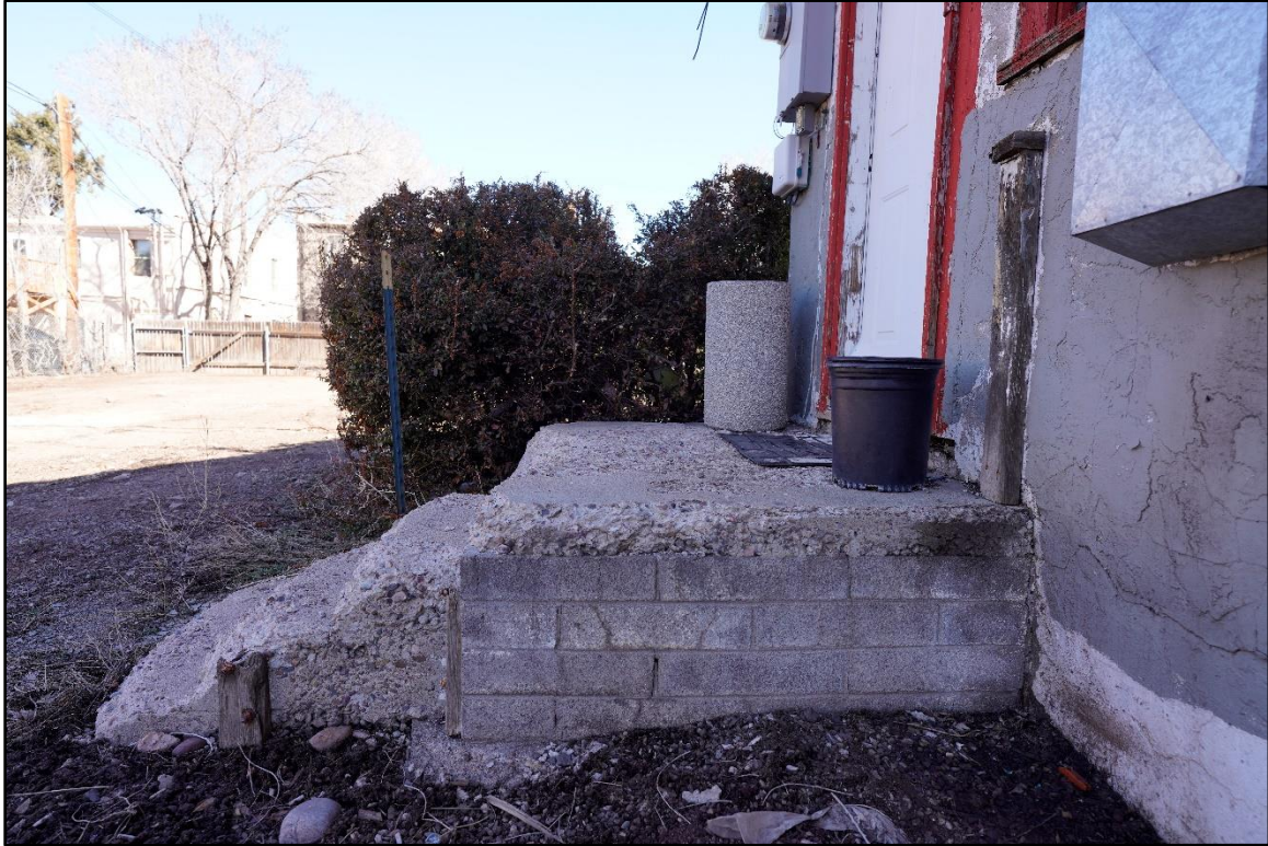
Appendix A- 13. Photograph of back stoop, facing north.
