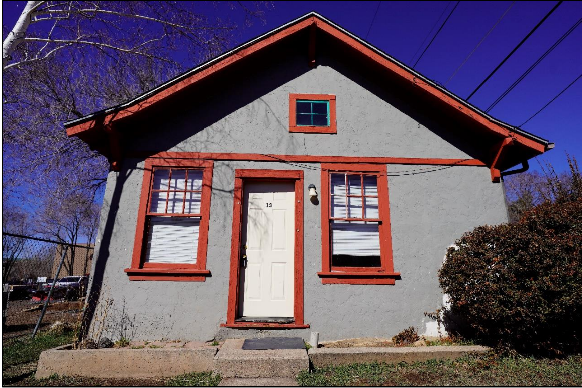
Photograph 17. Overview photograph of east elevation, facing west.
