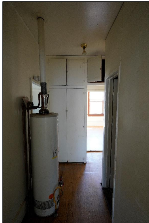
Appendix A- 8. Photograph of laundry/hall, facing east.
