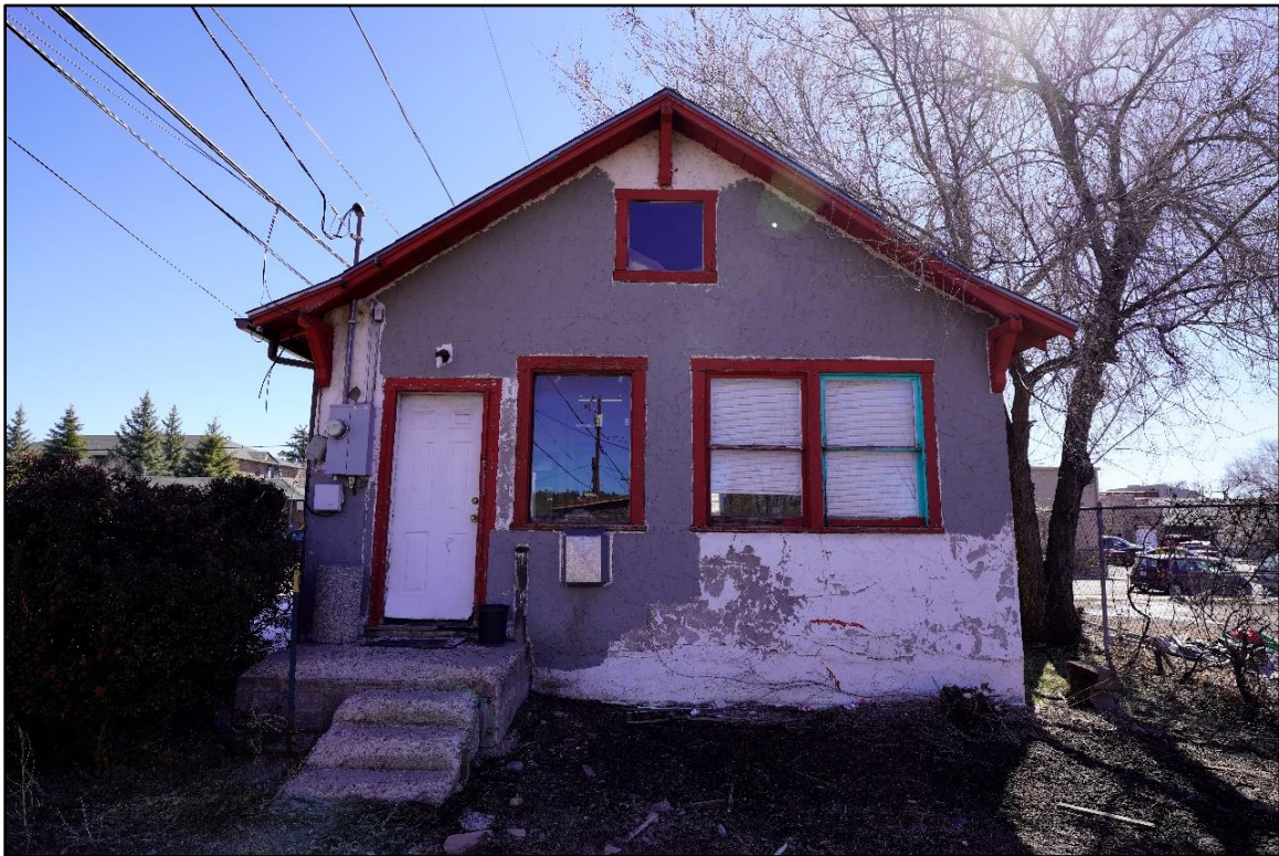
Photograph 18. Overview of west elevation, facing east.
