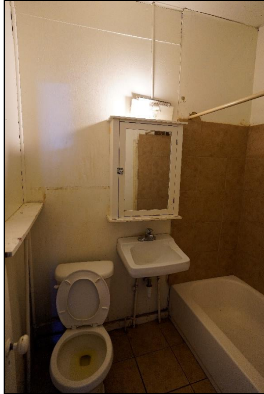
Appendix A- 9. Photograph of bathroom, facing southwest.
