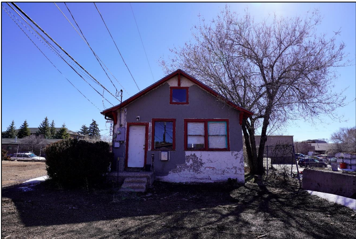
Appendix A- 4 Overview of MHCH, facing west
