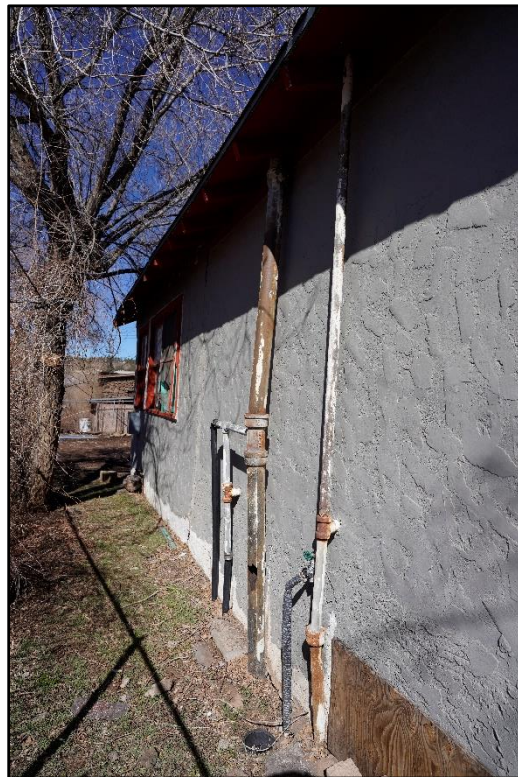
Appendix A- 14. Photograph of south elevation, facing northwest.
