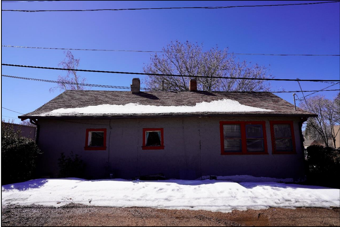
Photograph 19. Overview of north elevation, facing south.
