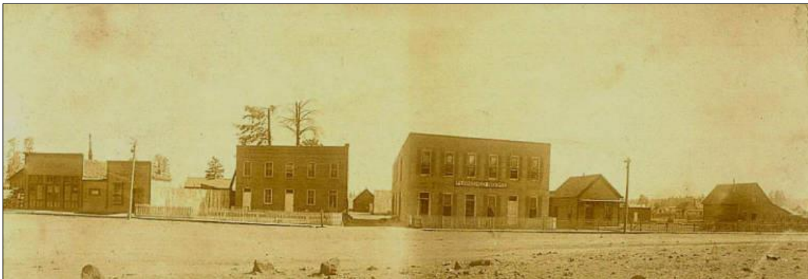
Photograph 12. 1910 Photograph of Hicks Boarding House (second from left), and St. Anne’s Apartments (right of Hicks Boarding House). Photo courtesy of Cline Library Special Collections, NAU.PH.91.7.254.
