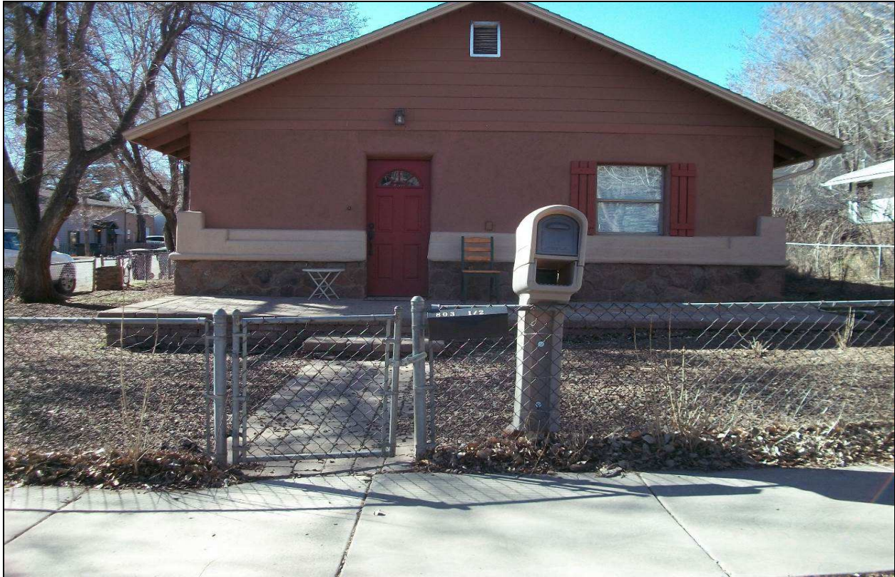
Figure 1. Main/north entrance of structure facing south.
