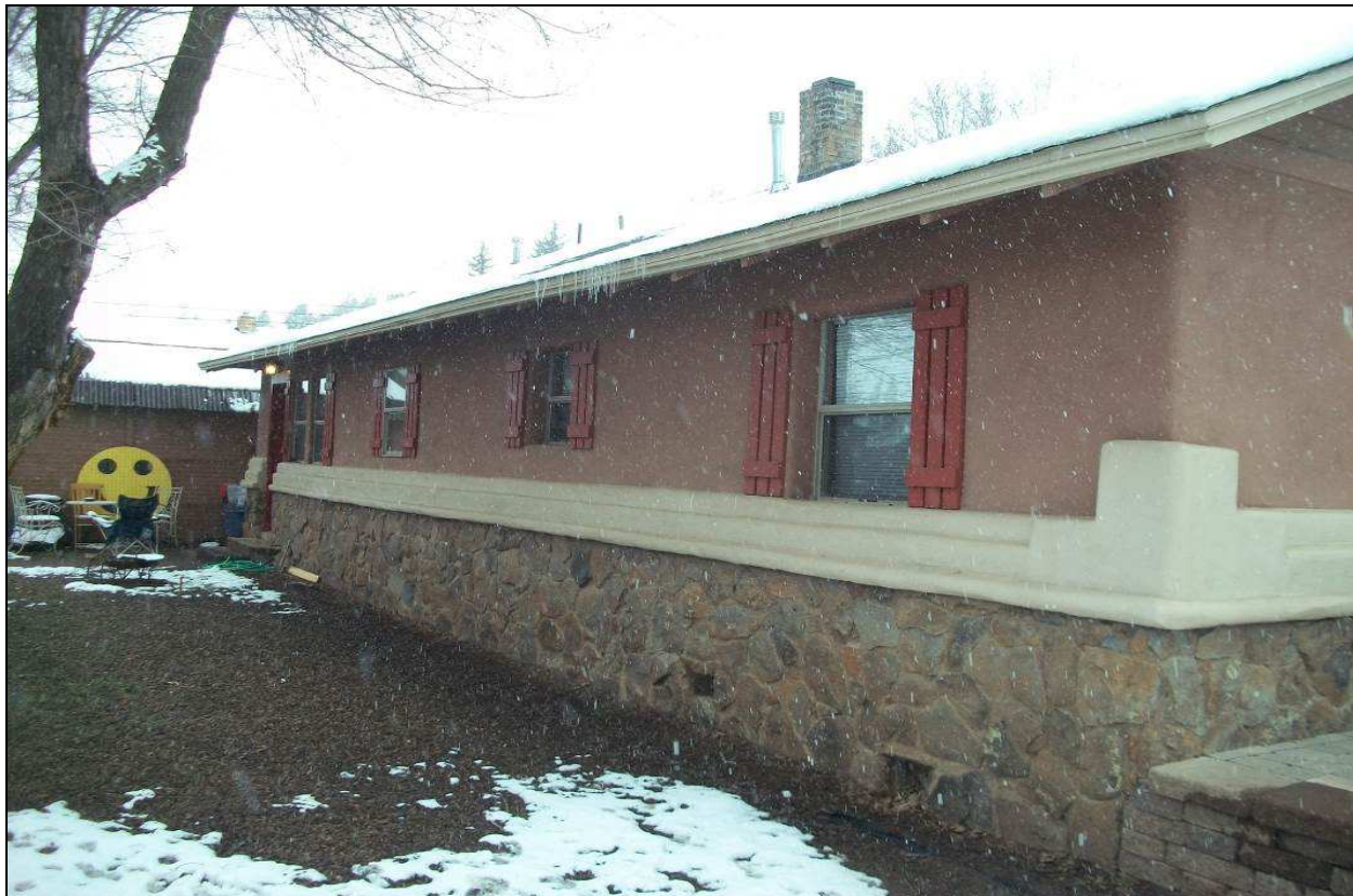
Figure 3. East side of structure showing roof eaves and rafters, facing southwest.
