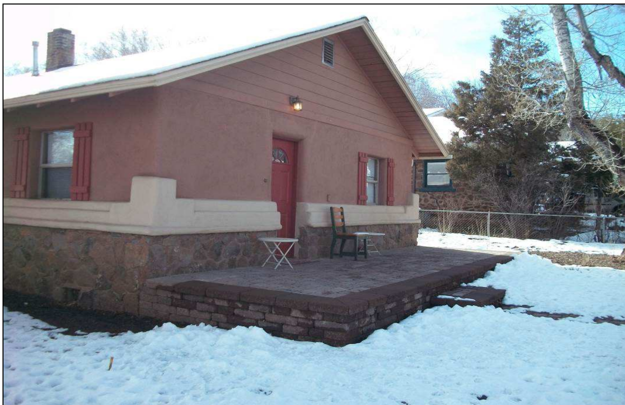
Figure 4. Main/north entrance showing significant exterior modifications including modern porch, facing southwest.
