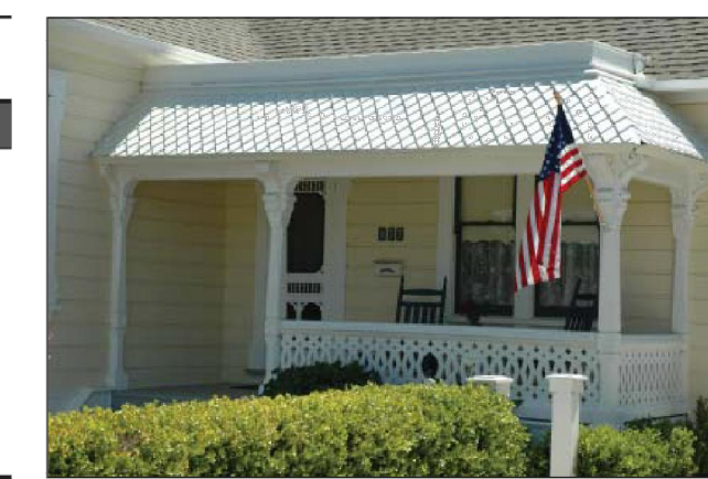
Engaged porch as an attached element.
