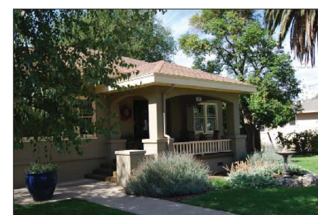
Partial-length projecting porch with stairs parallel to street.
