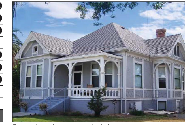
Engaged porch as an attached element.
