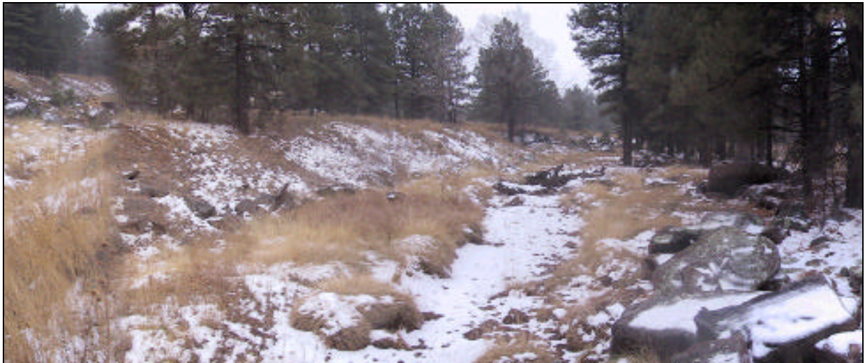
Figure A12. Bridge site #4 at Area “K”. Photo taken looking downstream.
