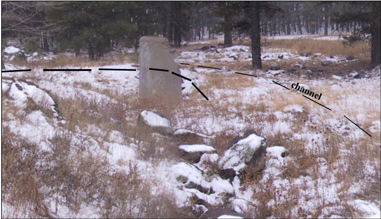
Figure A8. Existing manhole lies exposed in floodplain. Left terrace will be extended to include manhole to improve aesthetics and reduce floodplain scour. Area “N” on site map.
