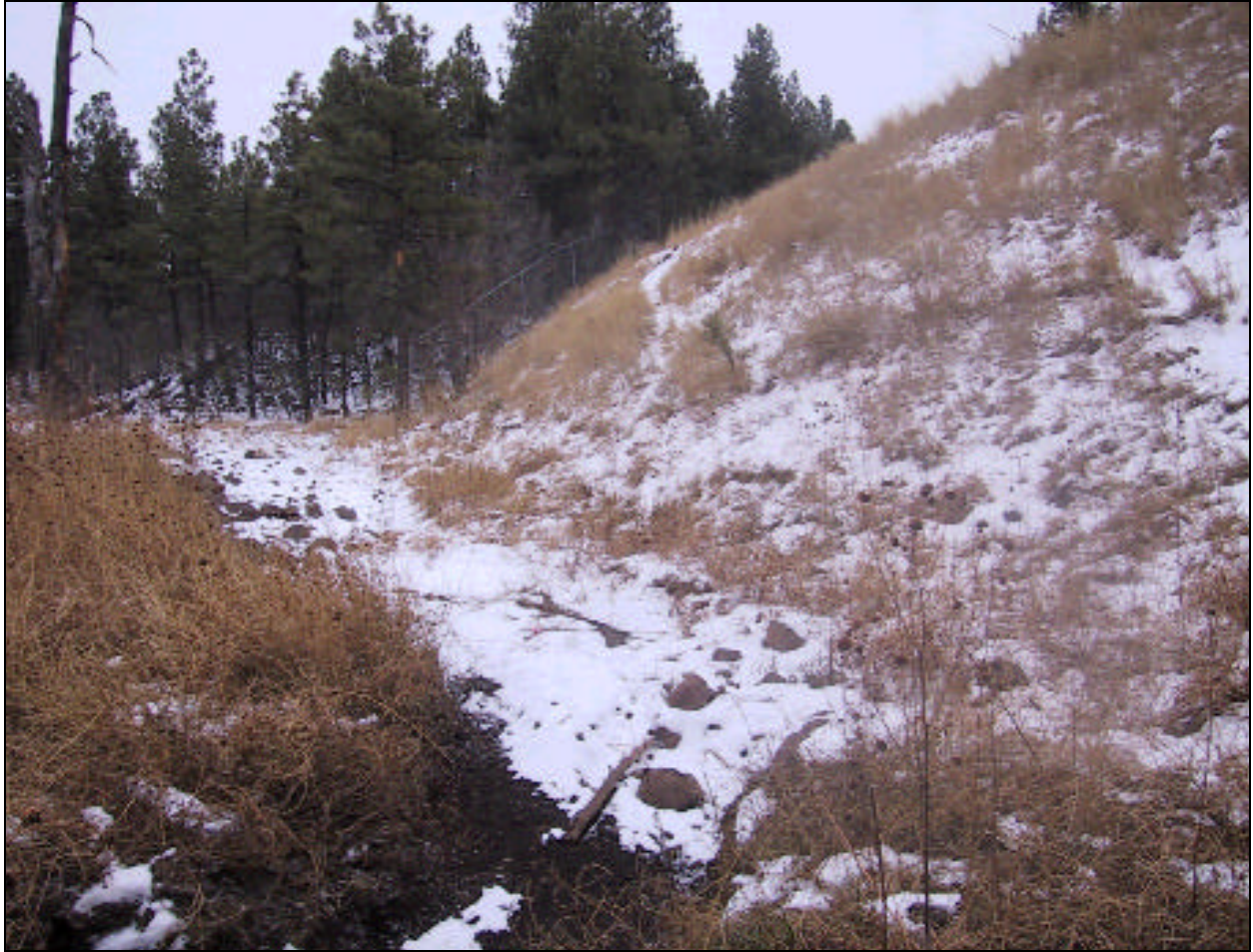
Figure A6. Steep road embankment at “C” adds excessive sediment to stream channel. Proposed action is to realign 150 ft of channel away from embankment. Area “C” on site map.
