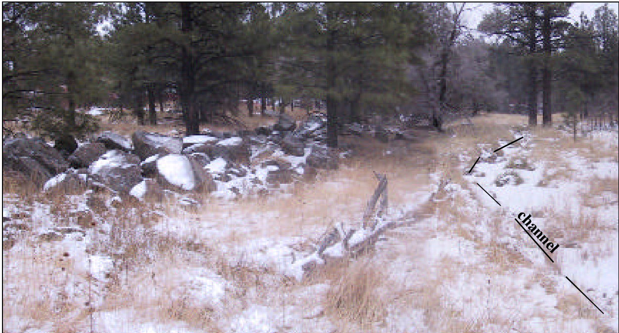
Figure A7. Large rock spoil piles along the floodplain at “D” on site map. Spoil material will be removed and/or smoothed to restore the floodplain.
