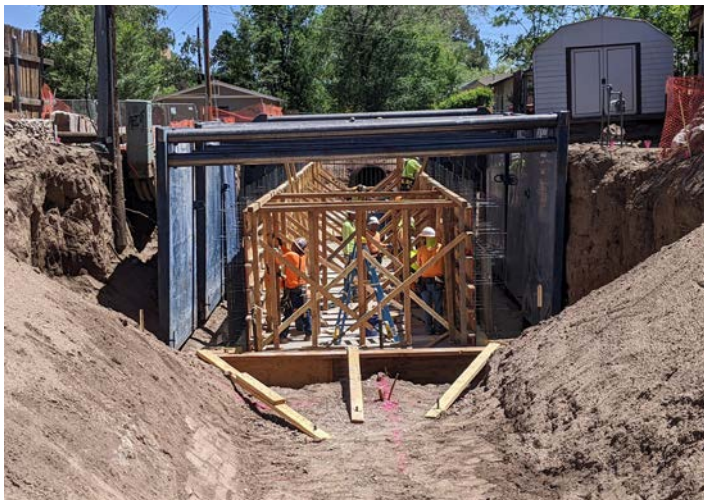
Drainage capital improvement.
