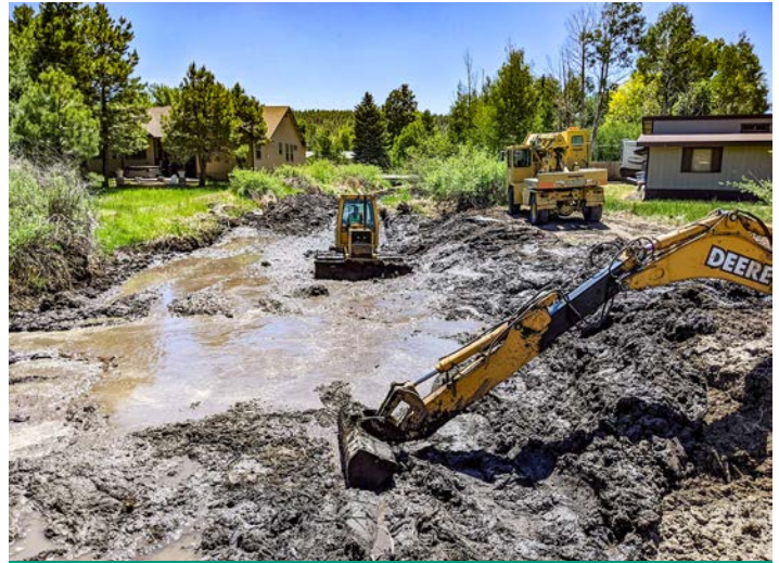
Open channel maintenance.
