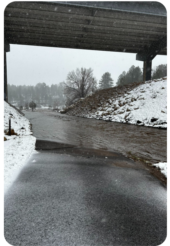
Rio de Flag plant IP crossing
