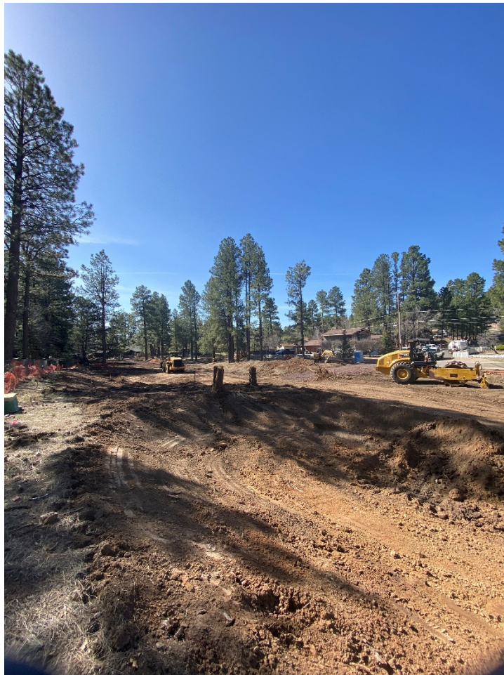
Earth work starting at Park Way Sediment Basins
