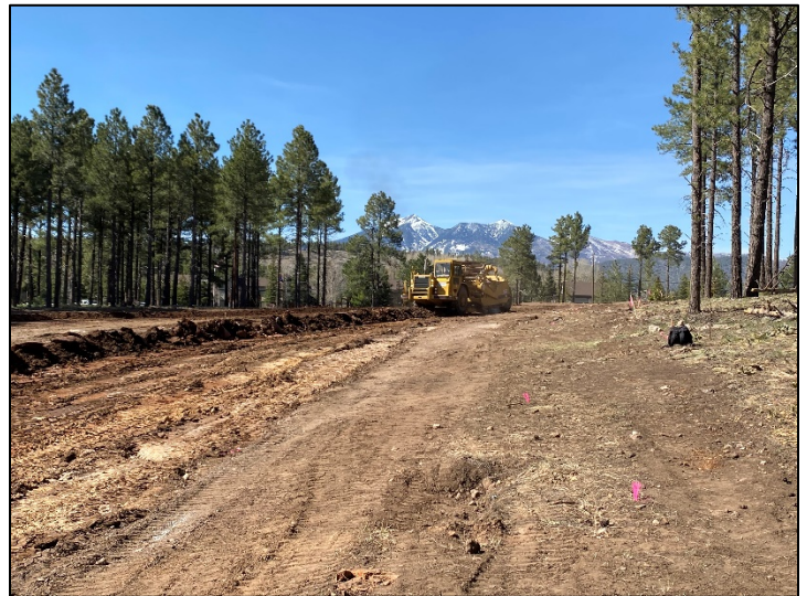
Grading Operations in Recently Cleared New Beulah Blvd
