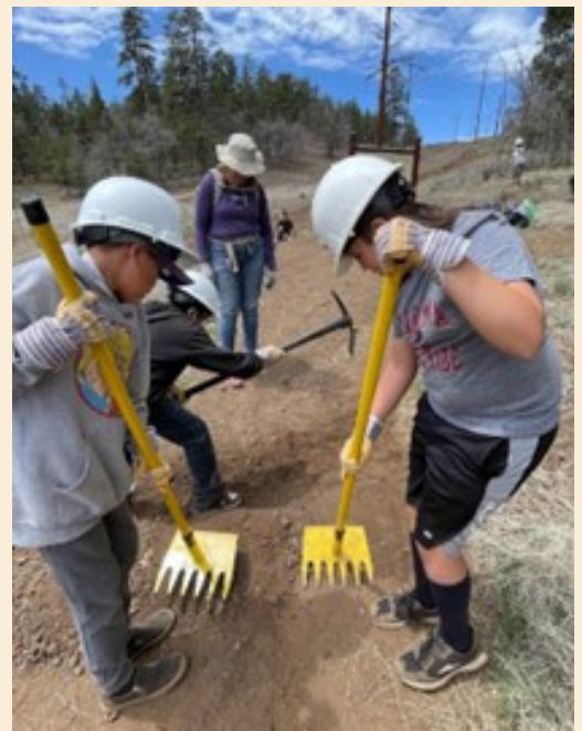
Right: Students use their tools to dig out a drainage canal and tamp down the berm.
