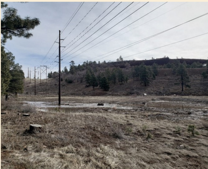
Flooding on the trail to deep water pond.
