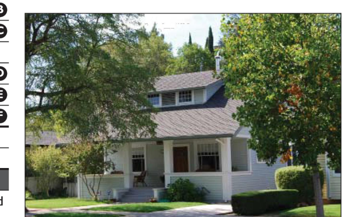
Full-length integral porch integrated into the overall massing.
