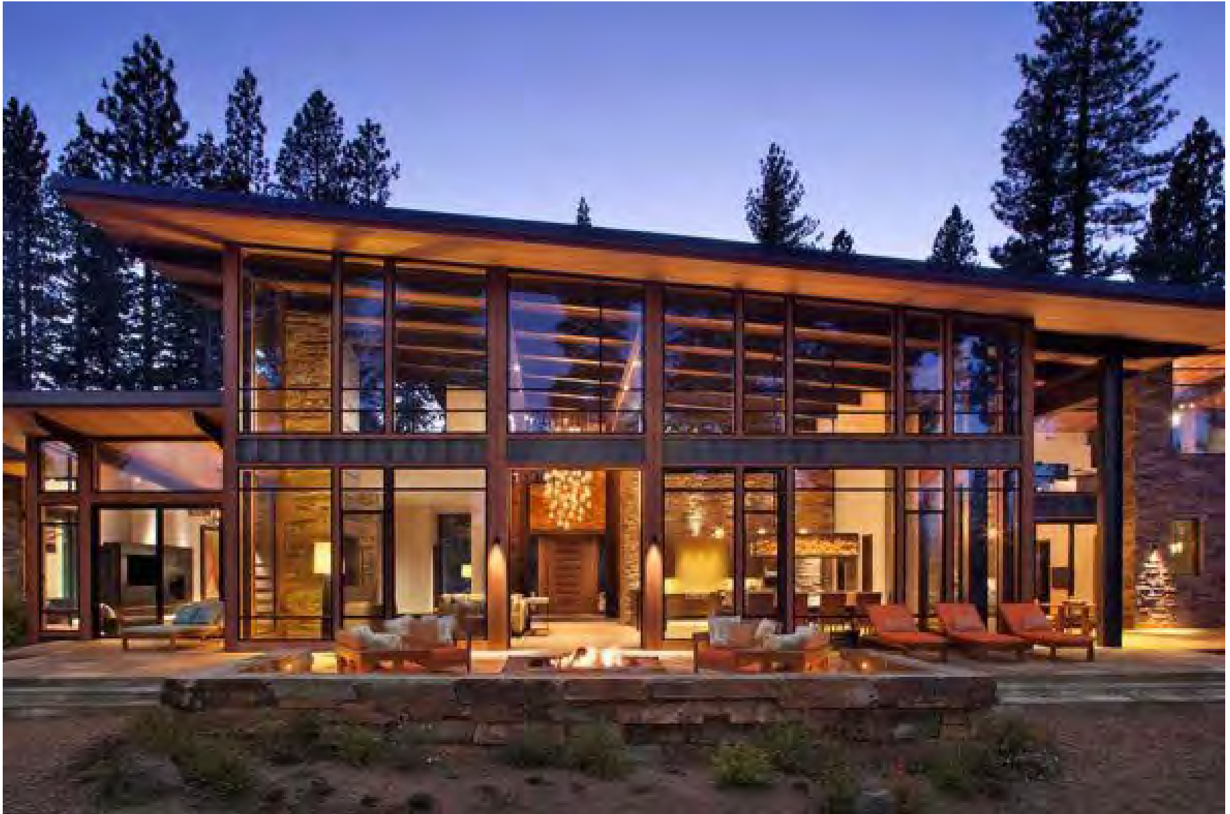
Image 60, Local vernacular with sloped roof form and exposed structure driven by views of the site.
