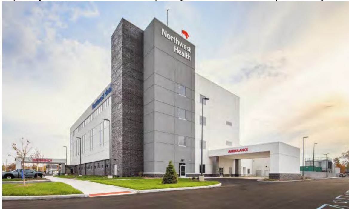
Image 57, EIFS as a primary material. EIFS forms define building elements and express articulation through different colors, scoring and texture.
