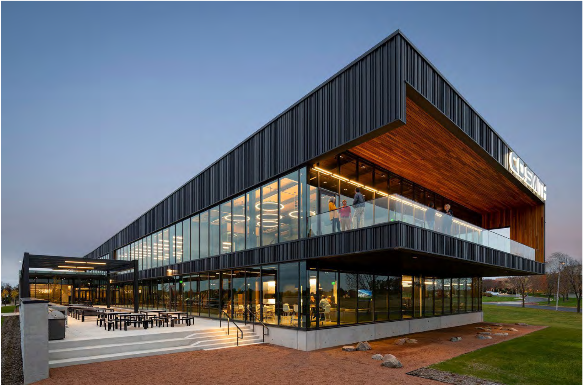
Image 54, Dark / contrasting metal panel with expressed ribs / texture, wood ceiling and wall material that extends from inside to outside. Deep overhangs and extended vertical planes.
