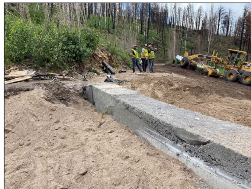
Concrete Encasement – Point I
