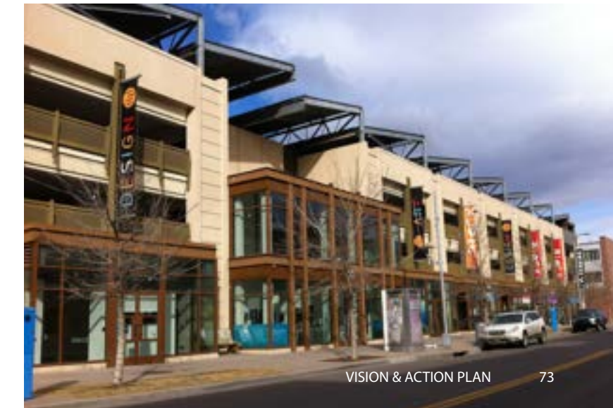
Parking structure with ground floor retail and roof top solar panels in Lakewood, CO
