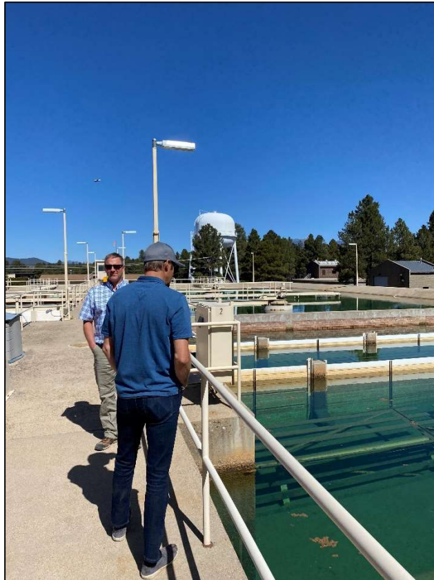
Staff and Brown & Caldwell taking a tour of the LMWTP basins
