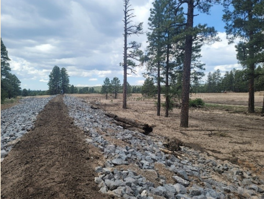
New trail between northern detention basins looking south.
