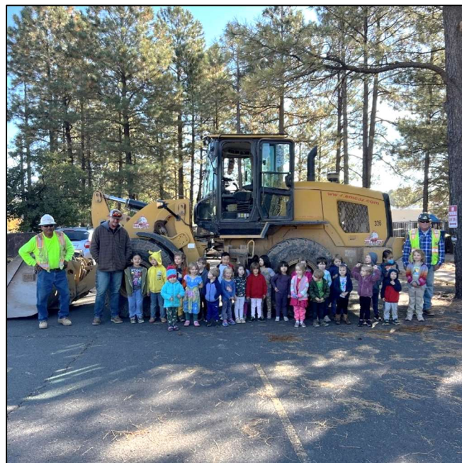
Eagle Mountain Construction takes time to have an equipment show and tell with the project adjacent Montessori School students
