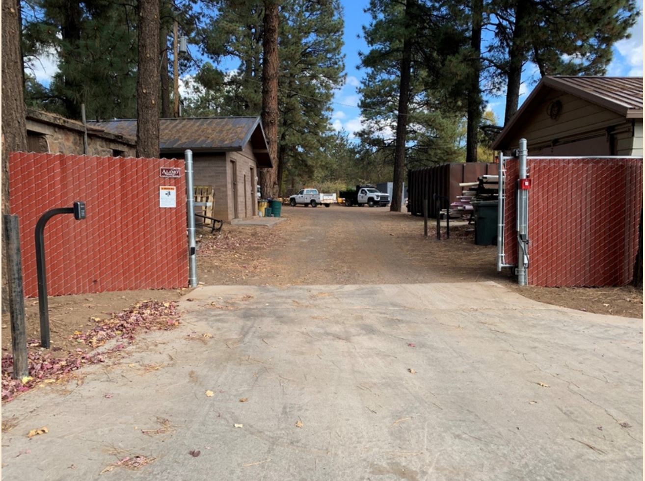
Above: The new automated gate.
