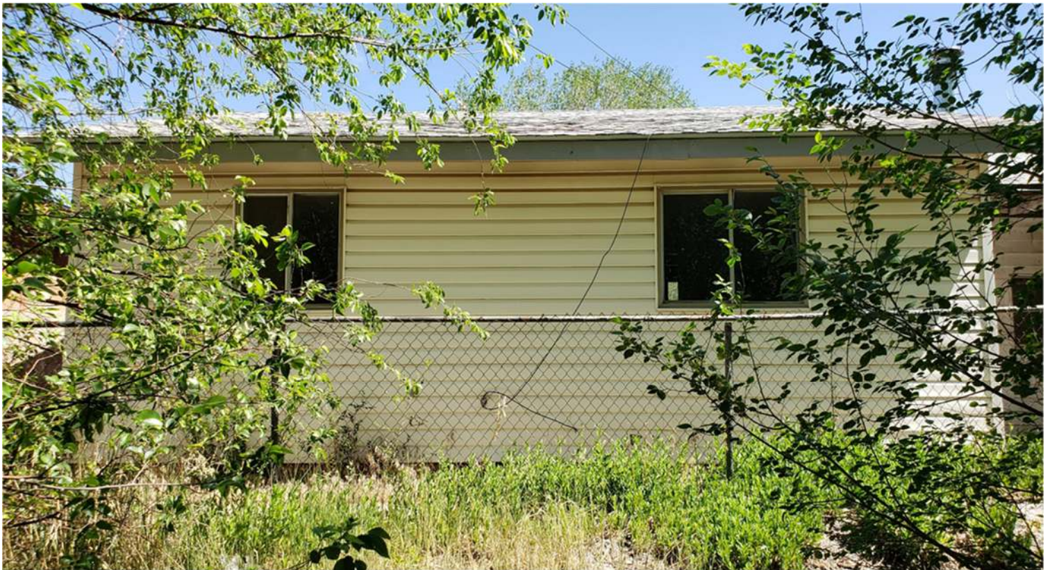
Photos 15–16. 609 S Lone Tree Rd S façade W half, alcove/enclosed porch entry of E half (top) and S façade W half (bottom); photos taken from neighboring property.
