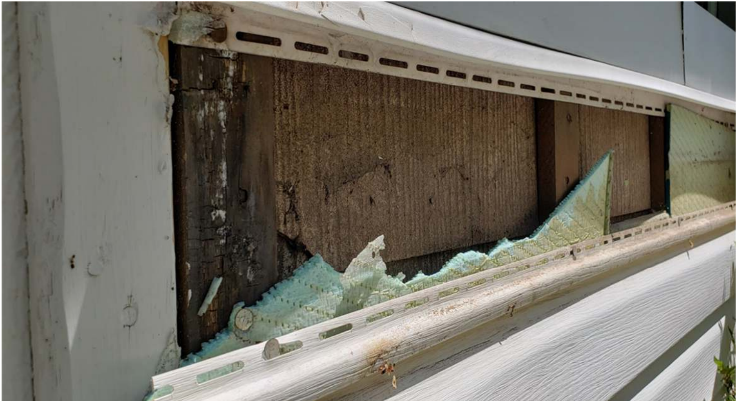
Photos 19–20. 609 S Lone Tree Rd W façade E half / N façade W half footer walls and wood-grained vinyl siding, view to SE (top); example of exterior finish layers on S façade E half, view to NE (bottom).
