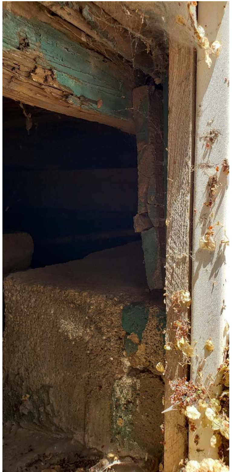
Photos 21–22. 609 S Lone Tree Rd E/front façade crawlspace opening showing footer wall, exterior finish layers, previous paint color; view to SSW (left) and NNW (right).
