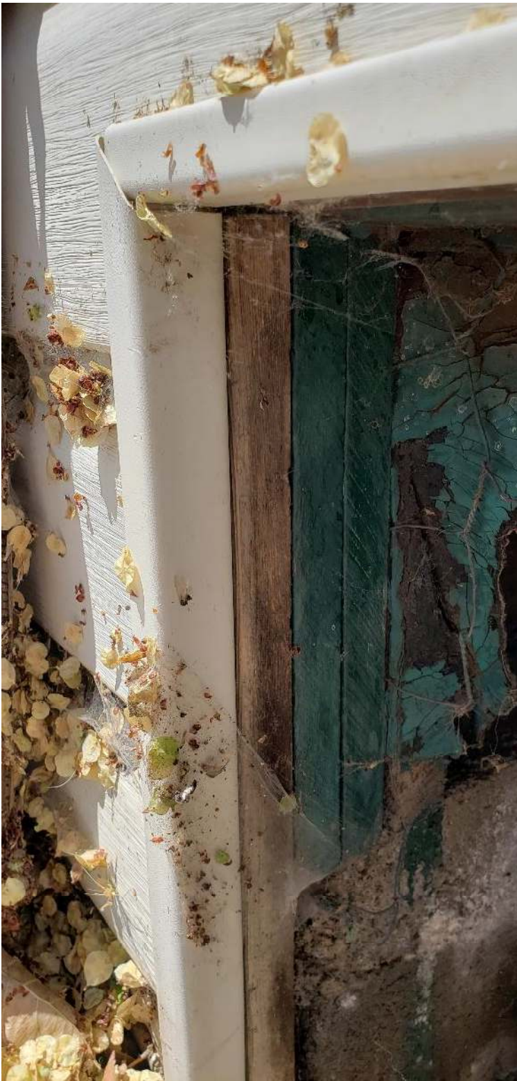
Photos 21–22. 609 S Lone Tree Rd E/front façade crawlspace opening showing footer wall, exterior finish layers, previous paint color; view to SSW (left) and NNW (right).
