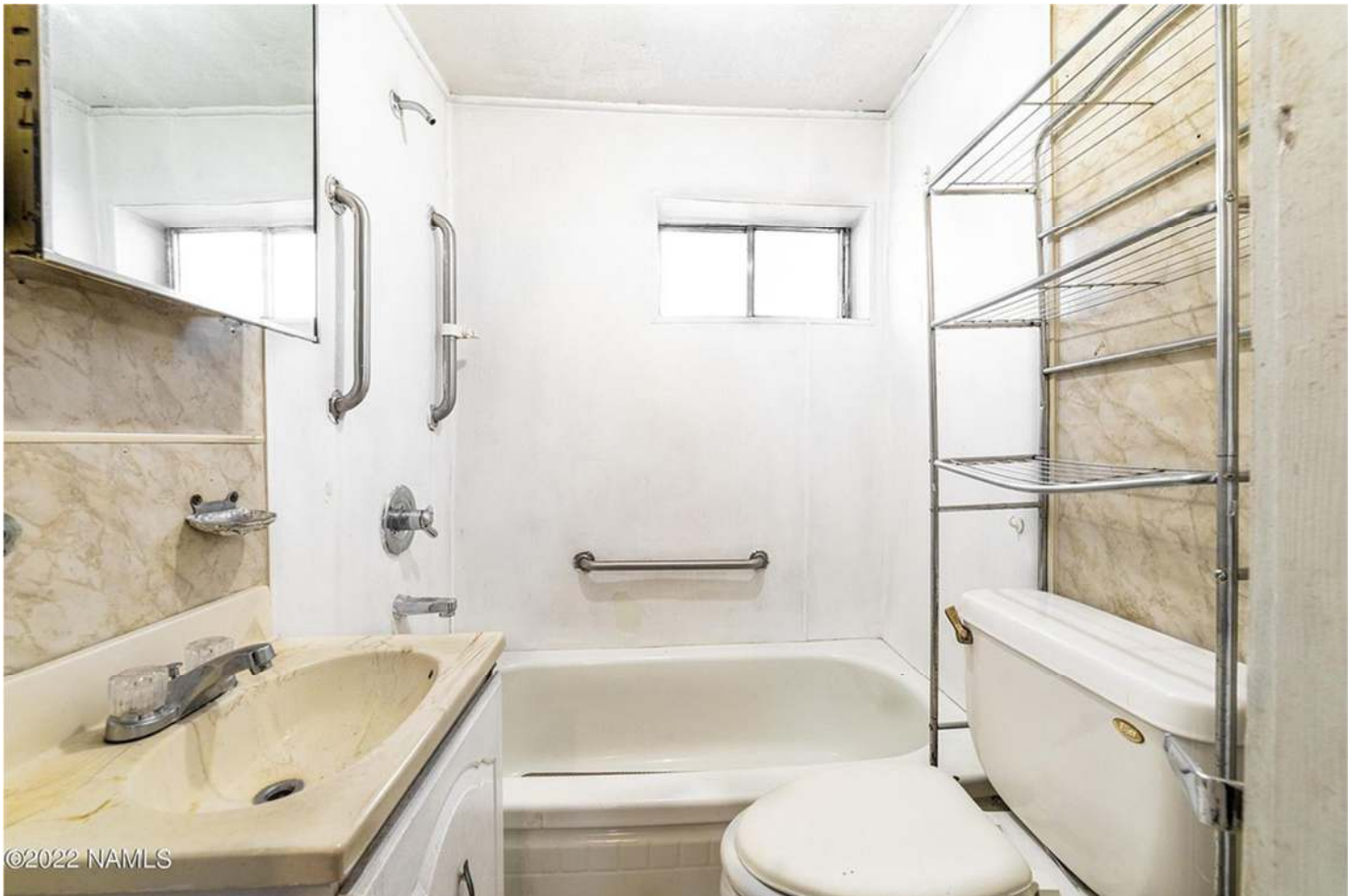
Photos 35–36. 609 S Lone Tree Rd kitchen S wall (top) and main house bathroom facing N (bottom).
