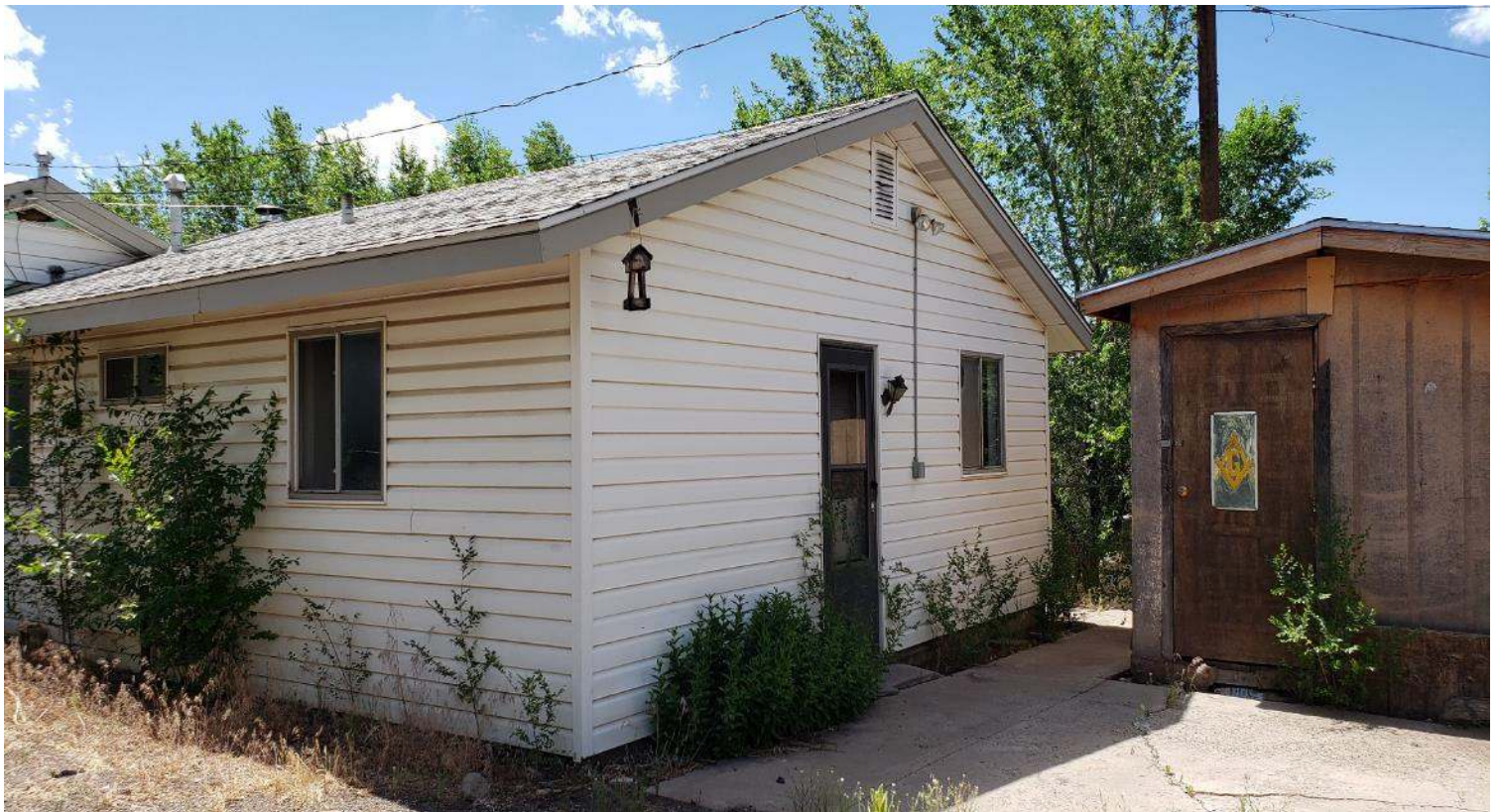
Photos 3–4. 609 S Lone Tree Rd front/E façade (top) and rear/W façade facing SE (bottom).
