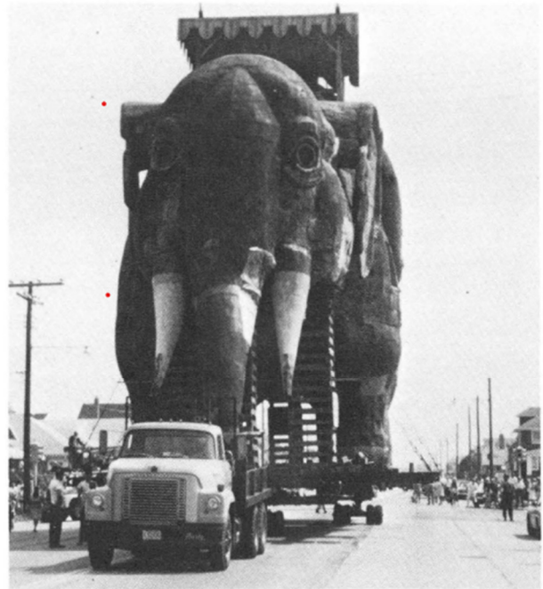
Following the move, "Lucy" was listed in the National Register of Historic Places, and thus was able to receive financial assistance from the Department of Housing and Urban Development and a grant from the National Park Service for restoration. The restored structure is now used as the Museum of New Jersey Shore History. [Photographs: Courtesy of John Milner Assoc.]
