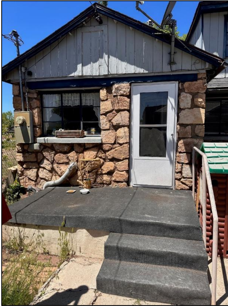
Plate 10. View west toward rear ell.
