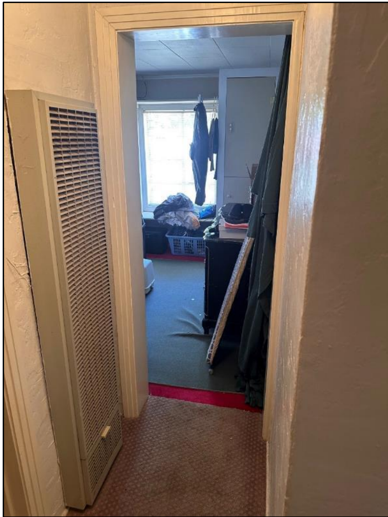
Plate 18. Hallway in front of bathroom toward rear bedroom/storage room.
