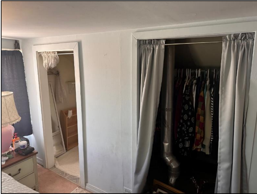
Plate 25. North bedroom, closets in east wall.
