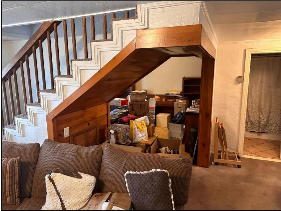
Plate 16. View from living room toward storage room in northwest corner and bathroom.
