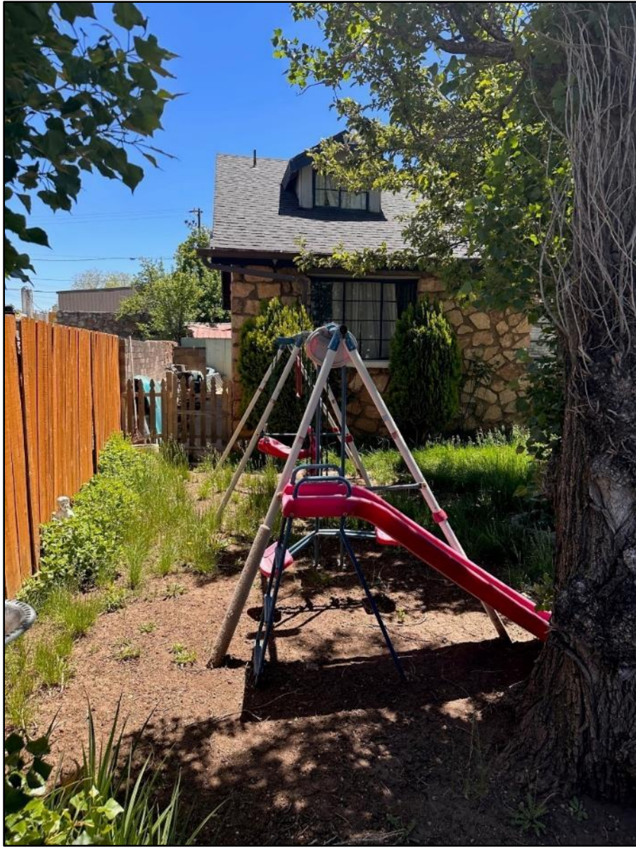
Plate 3. View east toward north half of west façade.
