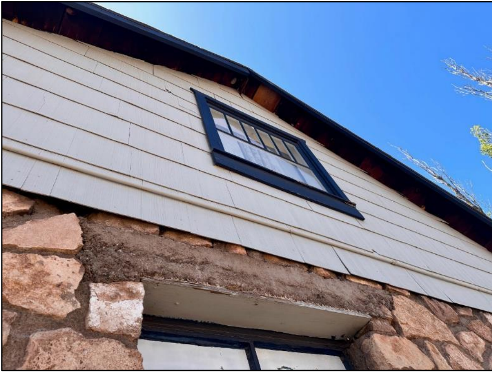
Plate 6. View of north gable details.
