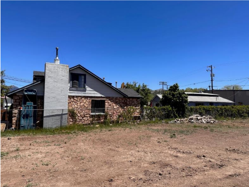
Plate 12. View of south elevation
